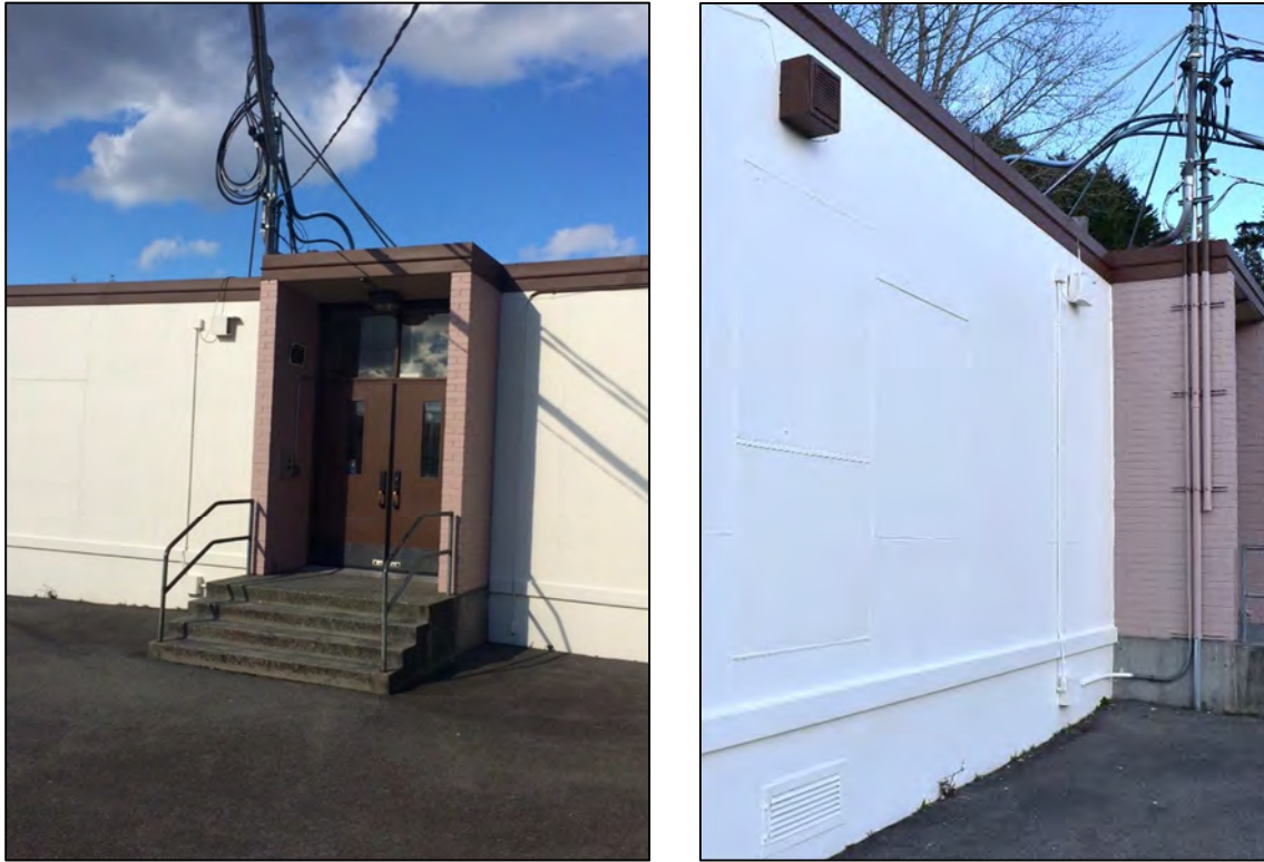
Fig. 33 – South facade of classroom wing, detail of entry and cement asbestos board panels
