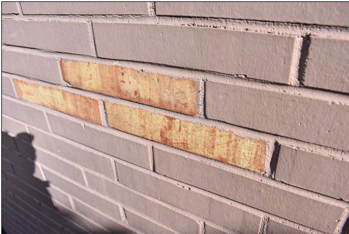
Fig. 30 – West facade of classroom wing, detail showing original brick coloration.
