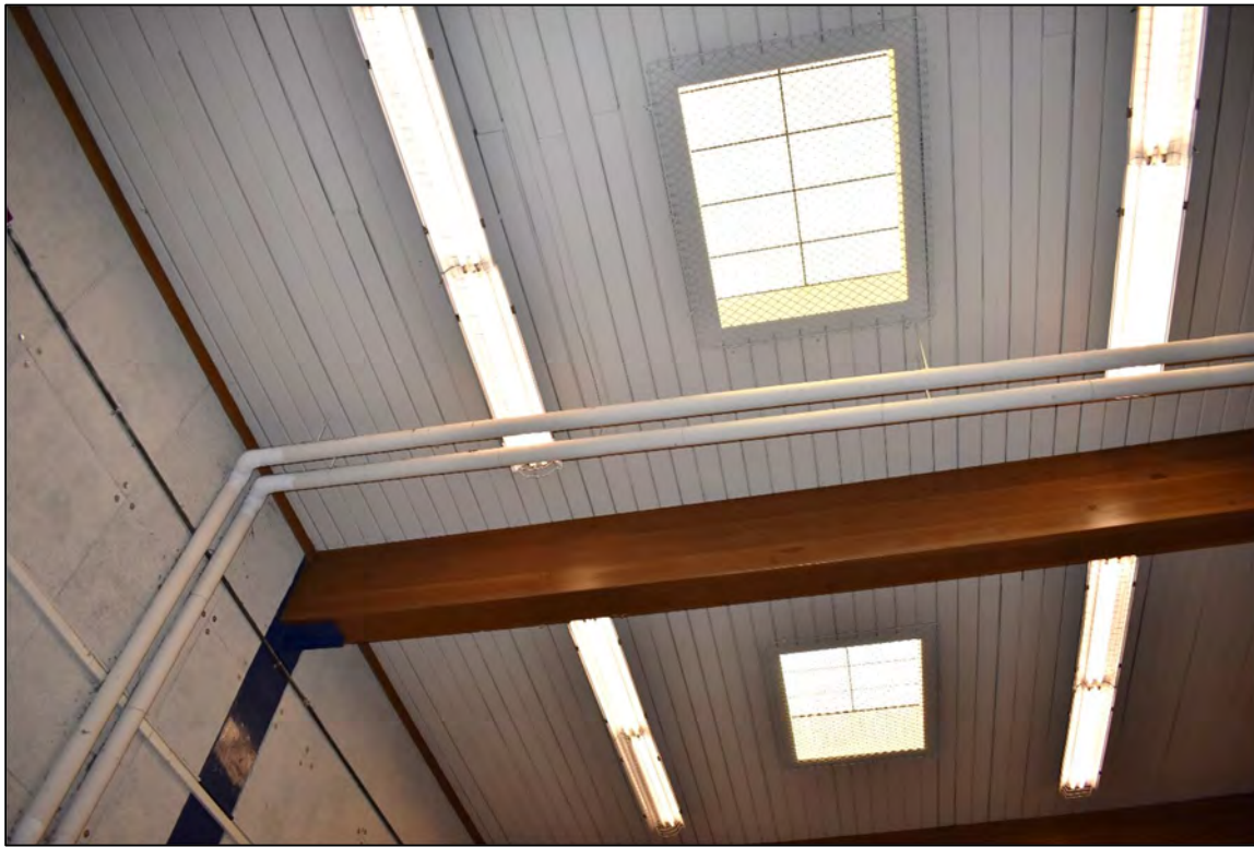
Fig. 57 – Interior, gymnasium, detail of skylights and glulams
