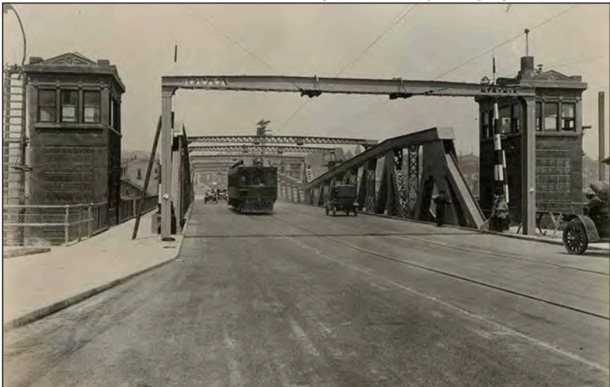
Figure 30 • Opening day of the Fremont Bridge, 1917 (The Fremont Bridge is a City of Seattle Landmark)
