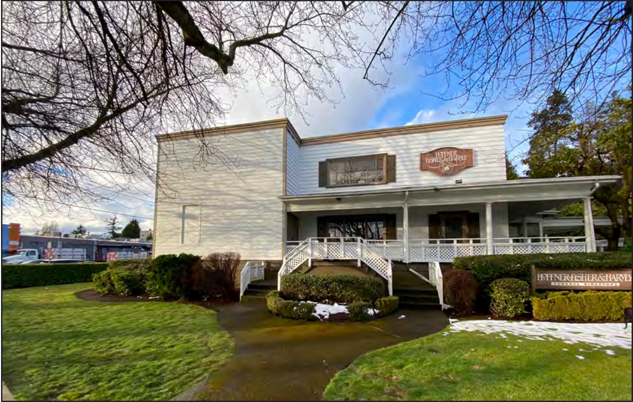
Figure 12 • Subject building, southern façade
