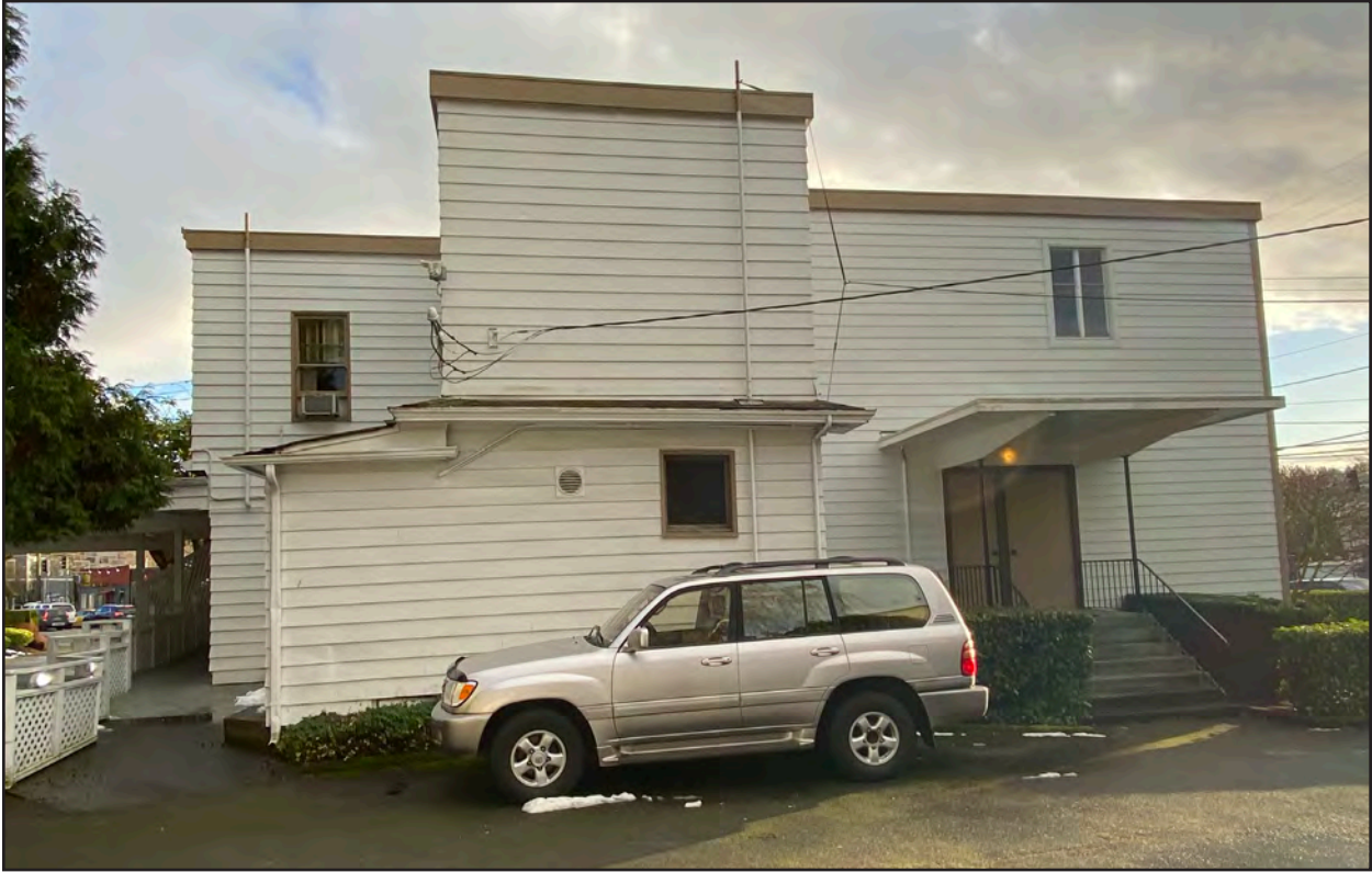
Figure 14 • Subject building, northern façade
