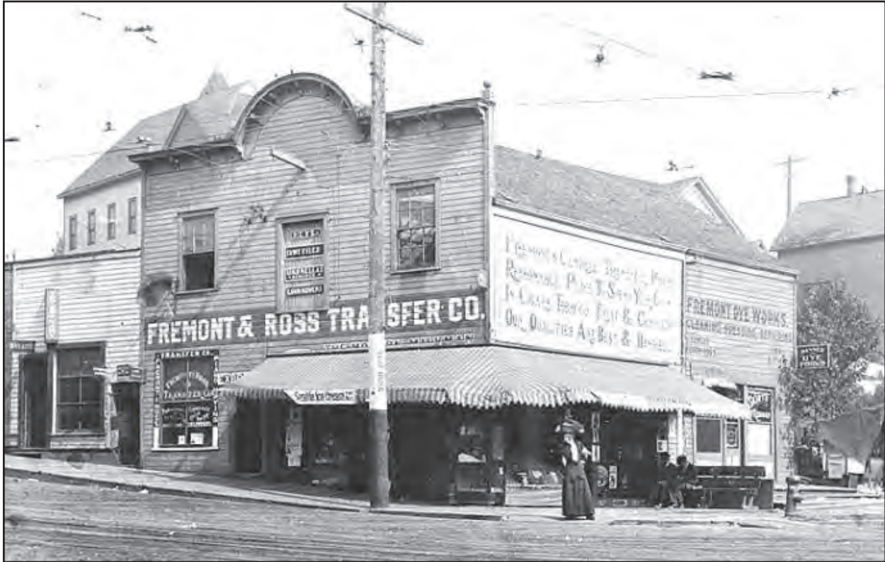
Figure 29 • Fremont & Ross Transfer Co., northeastern corner of Fremont Avenue and N 35th Street, 1910 (demolished)
