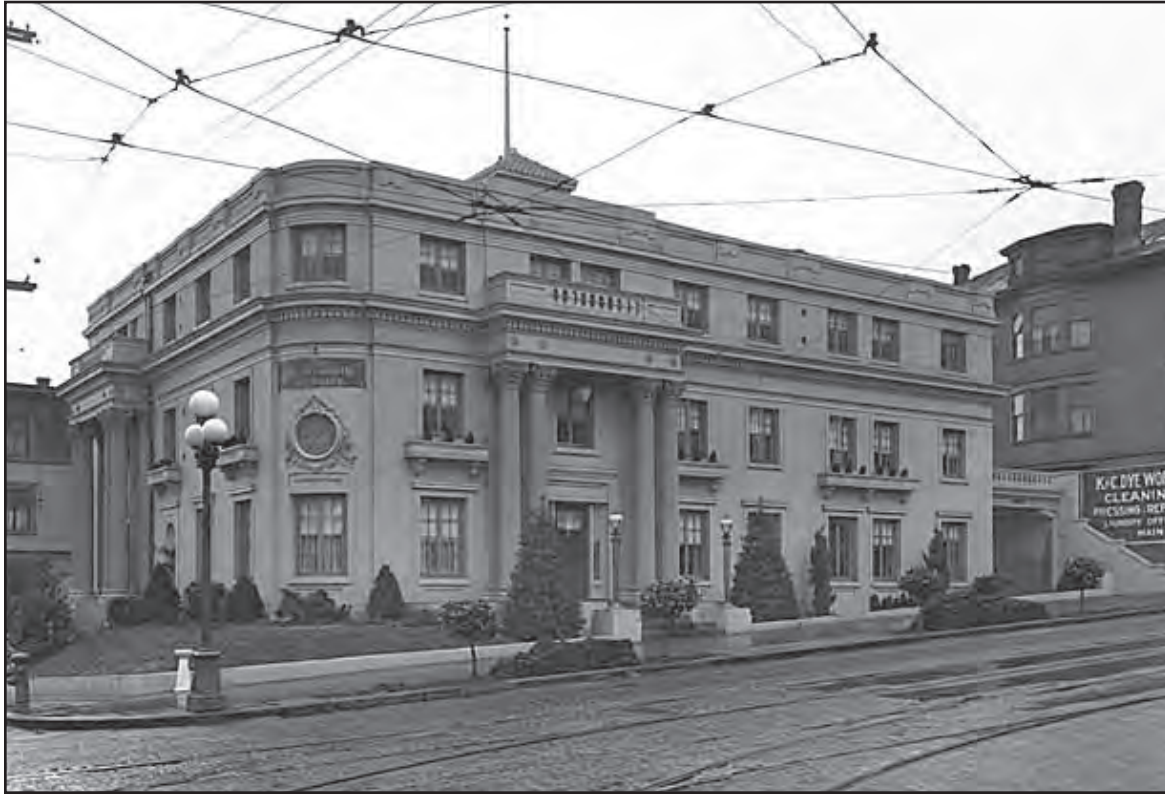
Figure 46 • E. R. Butterworth & Sons Mortuary, 3900 E Pine Street, ca. 1923 (extant)
