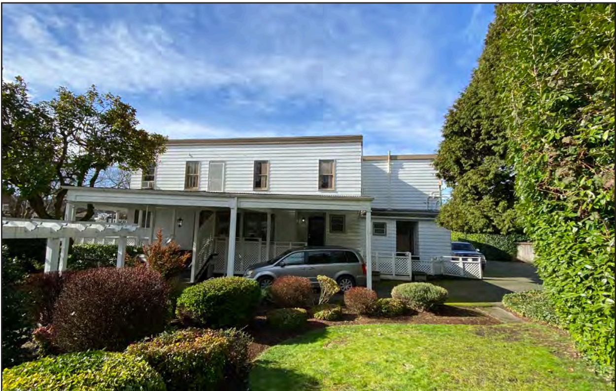
Figure 15 • Subject building, eastern façade
