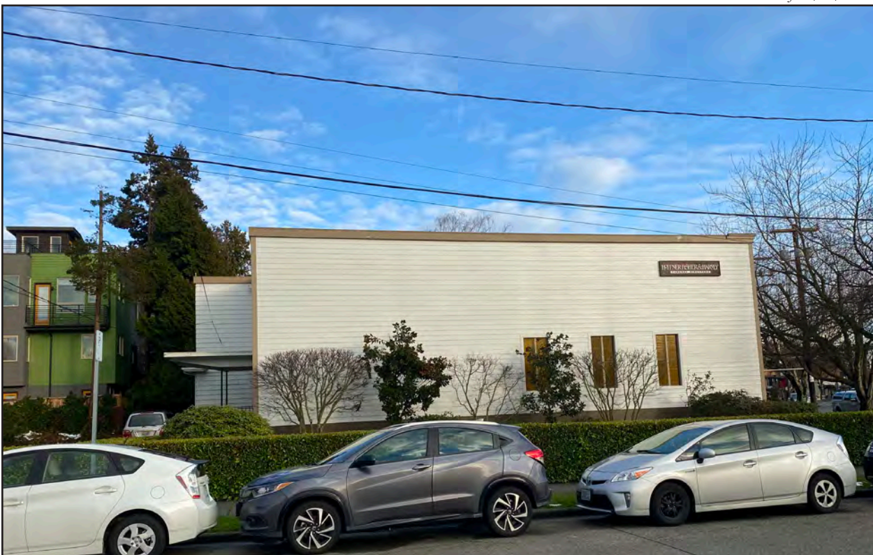
Figure 13 • Subject building, western façade
