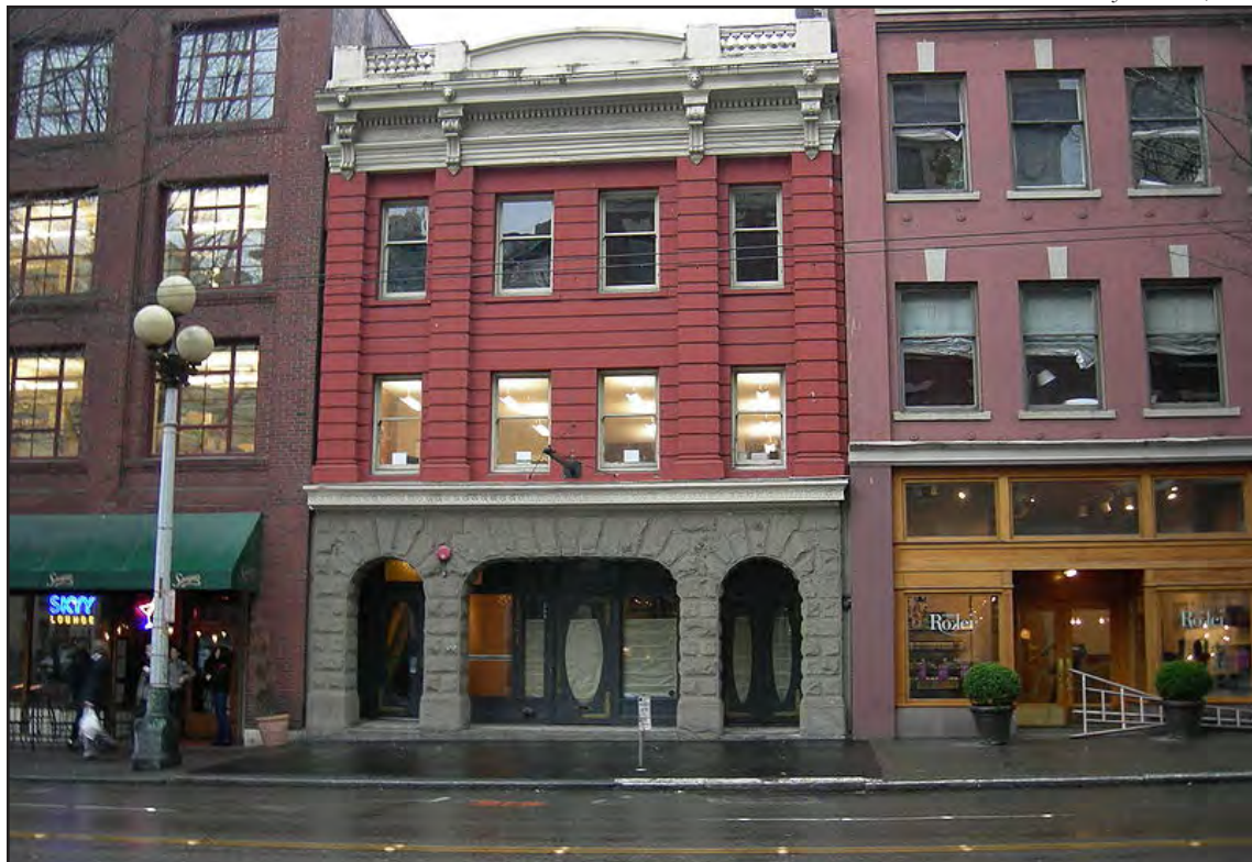
Figure 45 • Butterworth Building, 1921 First Avenue, 2008 (extant)
