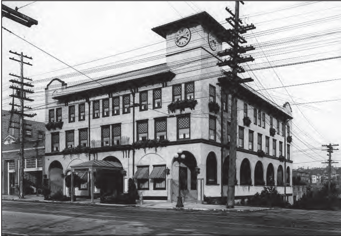
Figure 50 • Bonney-Watson Building, funeral parlor, 1702 Broadway, 1912 (Now demolished. Not to be confused with the Booth Building, located one block south, which has a similar building form and style.)
