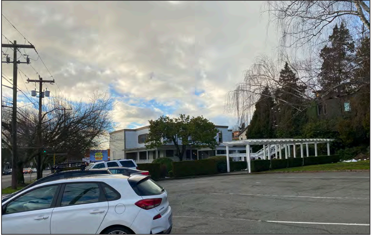
Figure 8 • Viewing northwest to subject building from parking lot
