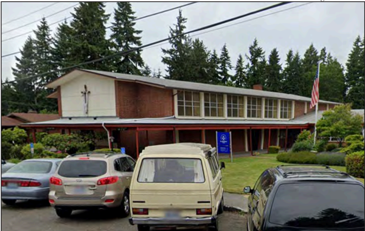
Figure 73 • St. Matthew Parish Church, 15th Avenue NE and E 127th Street (1954, James Klontz, extant)
