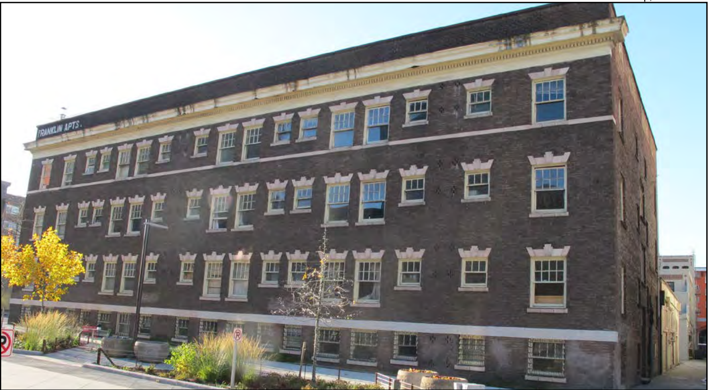
Figure 12 • Franklin Apartment Building, southern façade
