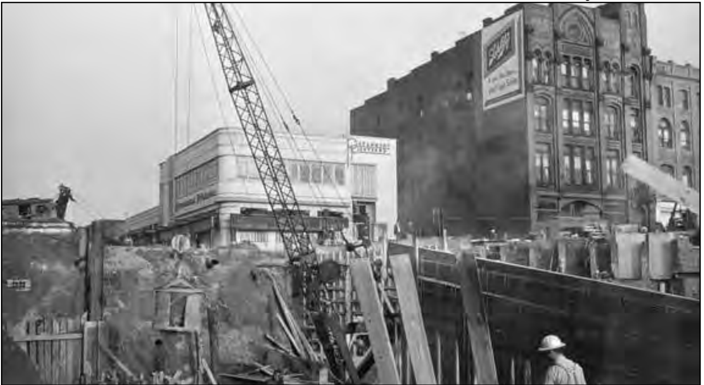
Figure 27 • Construction of the Battery Street Tunnel, 1952
