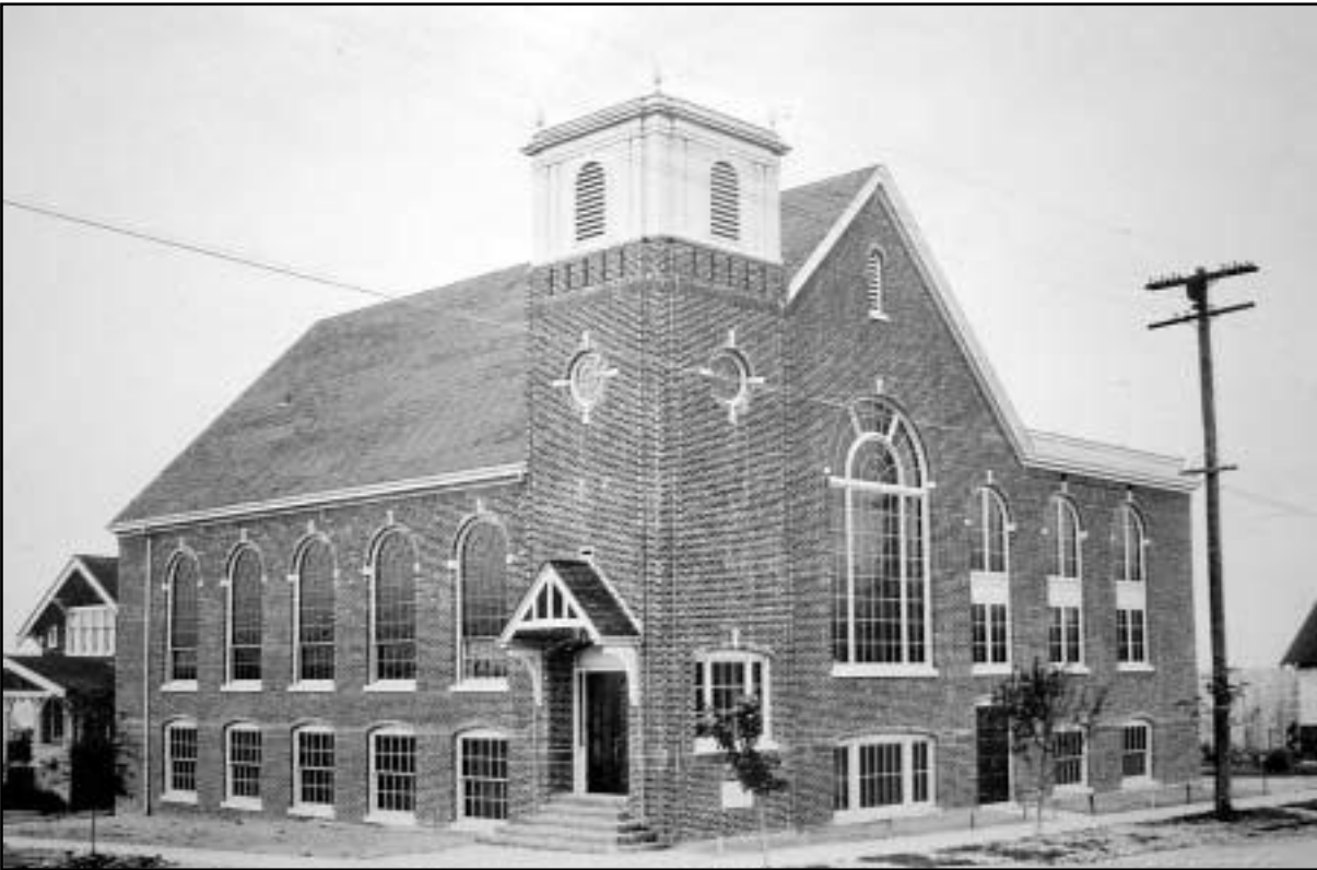
Figure 61 • Ravenna United Methodist Church (1922, Lawton and Moldenhour)
