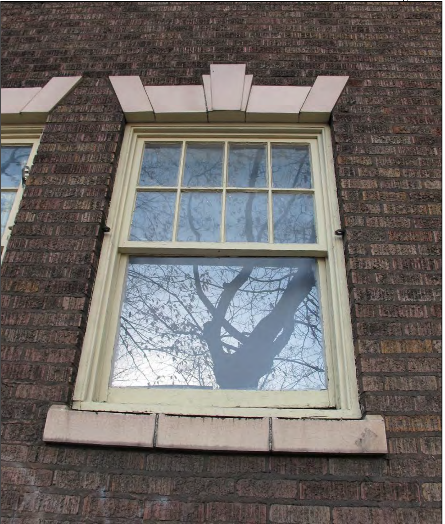
Figure 15 • Franklin Apartment Building, typical window
