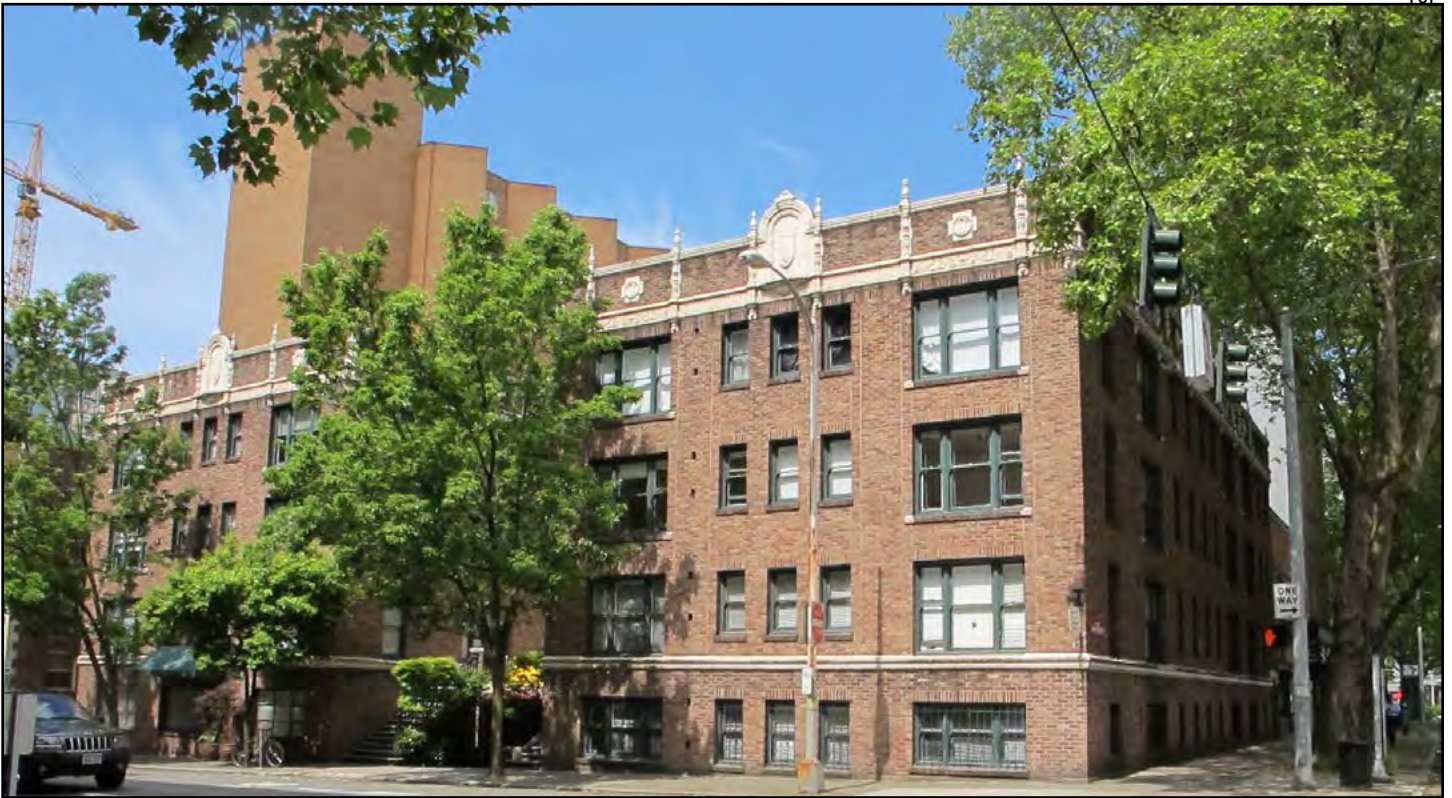
Figure 40 • The Davenport Apartments, 420 Vine Street (1925)
