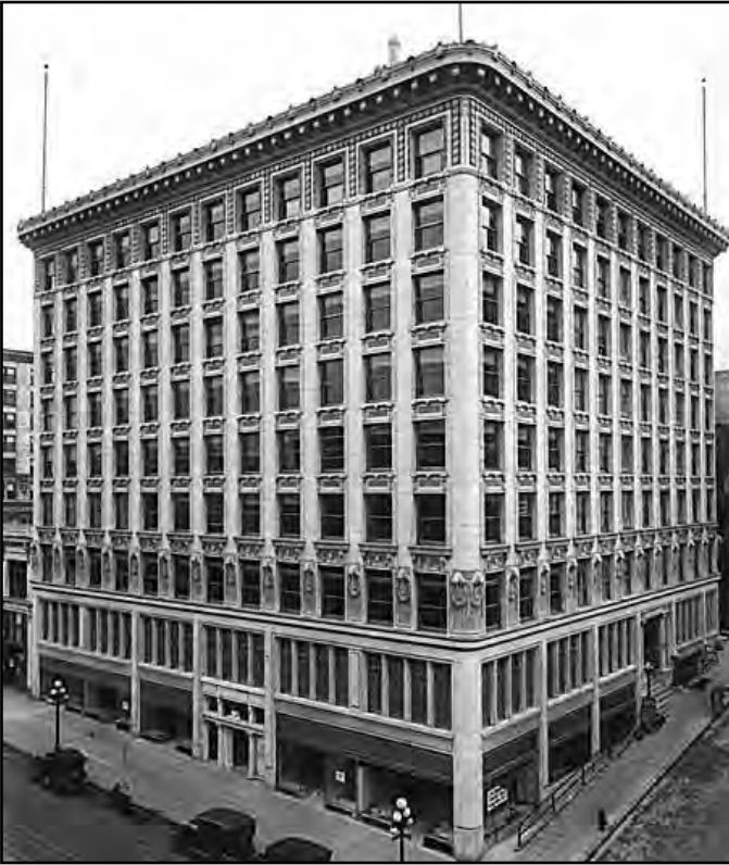
Figure 60 • Arctic Building, 700 Third Avenue (1913-17, A. W. Gould and Lawton)
