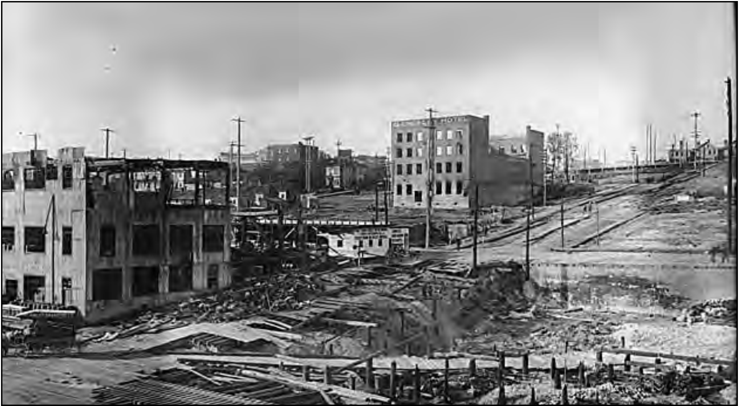
Figure 26 • Damage from Belltown Fire, 1910
