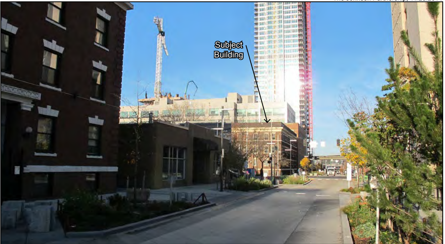
Figure 5 • View B--Viewing northeast on Bell Street
