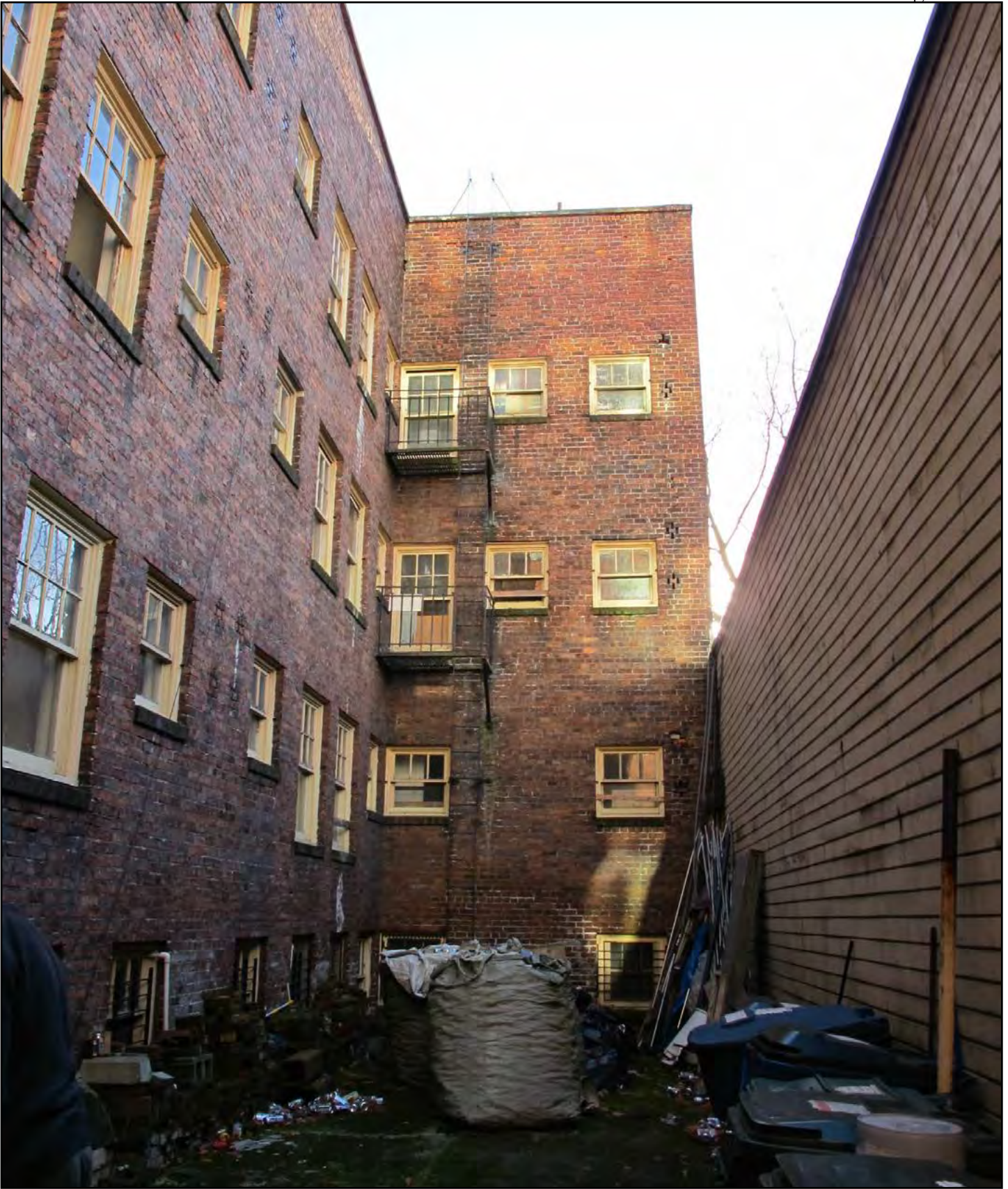
Figure 16 • Franklin Apartment Building, northern lightwell viewing west
