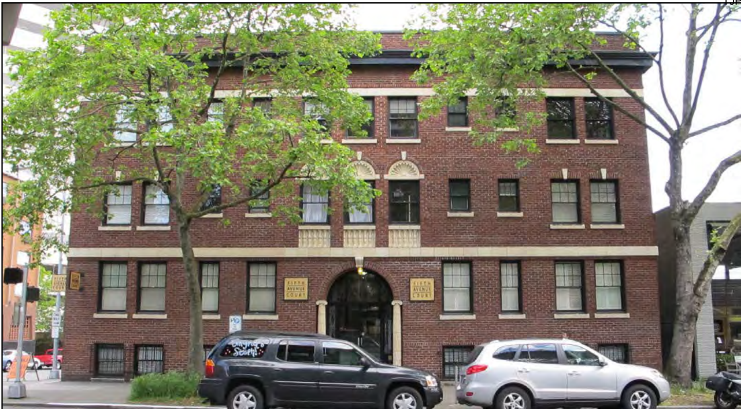
Figure 37 • Fifth Avenue Court, 2132 5th Avenue (1922, George W. Lawton and Herman Moldenhour)
