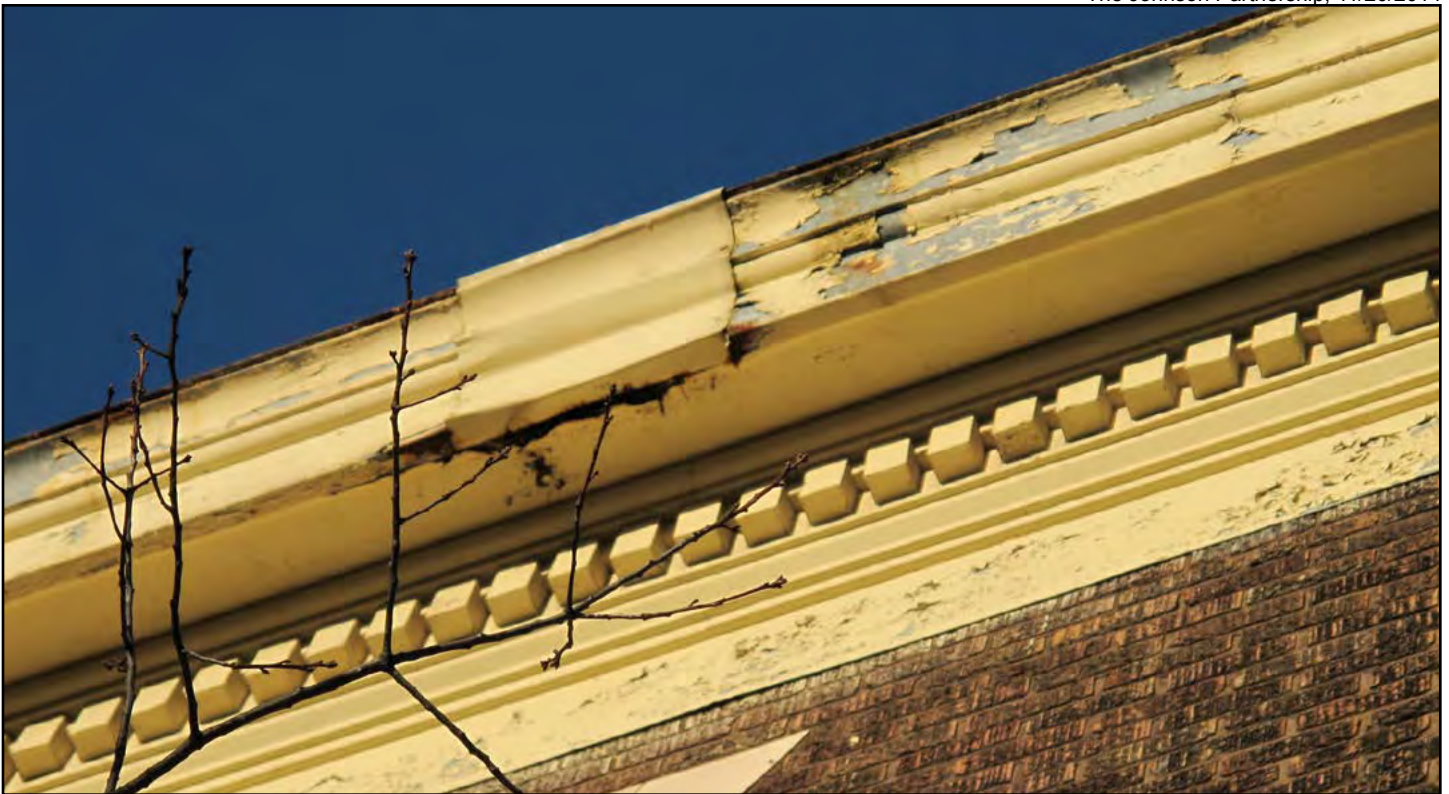
Figure 10 • Franklin Apartment Building, detail of metal cornice
