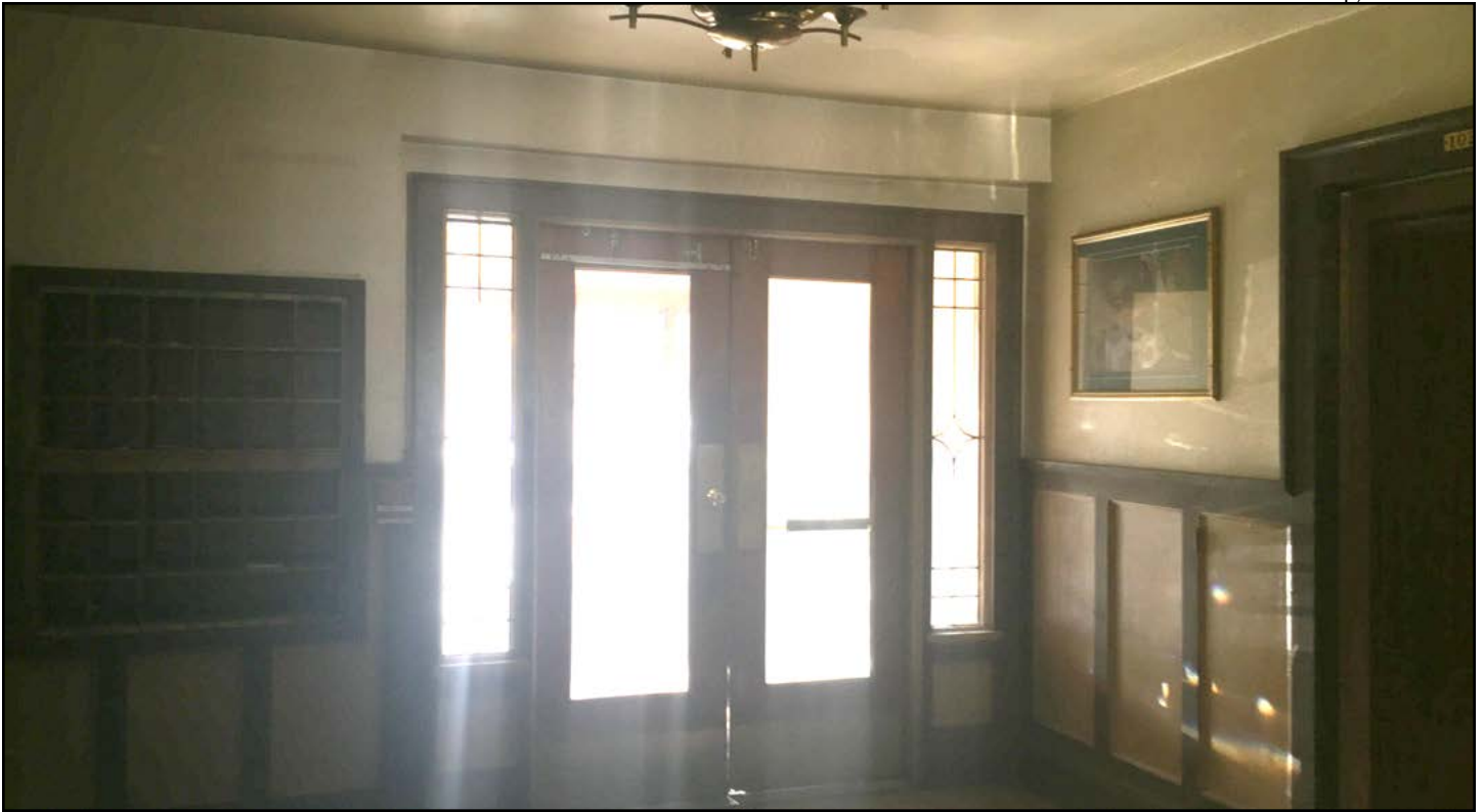
Figure 18 • Franklin Apartment Building, entry vestibule viewing southwest
