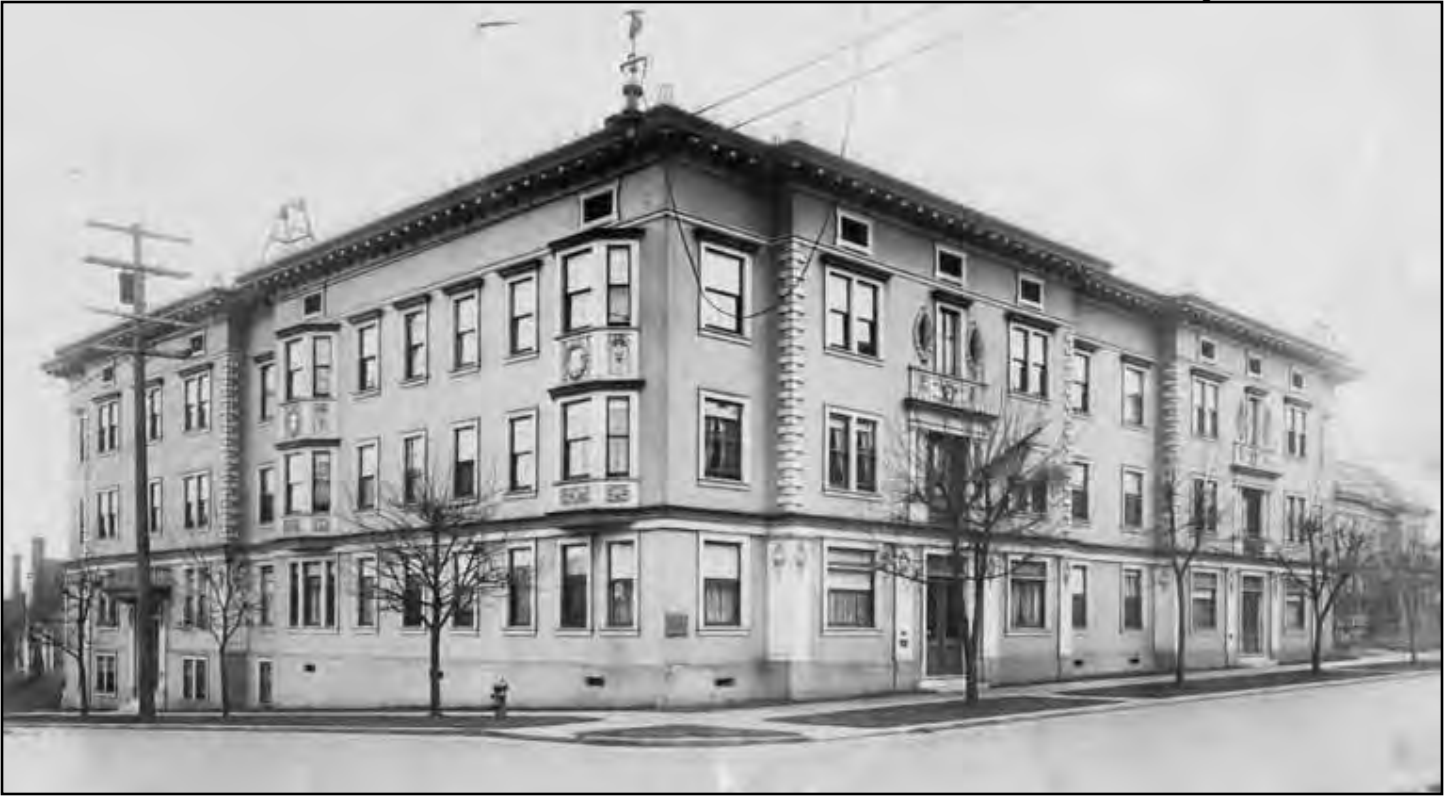
Figure 28 • St. Paul Apartment Building, First Hill, 1901
