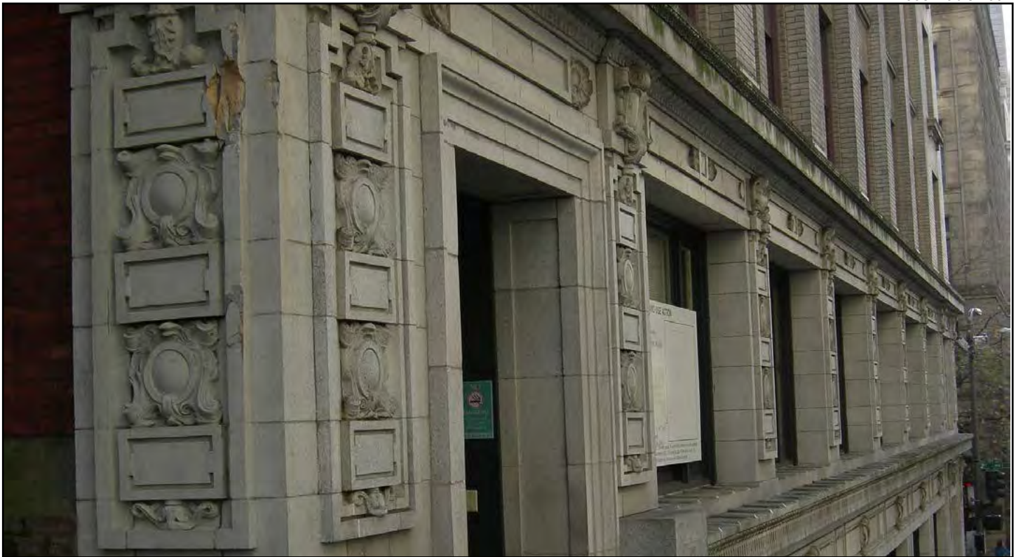
Figure 49 • Terra cotta detail on the Alaska Building
