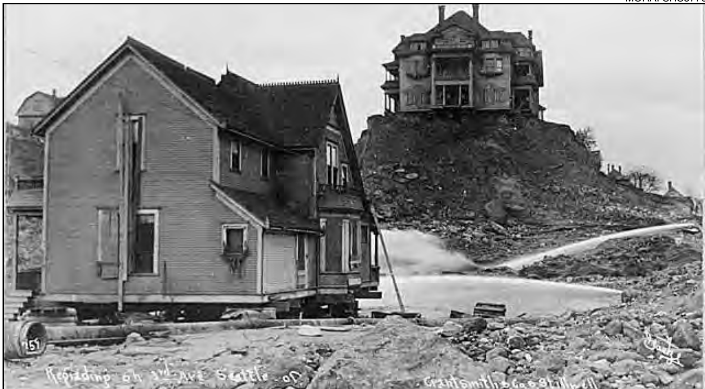
Figure 24 • Belltown, Third Avenue, 1908
