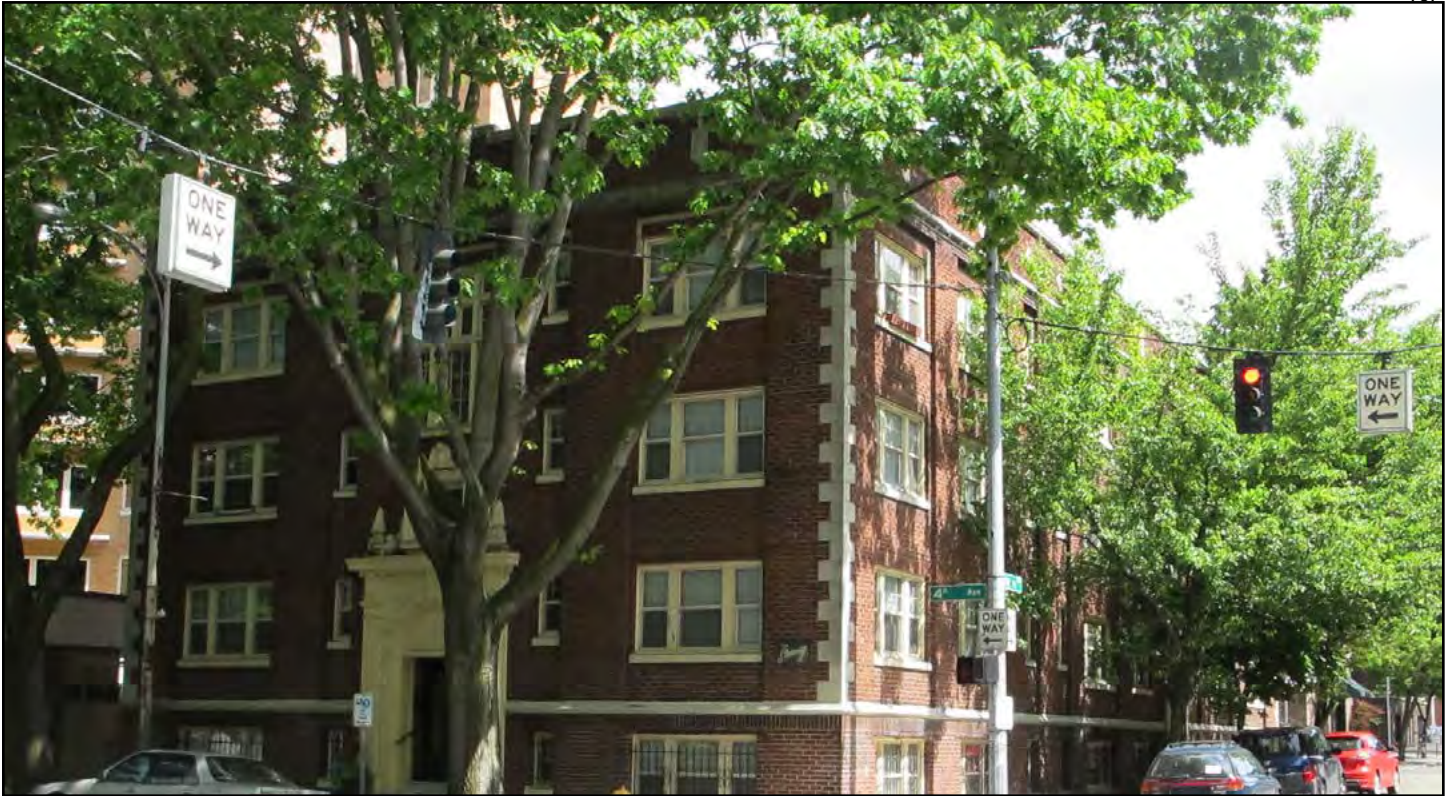
Figure 38 • The Stone Cliff Apartments, 2602 4th Avenue (1923)
