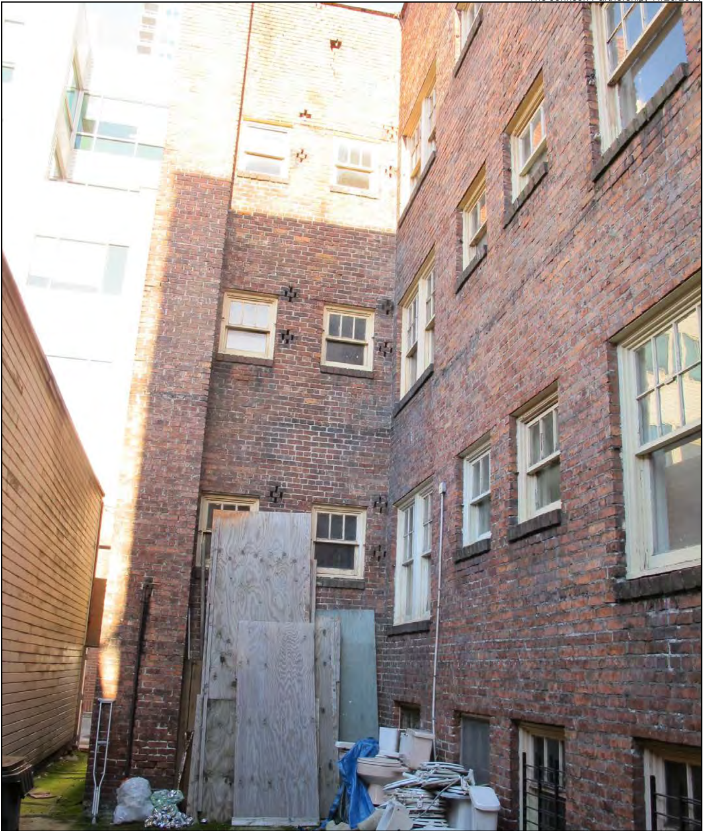
Figure 17 • Franklin Apartment Building, northern lightwell viewing east
