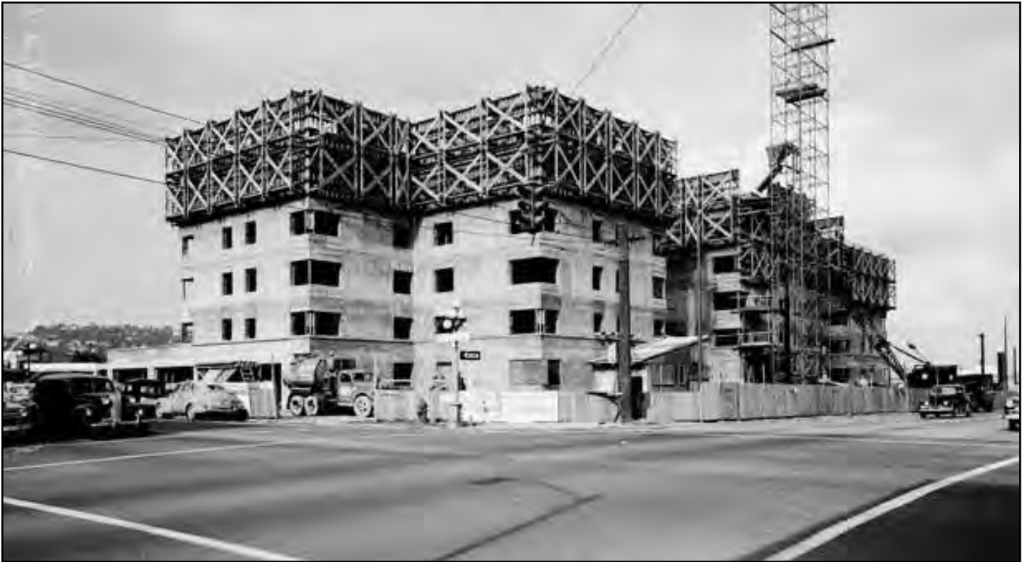
Figure 44 • The Grosvenor House Apartments under construction at 800 Wall Street, 1949
