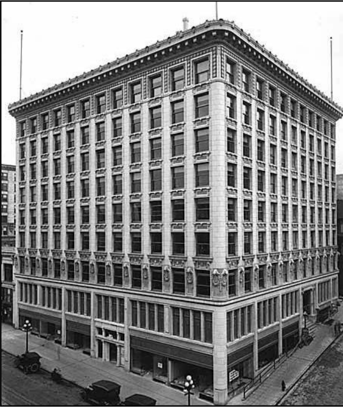
Figure 48 • Arctic Building, 700 Third Avenue (1913-17, A. W. Gould and Lawton)
