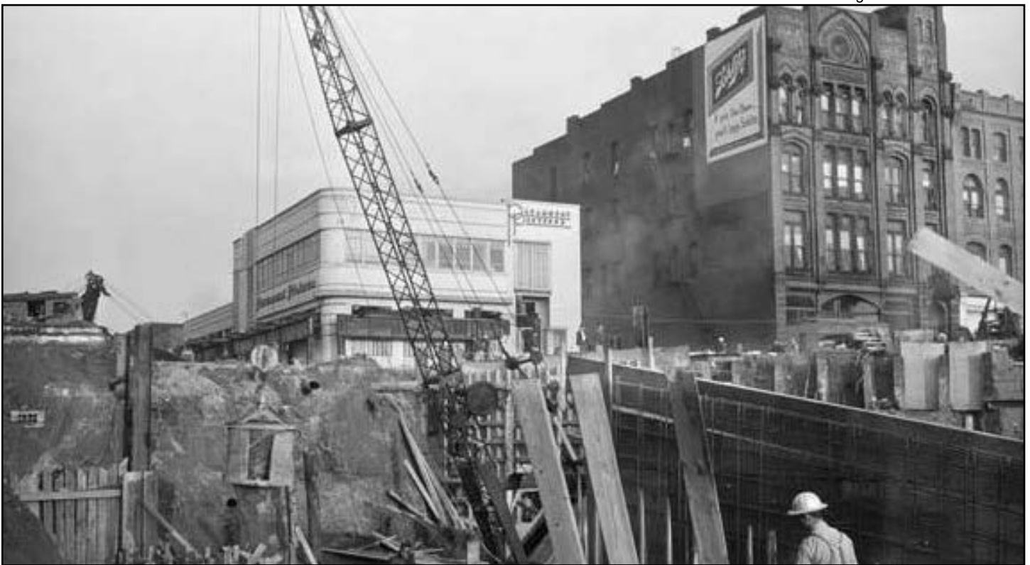
Figure 27 • Construction of the Battery Street Tunnel, 1952
