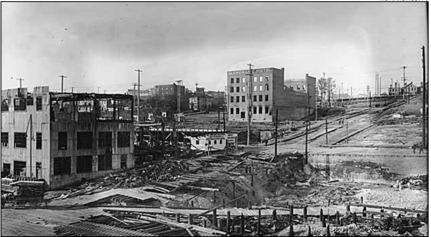
Figure 26 • Damage from Belltown Fire, 1910
