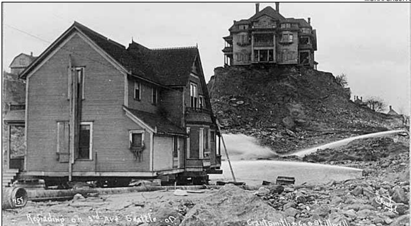
Figure 24 • Belltown, Third Avenue, 1908
