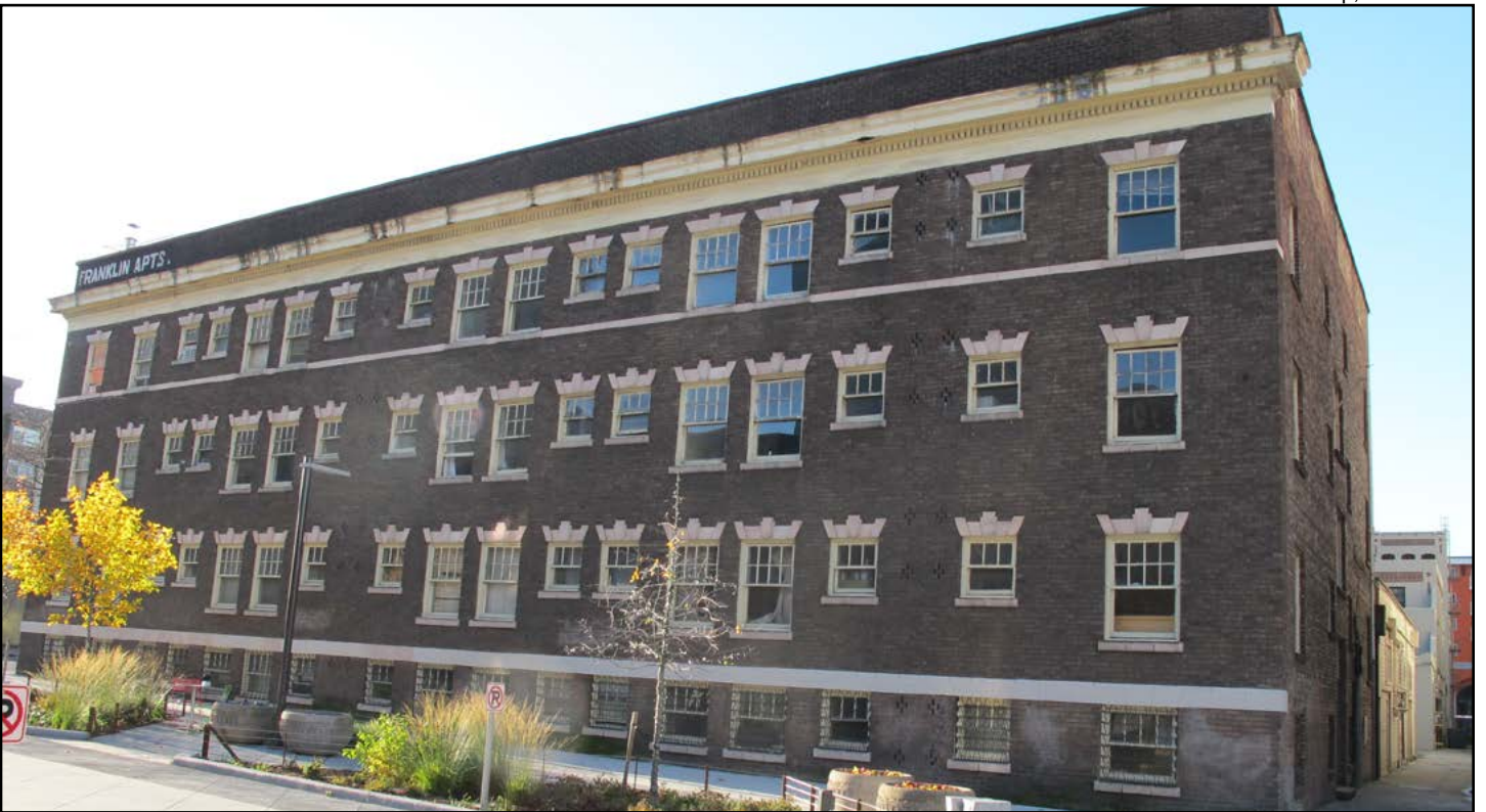
Figure 12 • Franklin Apartment Building, southern façade
