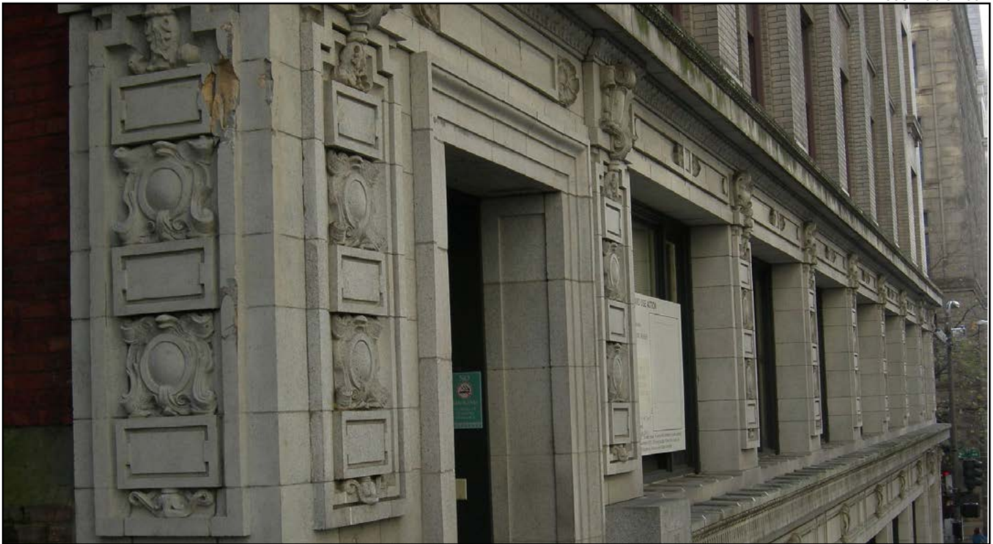
Figure 35 • Terra cotta detail on the Alaska Building
