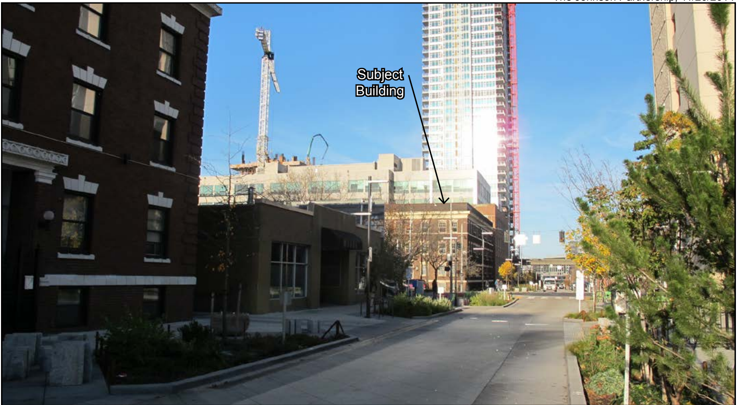
Figure 5 • View B--Viewing northeast on Bell Street
