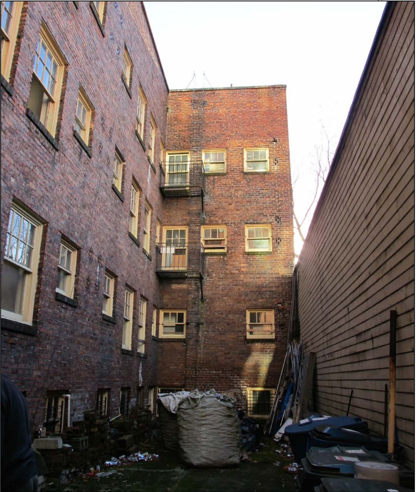
Figure 16 • Franklin Apartment Building, northern lightwell viewing west
