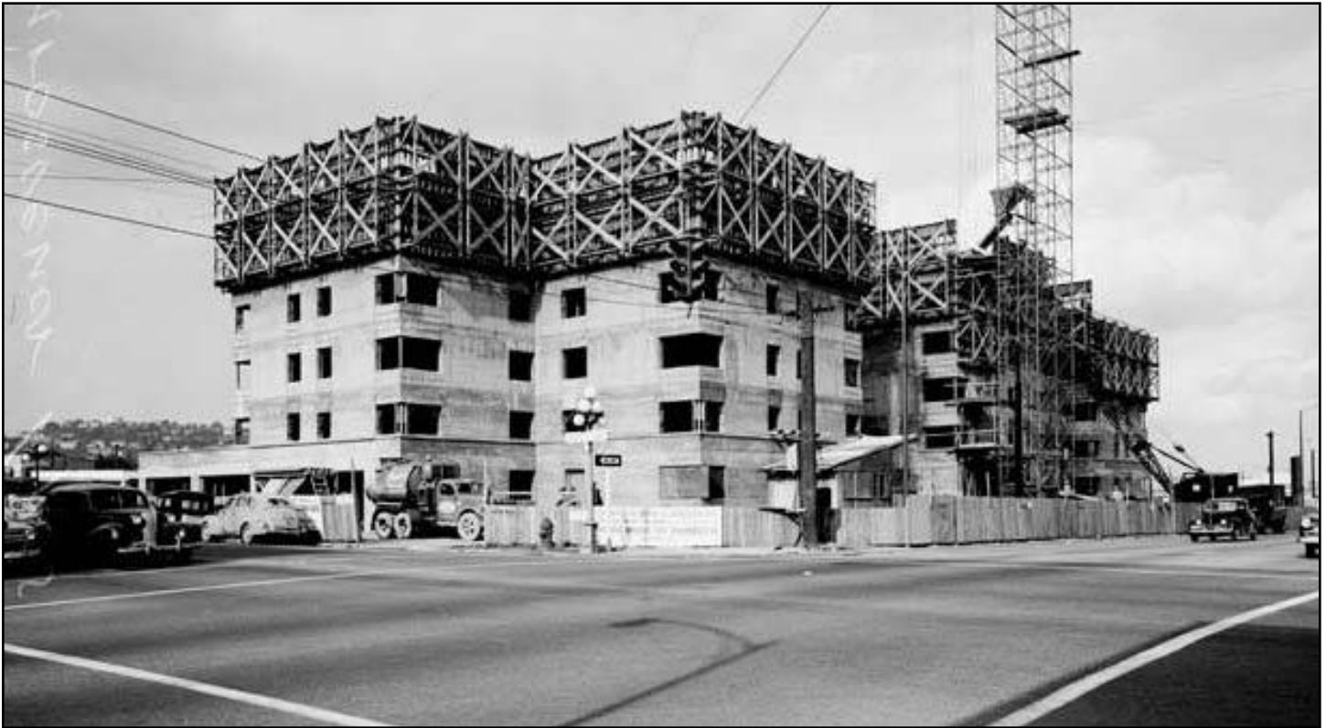
Figure 30 • The Grosvenor House Apartments under construction at 800 Wall Street, 1949
