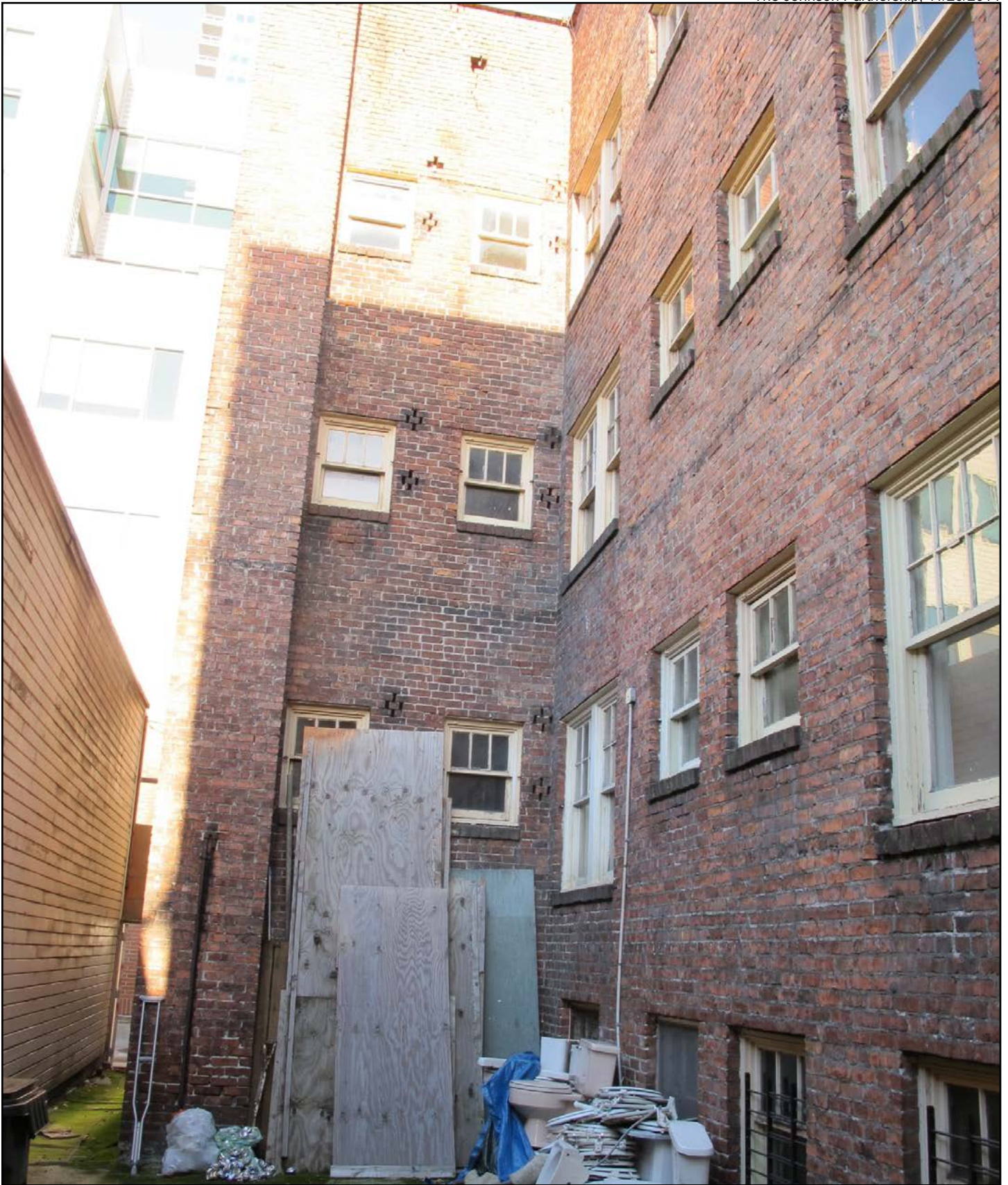
Figure 17 • Franklin Apartment Building, northern lightwell viewing east
