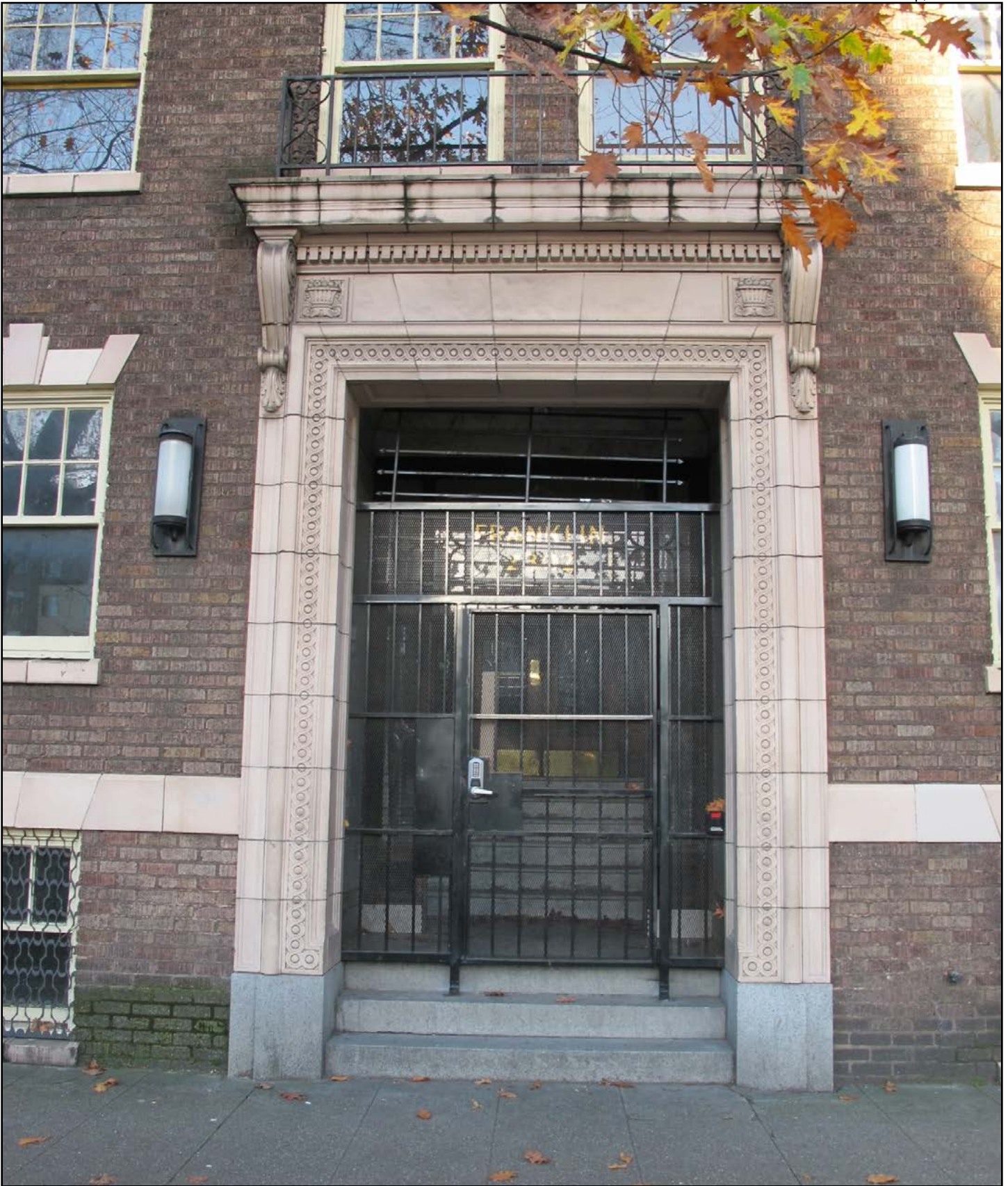
Figure 13 • Franklin Apartment Building, terra cotta at entry on western façade
