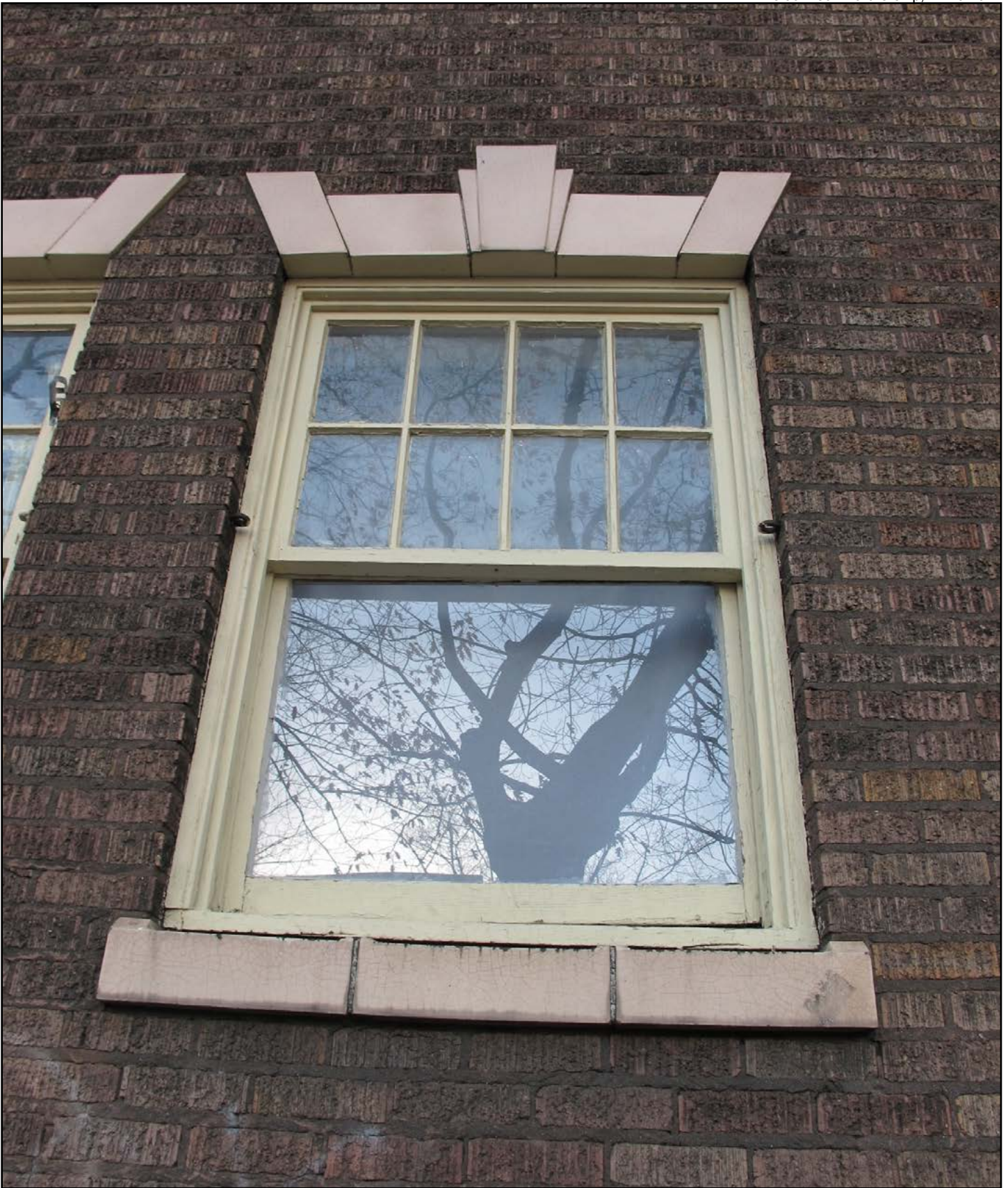
Figure 15 • Franklin Apartment Building, typical window
