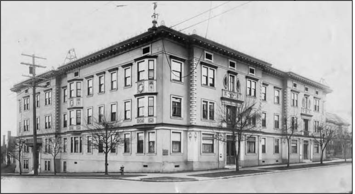
Figure 28 • St. Paul Apartment Building, First Hill, 1901
