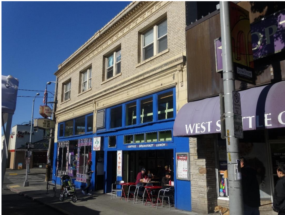
C4: Crescent-Hamm Bldg., east-facing façade. Camera facing SW.
