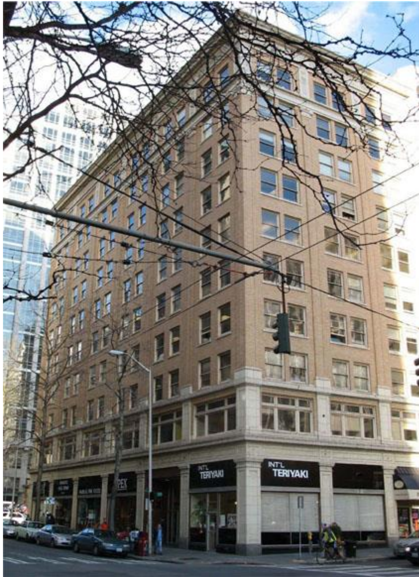
D7: Lloyd Building (1926), 601 Stewart Street. Photo: 2010, Seattle Landmark Nomination.
