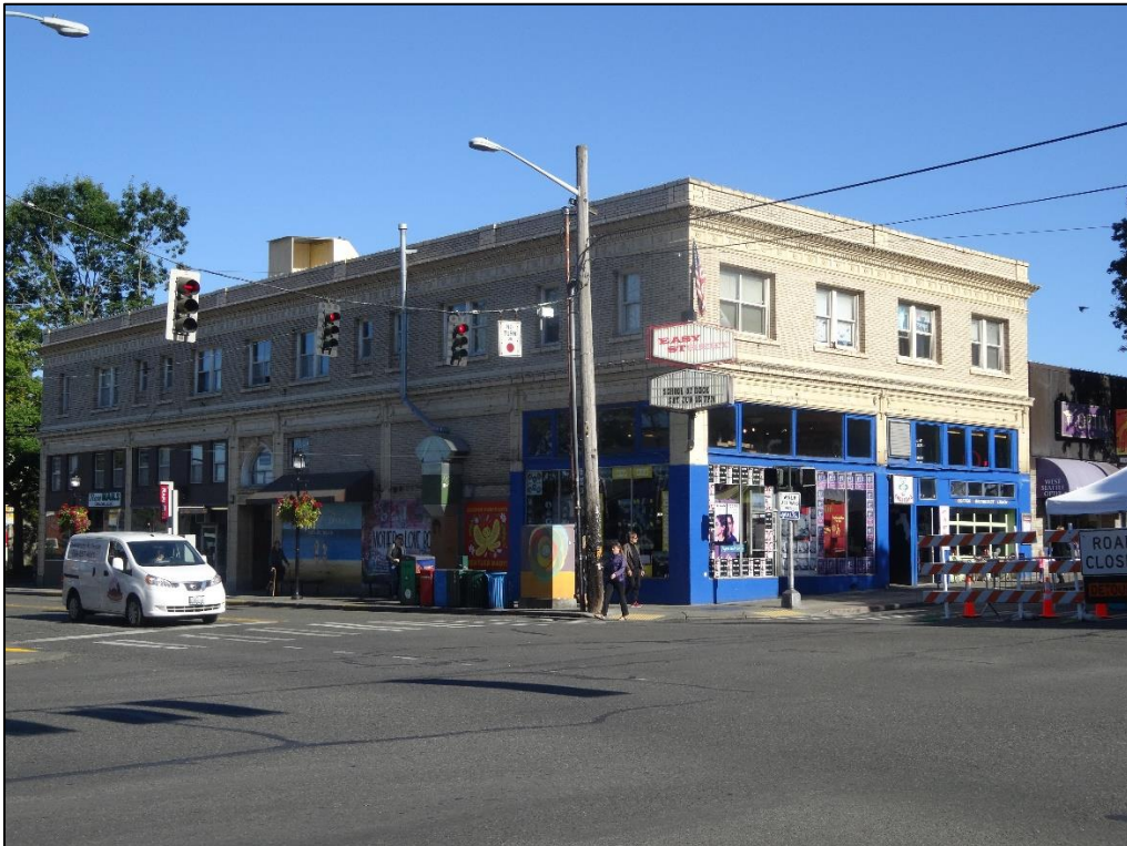
C2: Crescent-Hamm Building. Camera facing NW.
