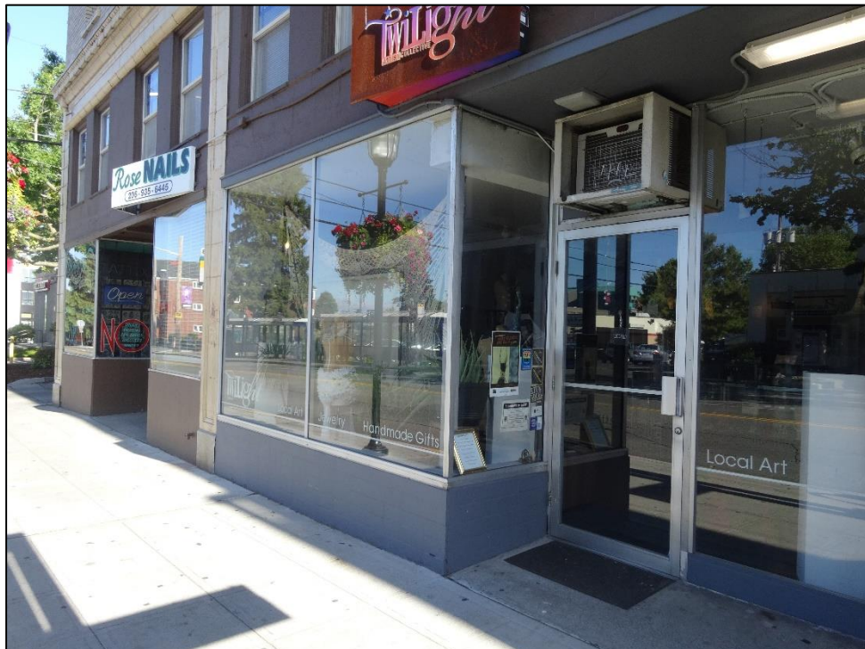
C8: Crescent-Hamm Bldg., storefronts along south elevation. Camera facing NW.
