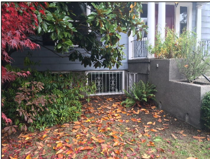
Figure 28. Below, detail view of basement window, and concrete porch steps and cheek blocks.
