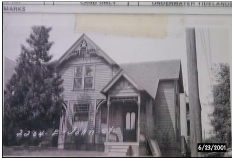
Figure 51 A & B. 2204 E John Street (1890), Parcel 095500-0120 Below left, 1937; below right, current.
