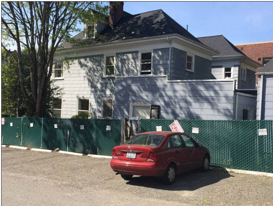
Figure 33. Below, looking northwest at the south facade, back wings, single-story southeast addition and a portion of the detached garage.
