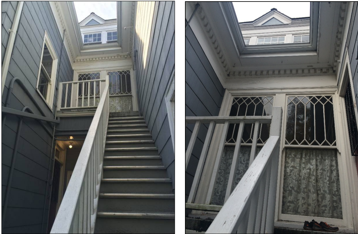
Figures 38. & 39. Above left and right, the opening and exterior stair between the two east wings. Paired windows in the center with decorative divided lights, open onto the interior stair landing, while other windows into the apartments are simpler 1:1 sash. The attic dormer windows visible above.
