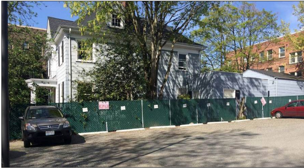
Figure 32. Above, view looking north at the south and part of the west facade.
