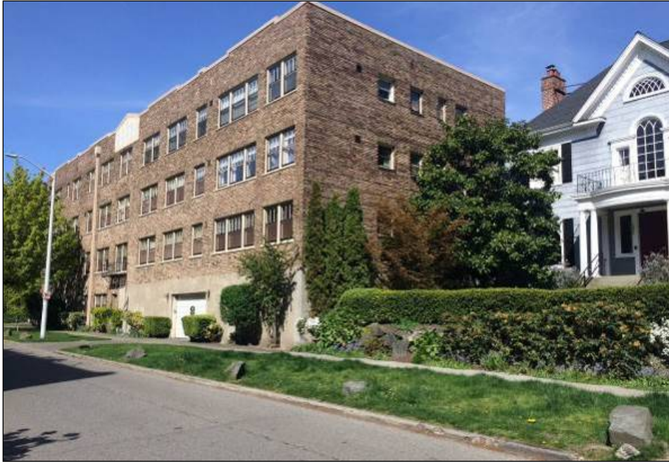
Figure 22. Above, looking northeast at the Marquis Apartments (1926), 1605 E Olive Street.
