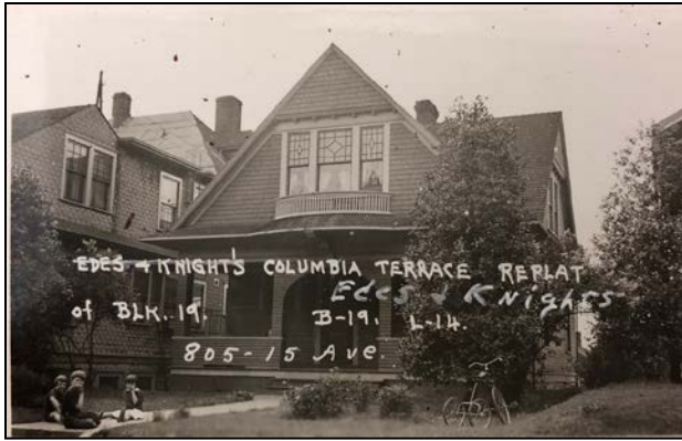
Figures 53 A & B. 805 15 th Avenue (1895), Parcel 1710400070 Below left 805 15 th Avenue (1895), Parcel 171040-0070
