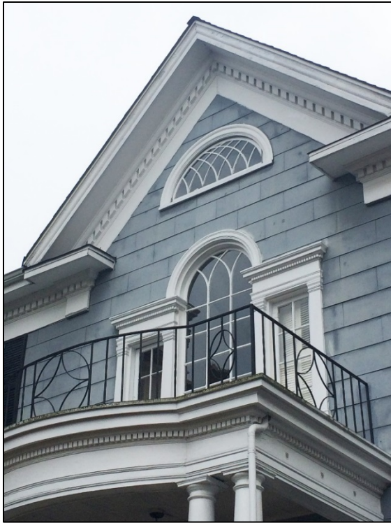
Figure 29. Above, a detail view of the upper story windows and trim, non-original balustrade and siding.
