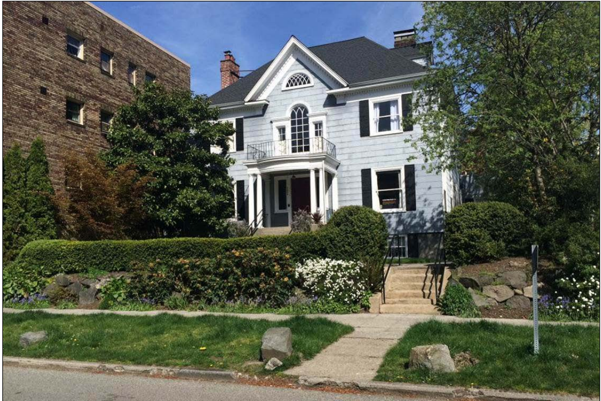
Figure 26. Above, view looking northeast at the primary (west) facade and front yard from 16 th Avenue.
