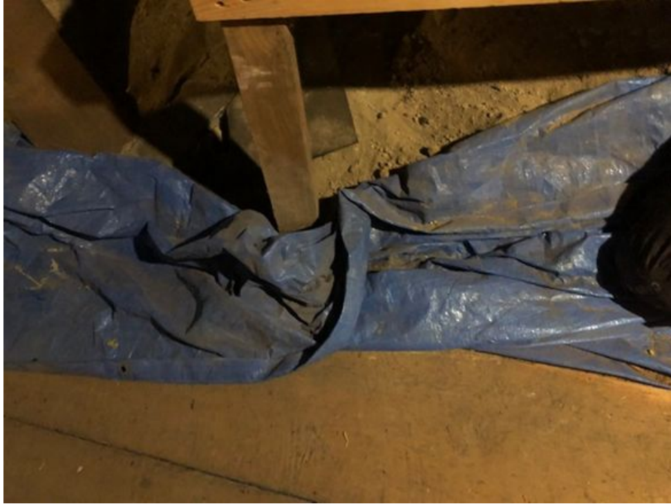
Figure 122. Partial dirt floor in cellar.
