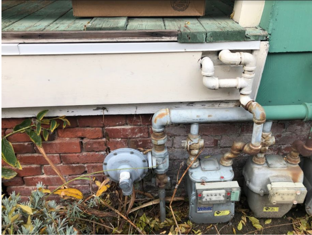
Figure 74. Image of 518 14th Avenue East in 2020, exterior foundation, south side below porch.
