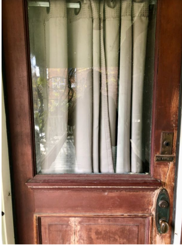
Figure 78. Exterior door (South-facing).
