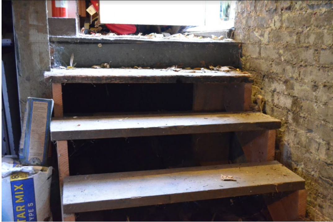
Figure 116. Cellar steps looking up. (Photograph courtesy Ryan Anthony Donaldson, 2020).
