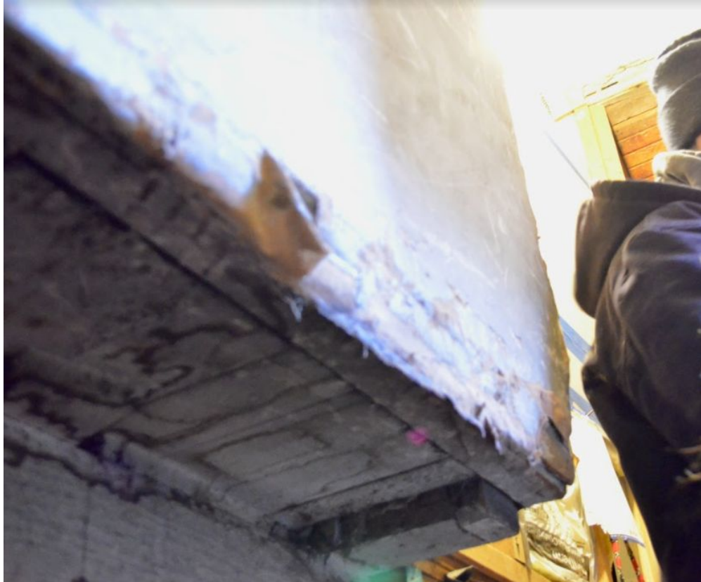
Figure 118. From cellar steps, one can see the wood-joining construction technique used to create the main kitchen floor.
