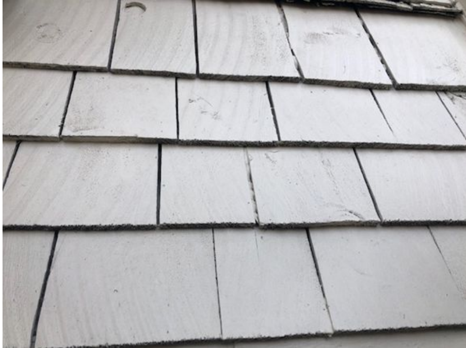
Figure 62. Gable shingles.
