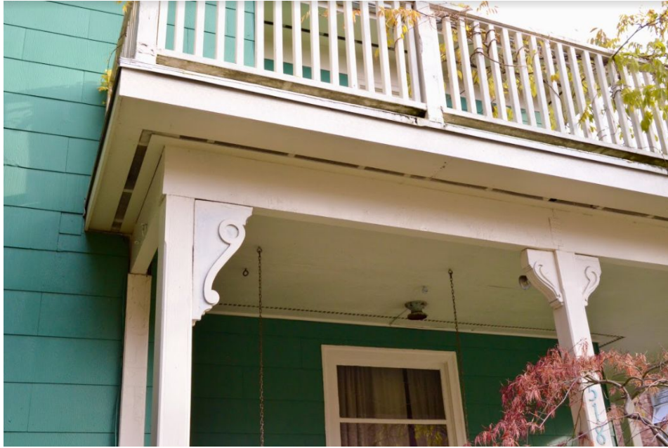
Figure 58. Image of 518 14th Avenue East in 2020, porch detail.
