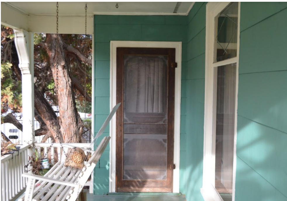
Figure 77. Exterior door (South-facing). (Photograph courtesy Ryan Anthony Donaldson, 2020).
