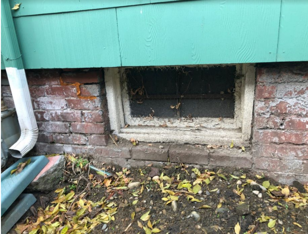
Figure 76. Image of 518 14th Avenue East in 2020, exterior foundation and cellar window.
