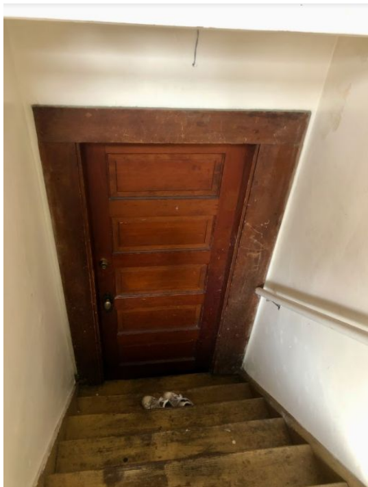
Figure 109. Interior door separating second floor from attic.
