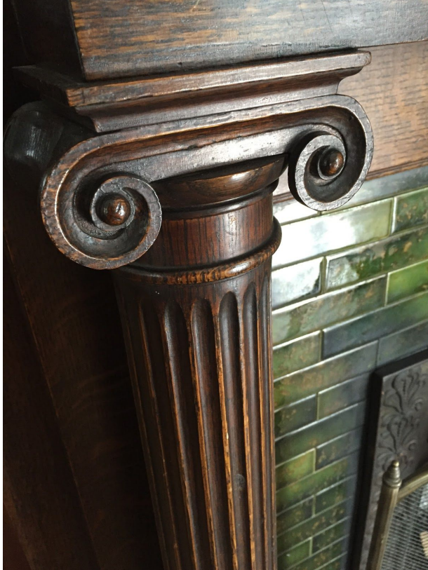
Figure 86. Main floor fireplace detail with original ornamental wood mantel and decorative green tile.
