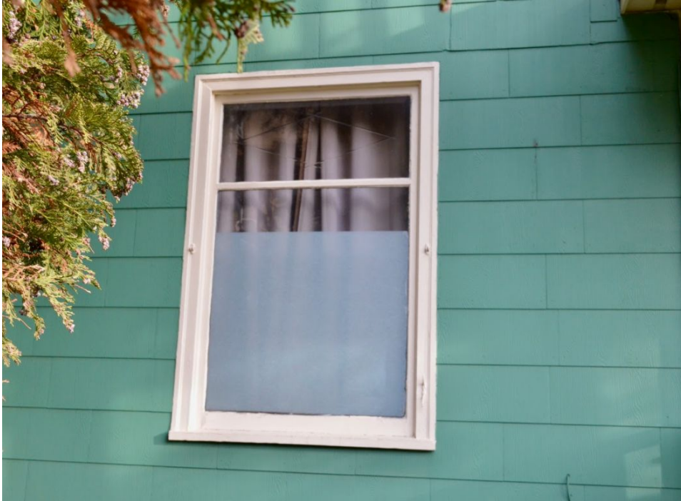
Figure 60. Image of 518 14th Avenue East in 2020, close-up of West-facing window (note where former window awning used to attach).
