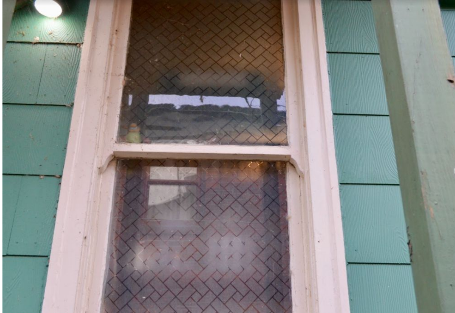
Figure 66. Image of 518 14th Avenue East in 2020, detail of rear (East-facing) window on kitchen.
