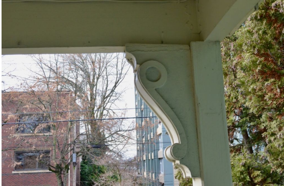
Figure 68. Image of 518 14th Avenue East in 2020, detail of porch bracket. (Photograph courtesy Ryan Anthony Donaldson, 2020).
