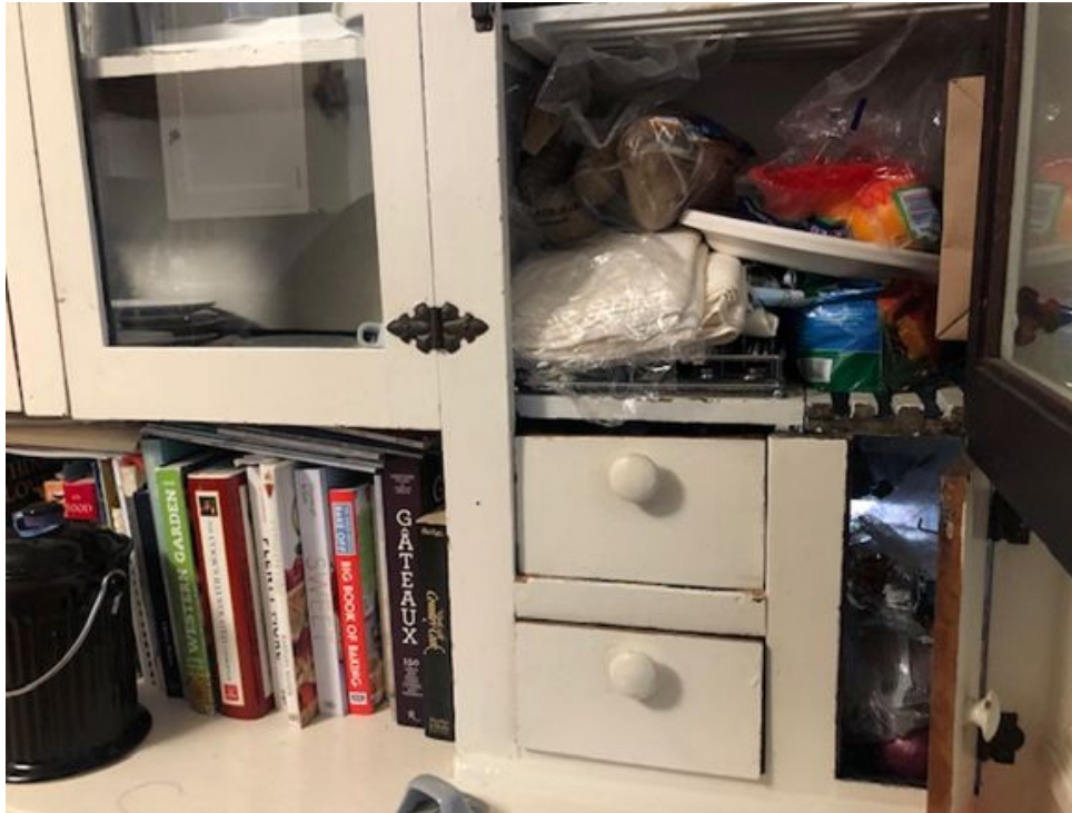
Figure 102. Interior of 518 14th Ave. E., detail of original built-in wood kitchen cabinets with “ice-box” cupboard on lower right (holes allow cold air from outside).
