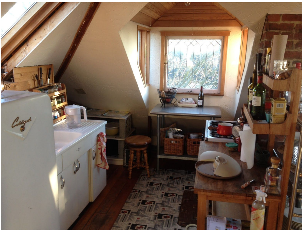
Figure 111. Attic with leaded south-facing dormer window added later. (Note modified kitchen area, which creates a separate unit.) (Photograph courtesy Ryan Anthony Donaldson, 2020).
