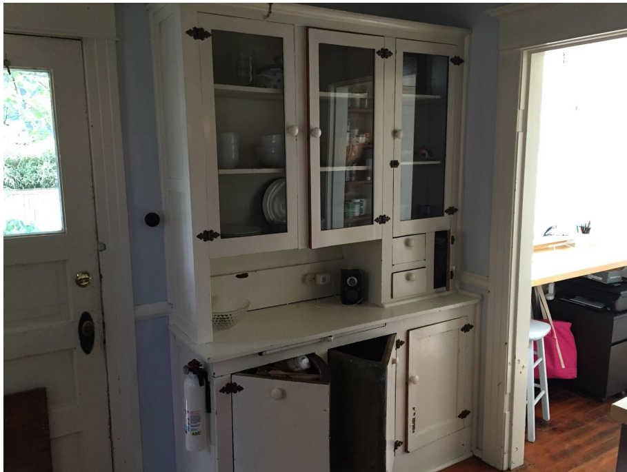
Figure 101. Main floor original built-in wood kitchen cabinets with pull-out flour and produce bins, as well as a cold-storage cabinet
