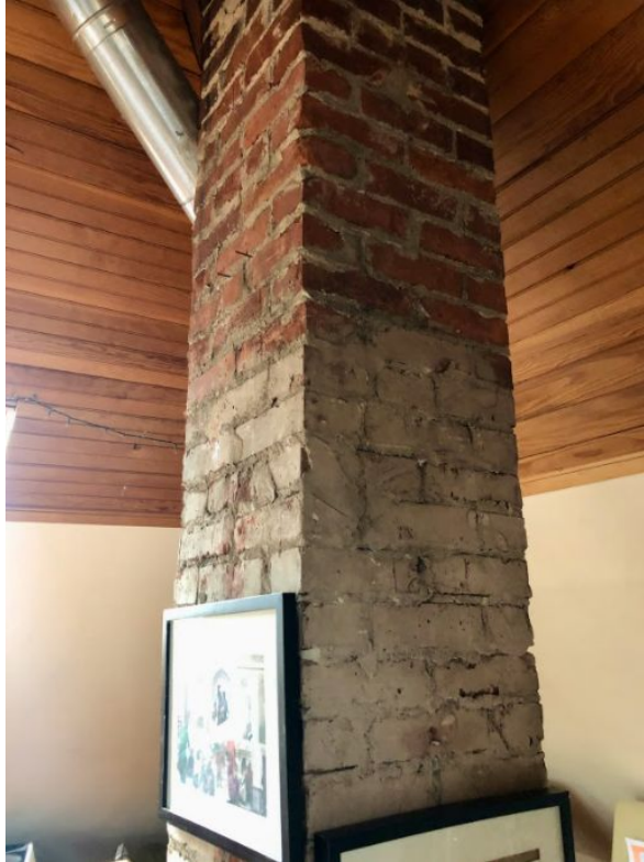
Figure 112. Chimney shaft in attic (note ceiling has been modified).
