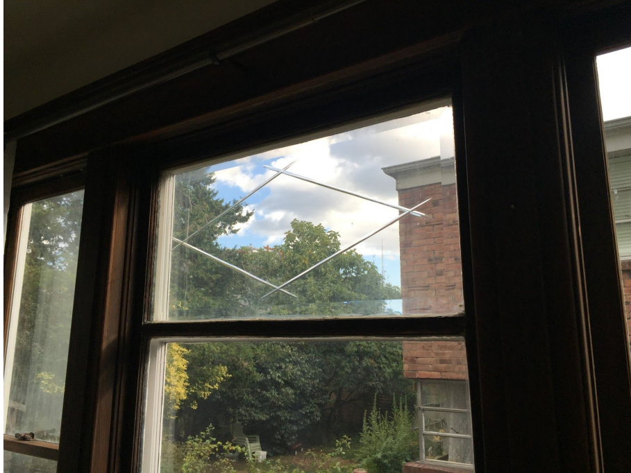
Figure 84. Main floor front room windows with cut-glass design
