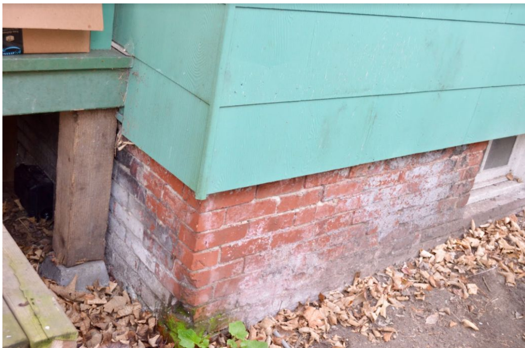
Figure 73. Image of 518 14th Avenue East in 2020, exterior foundation, NE corner.
