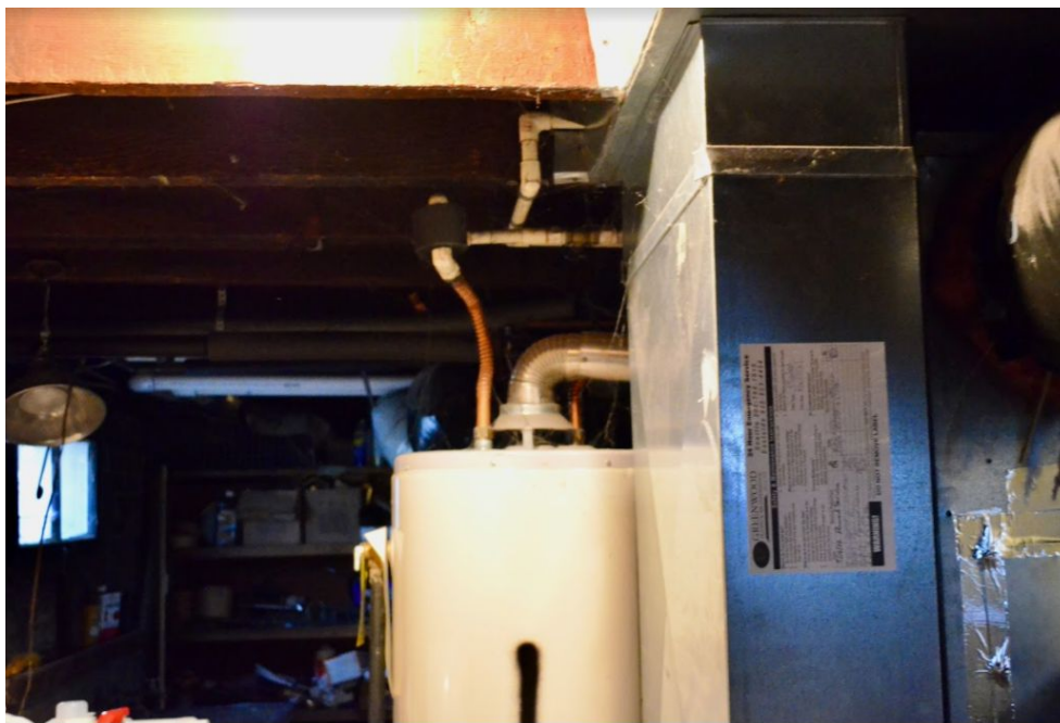
Figure 119. Low-ceilinged cellar with wood rafters; partial concrete-slab and dirt floor.
