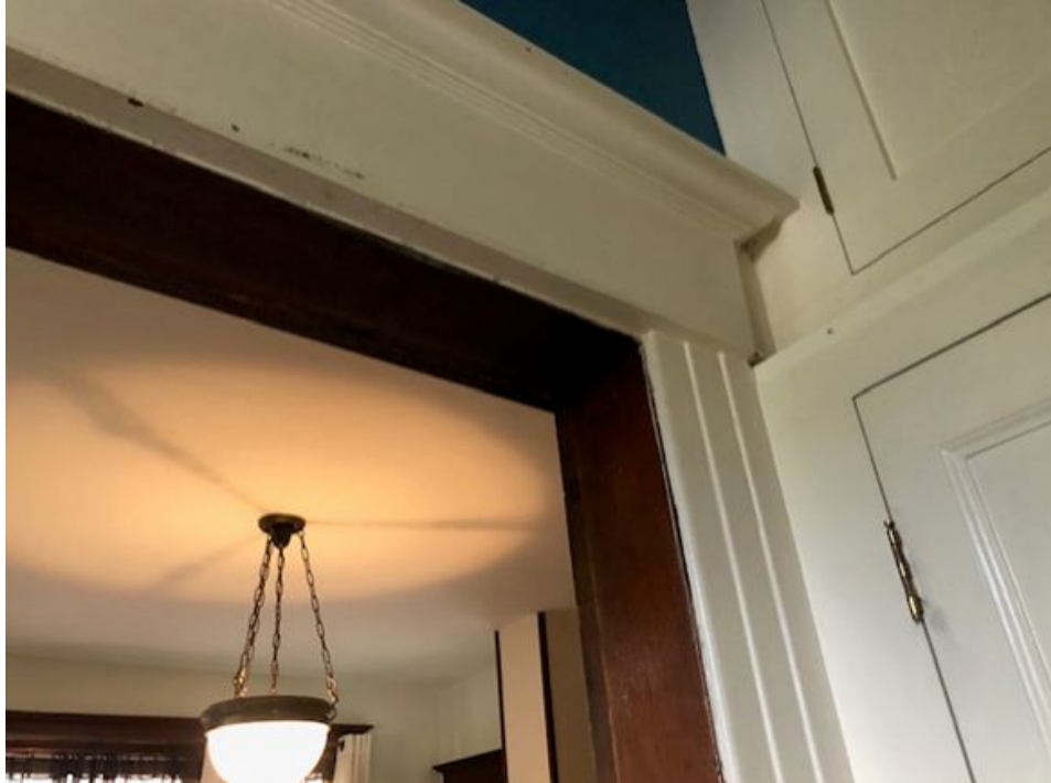
Figure 90. Interior of 518 14th Ave. E., detail above doors.
