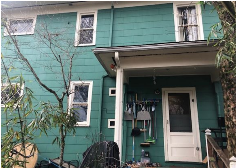
Figure 69. Image of 518 14th Avenue East in 2020, rear. Note the small square holes between the window and porch door--these provide cold air to the "ice-box" built-in cupboard in the kitchen.
