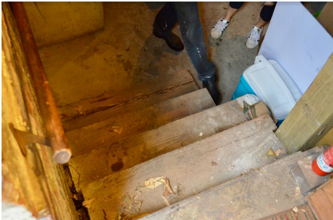
Figure 117. Cellar steps looking down.
