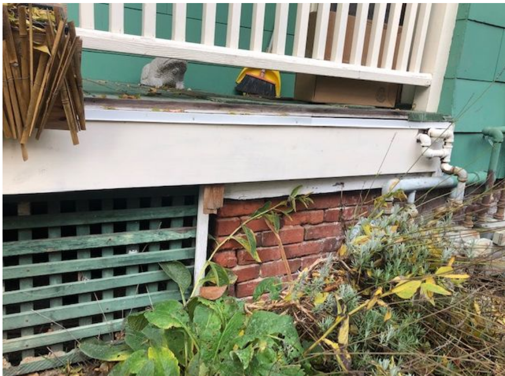
Figure 75. Image of 518 14th Avenue East in 2020, exterior foundation, south side below porch.
