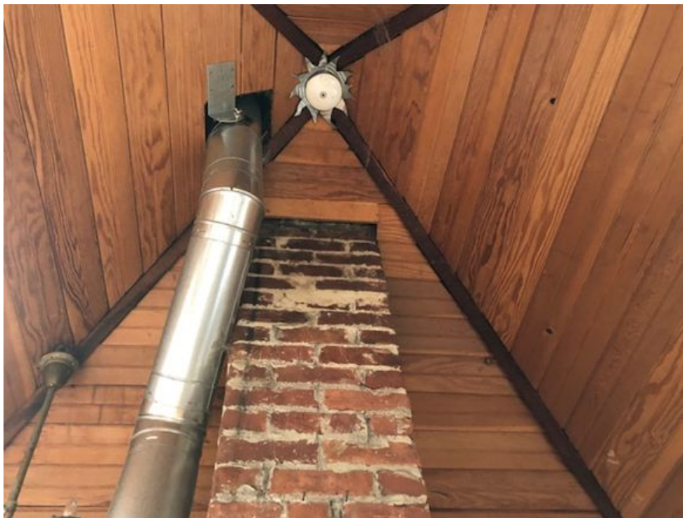
Figure 113. Chimney shaft in attic (note ceiling has been modified).
