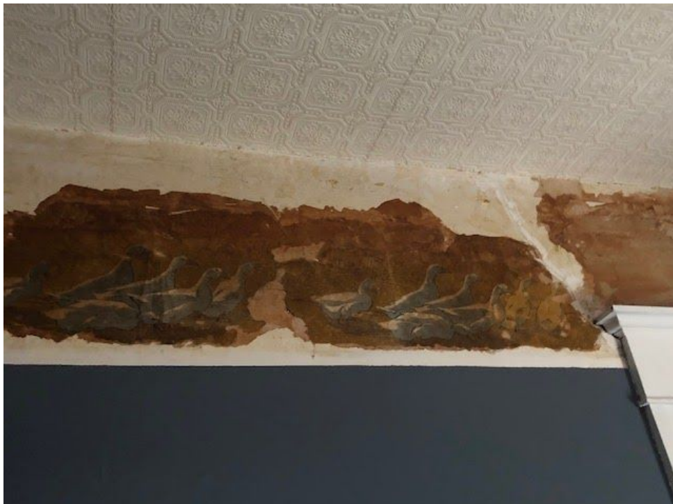
Figure 107. Interior of 518 14th Ave. E. in 2020: Second floor bedroom with recently discovered original children's wallpaper (note the tin ceiling is a contemporary modification).
