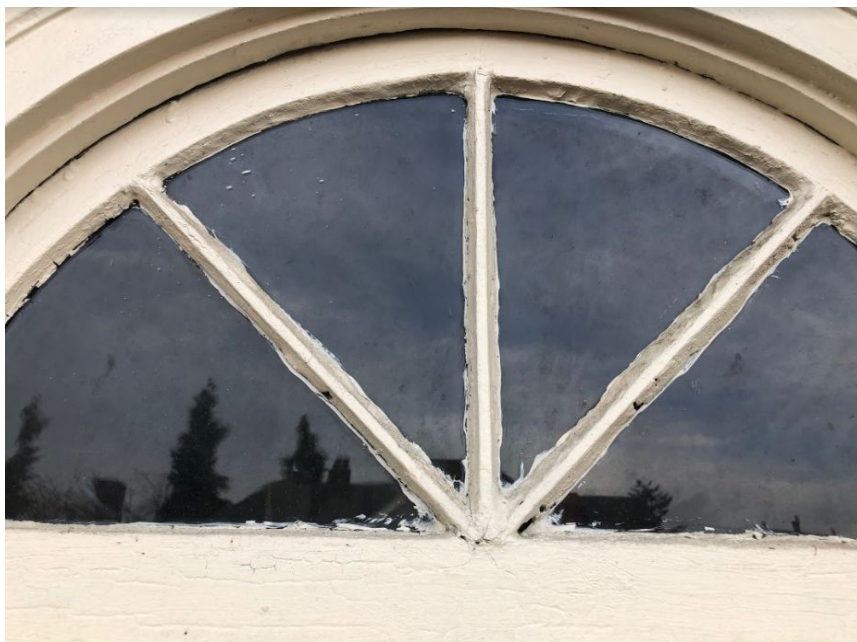
Figure 63. Close-up of gable window.
