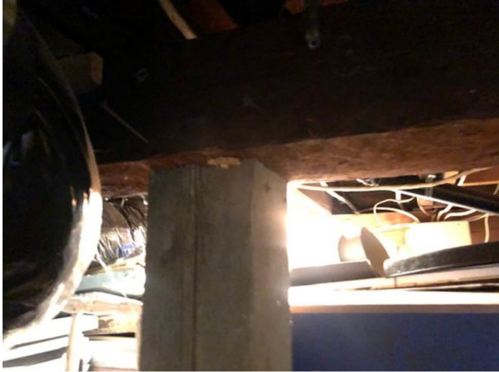
Figure 120. Cellar support post.
