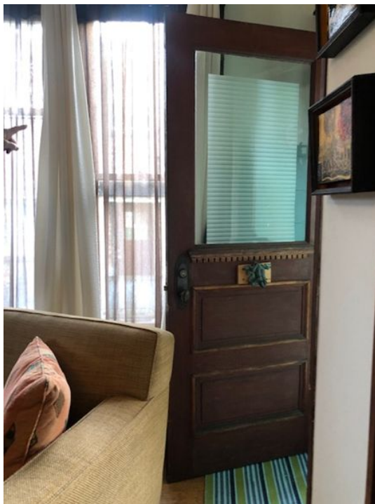
Figure 79. Exterior door (West-facing).
