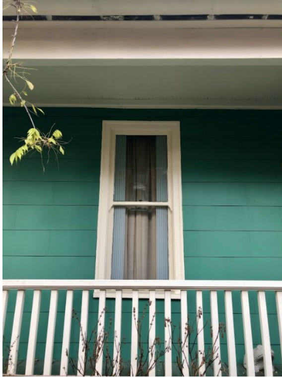
Figure 64. Image of 518 14th Avenue East in 2020, detail of South-facing window.
