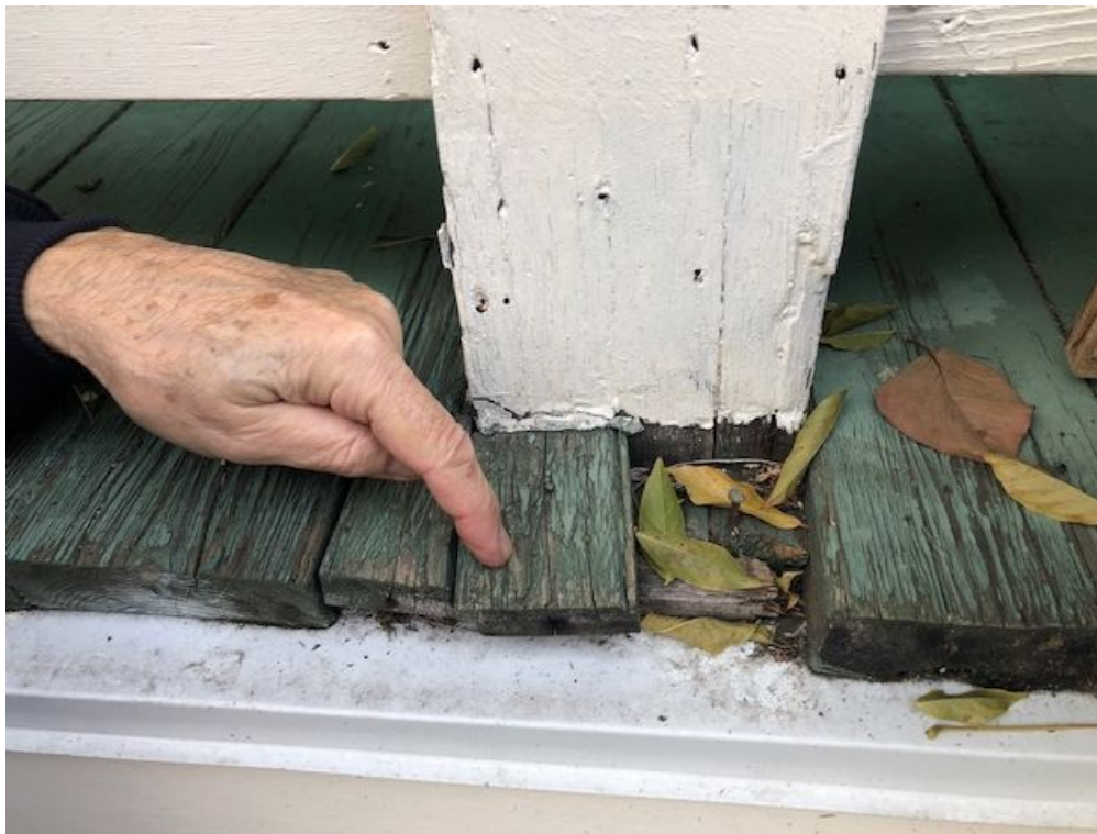
Figure 59. Porch floor boards.
