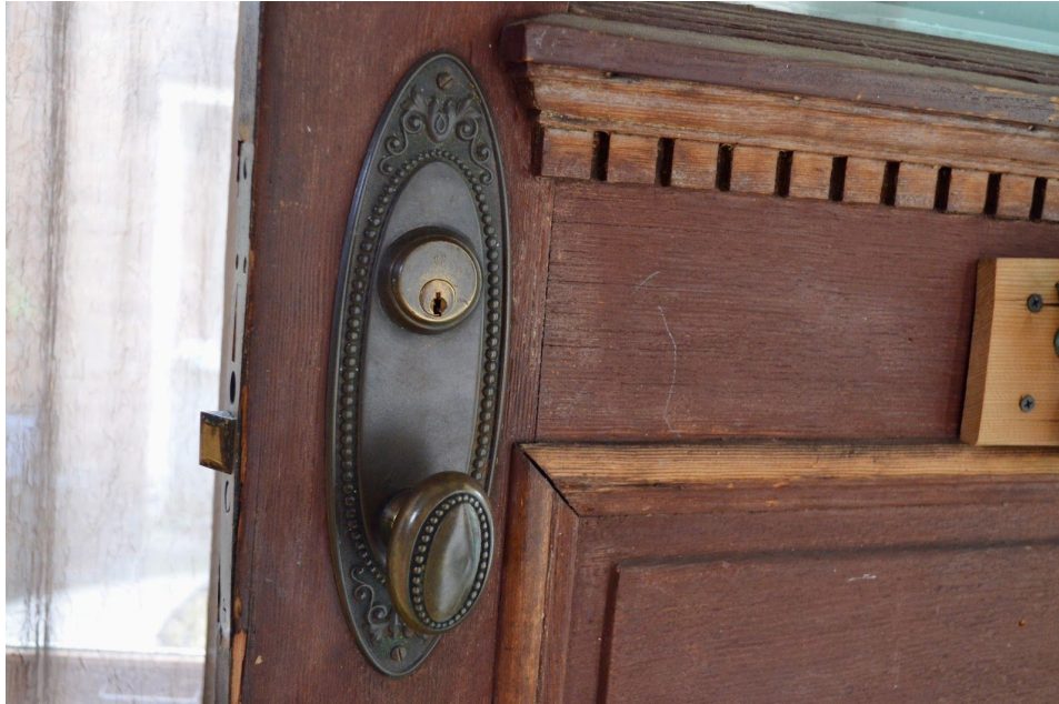
Figure 80. Exterior door (West-facing) detail and doorknob.
