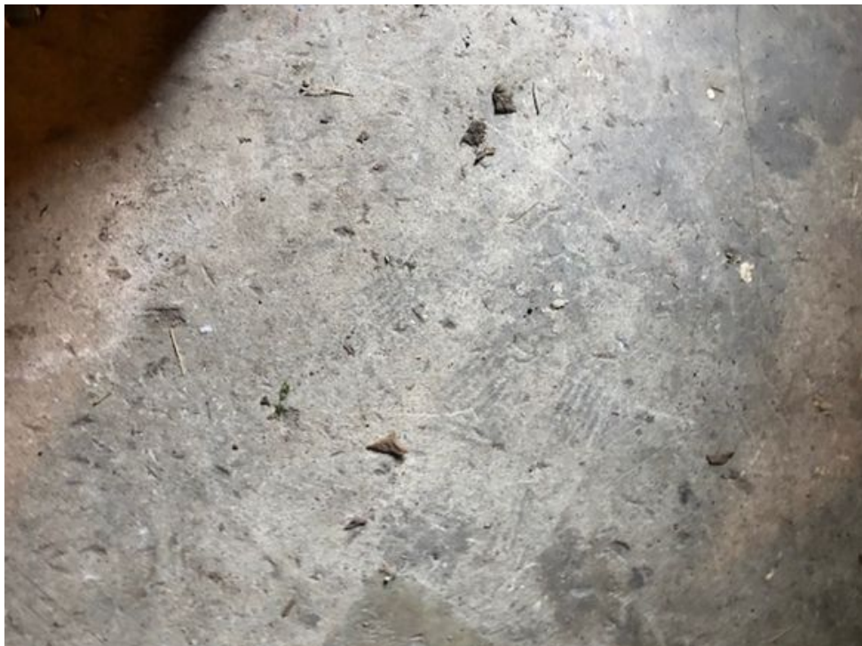
Figure 123. Partial cement slab floor in cellar, added later.
