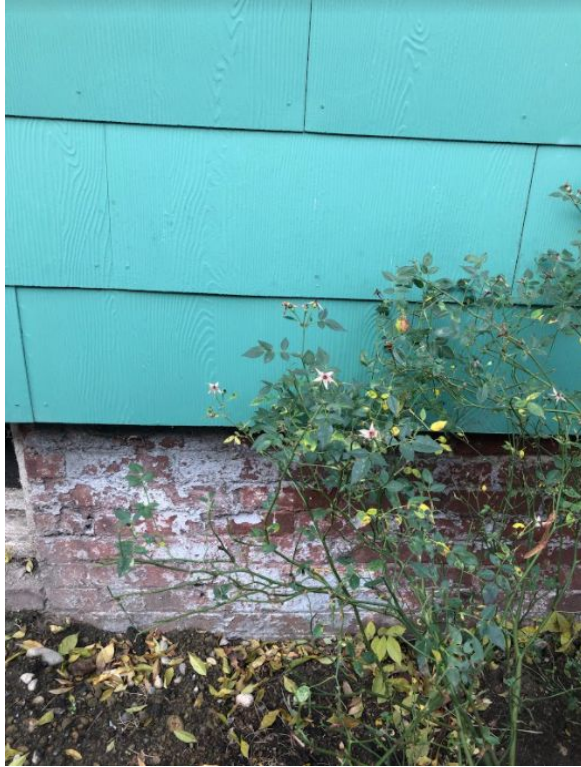
Figure 72. Image of 518 14th Avenue East in 2020, exterior foundation.
