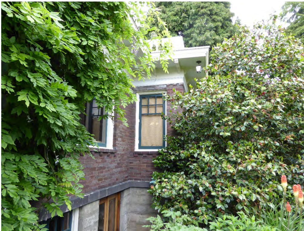
Fig. 10 South Elevation – Conservatory Wing [May 2015]
