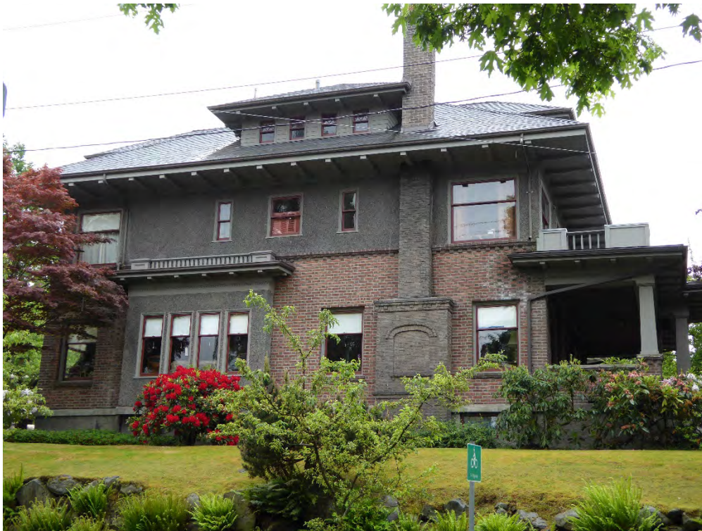
Fig. 59 SIMILAR PROPERTY: Residence at 2836 Harvard Ave. E., 1908 [May 2015]
