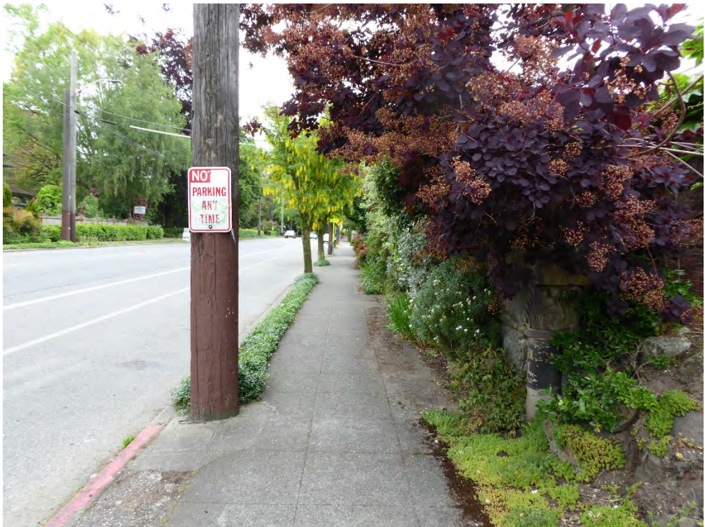
Fig. 26 SITE DETAIL - Historic sandstone retaining wall at Tenth Ave E. [May 2015]
