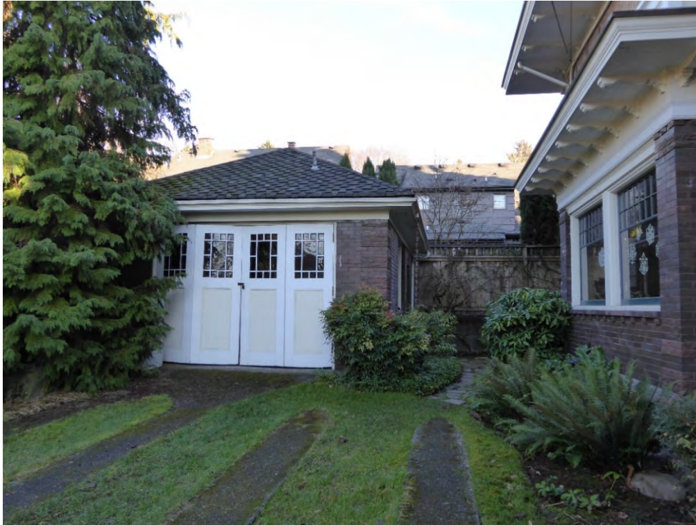
Fig. 23 GARAGE - View of West Elevation (Jan 2015)
