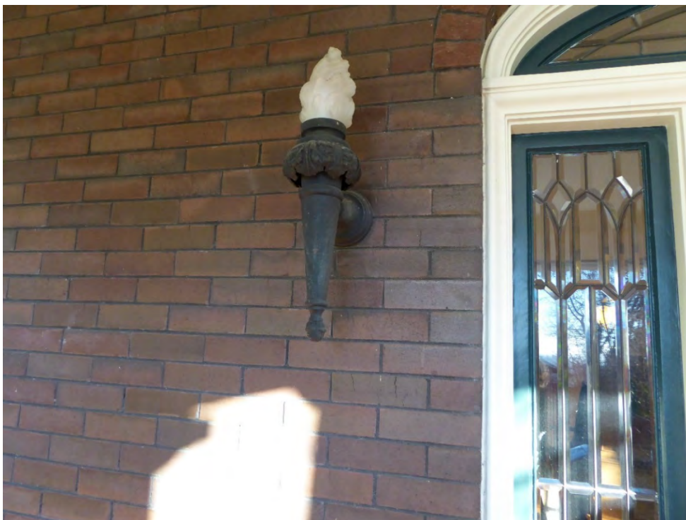
Fig. 22 Detail: Typical historic sconce lighting fixture at entry door (Jan 2015)
