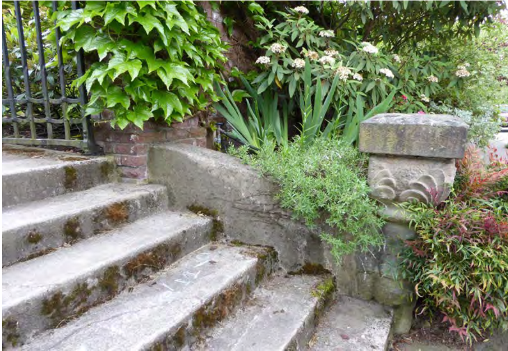
Fig. 27 SITE DETAIL - Historic entrance stairs & sandstone retaining wall [May 2015]
