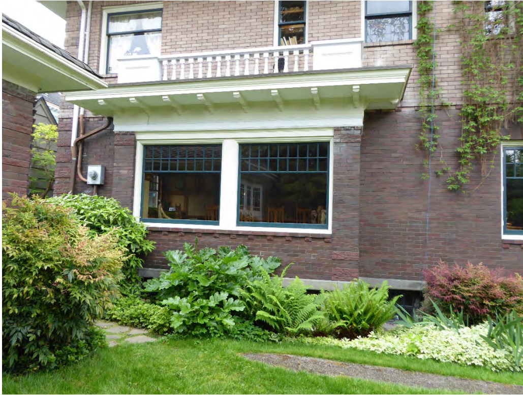
Fig. 15 North Elevation – East end at Dining Room [May 2015]
