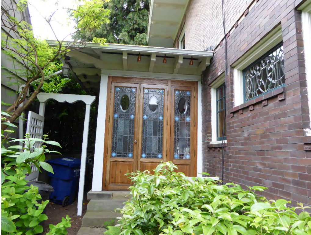
Fig. 14 North Elevation at Rear Porch & East Elevation at Main Wing/Dining Room [May 2015]
