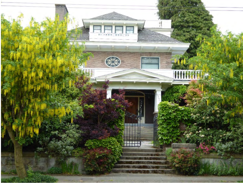
Fig. 7 Entry Stairs & West Elevation [May 2015]
