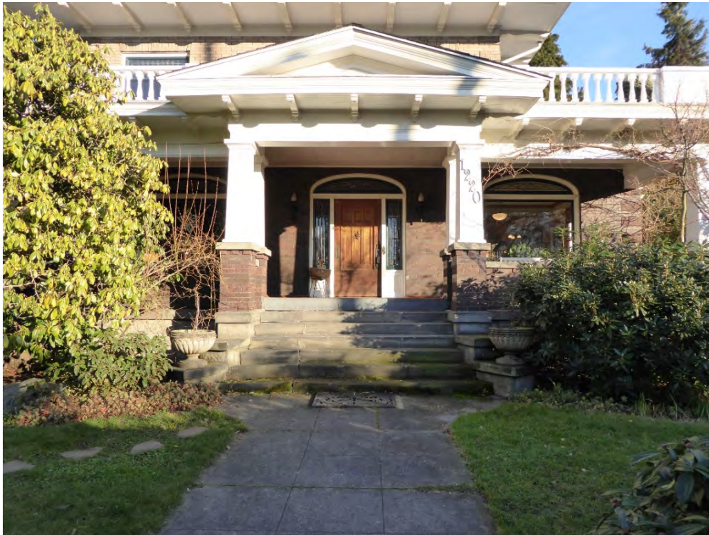
Fig. 8 Entrance Porch – West Elevation (Jan 2015)
