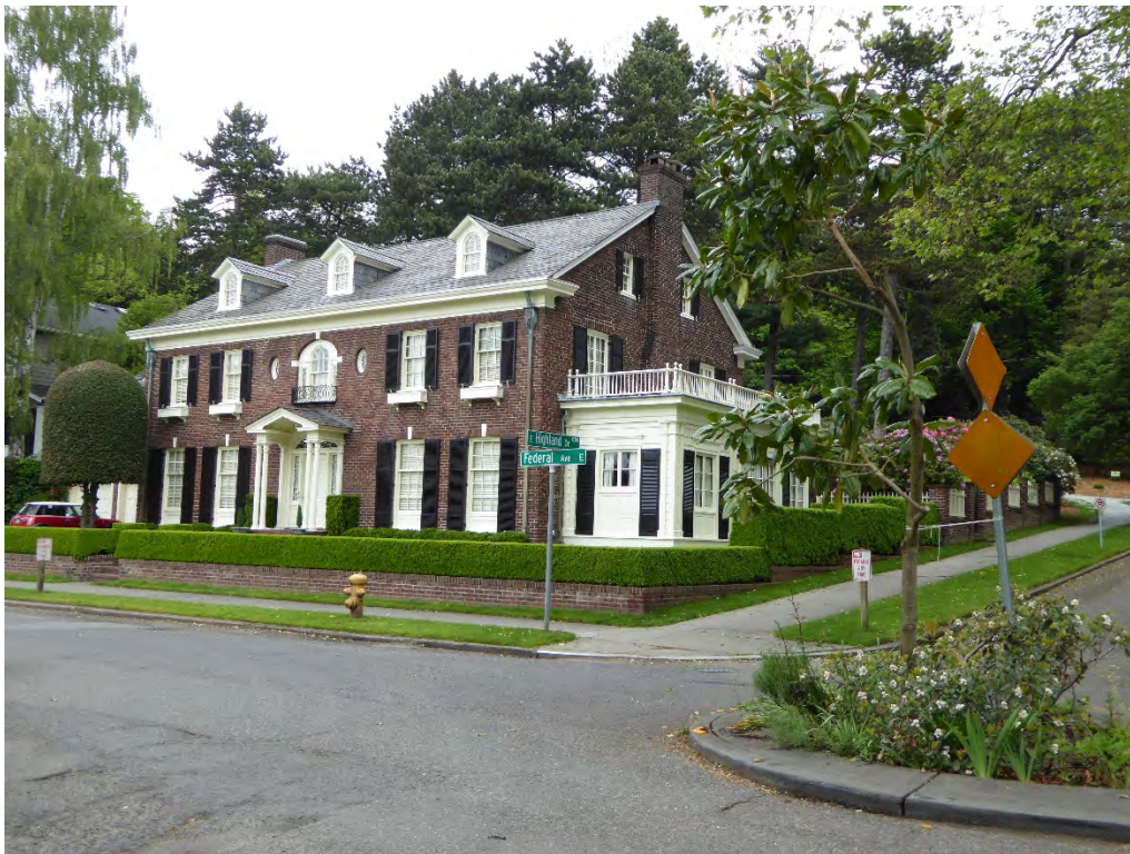
Fig. 55 NEIGHBORHOOD CONTEXT: Dr. Frederick Bentley House at 1204 Federal Ave. E (Joseph Cote, 1914) [May 2015]
