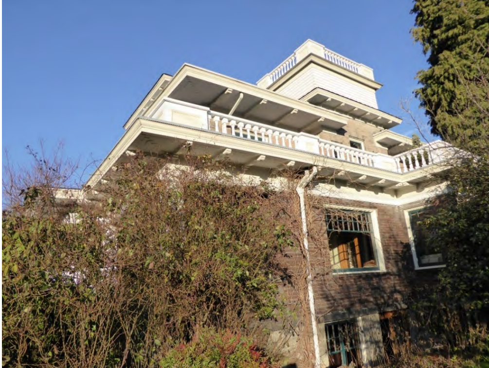
Fig. 9 South Elevation - West end (Jan 2015)
