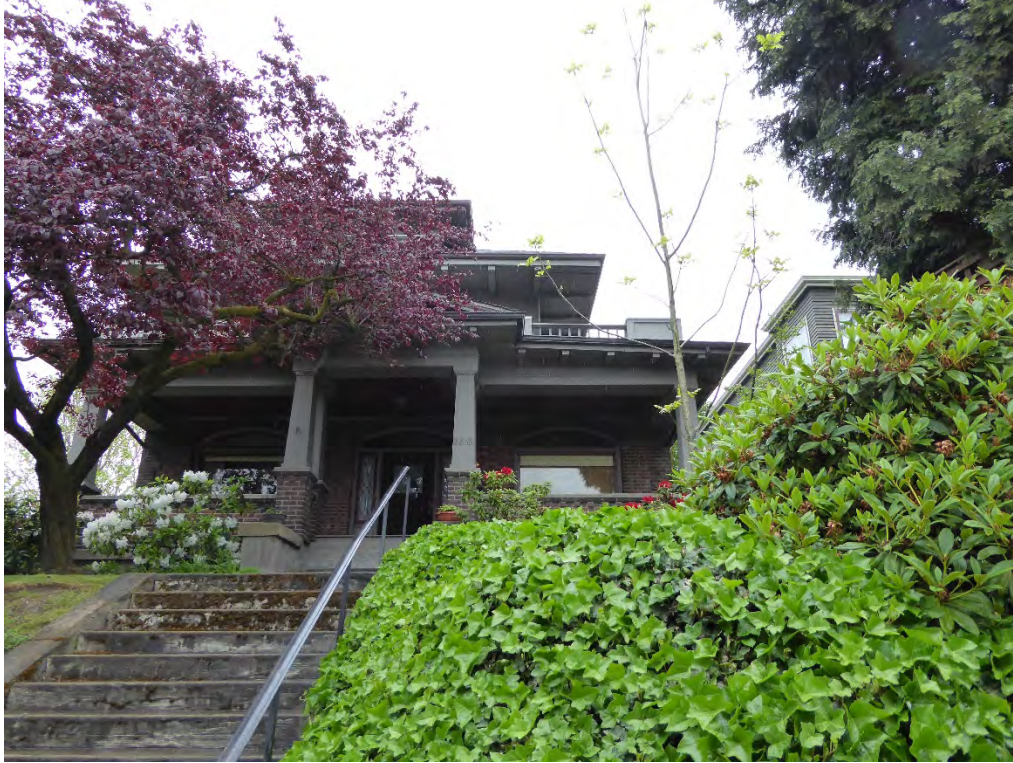
Fig. 58 SIMILAR PROPERTY: Residence at 2836 Harvard Ave. E., 1908 [May 2015]
