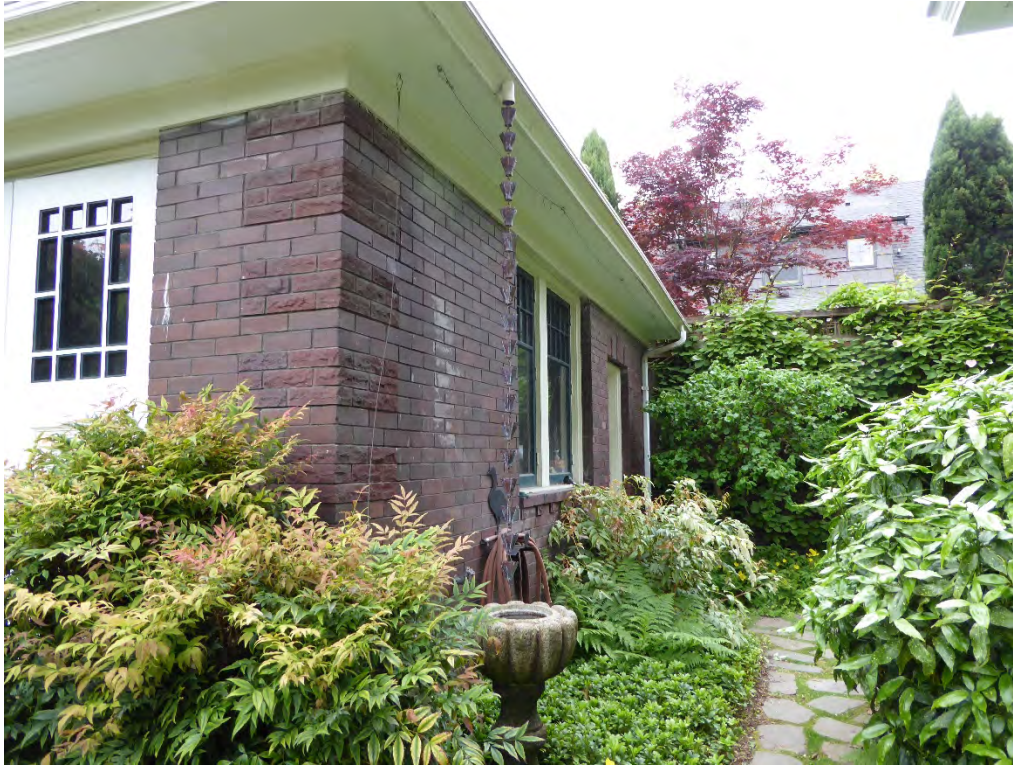
Fig. 25 GARAGE – South Elevation [May 2015]
