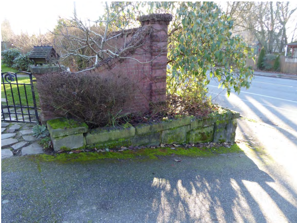
Fig. 28 SITE DETAIL - Historic sandstone retaining wall & brick masonry sound barrier (Jan 2015)
