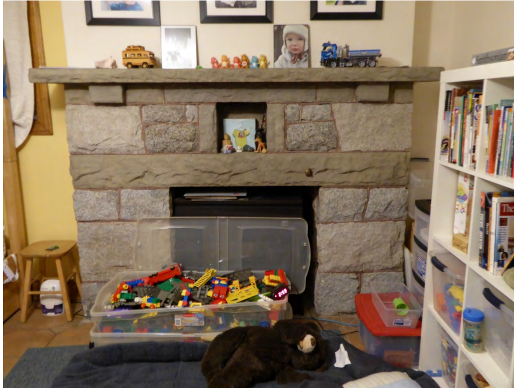
Fig. 52 Fireplace (Sandstone) at Basement level (Jan 2015)
