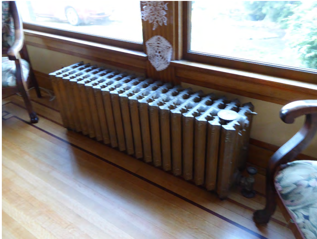
Fig. 53 Typical historic heat register (Jan 2015)
