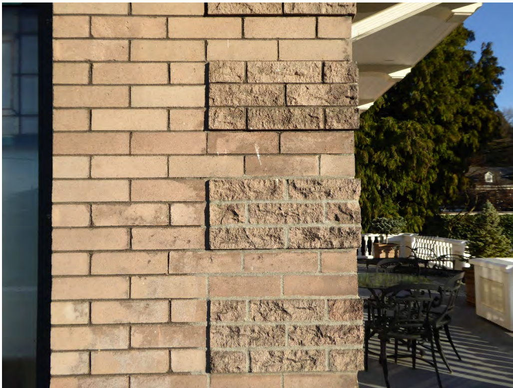
Fig. 20 Detail: Typ. Quoin Details at corners (Jan 2015)
