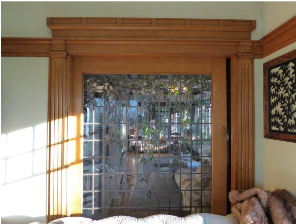
Fig. 41 Study – View East of Stained Glass door leading to former Conservatory (Jan 2015)
