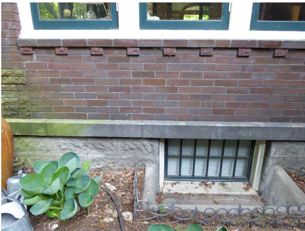
Fig. 18 Typical concrete foundation wall & window well [May 2015]
