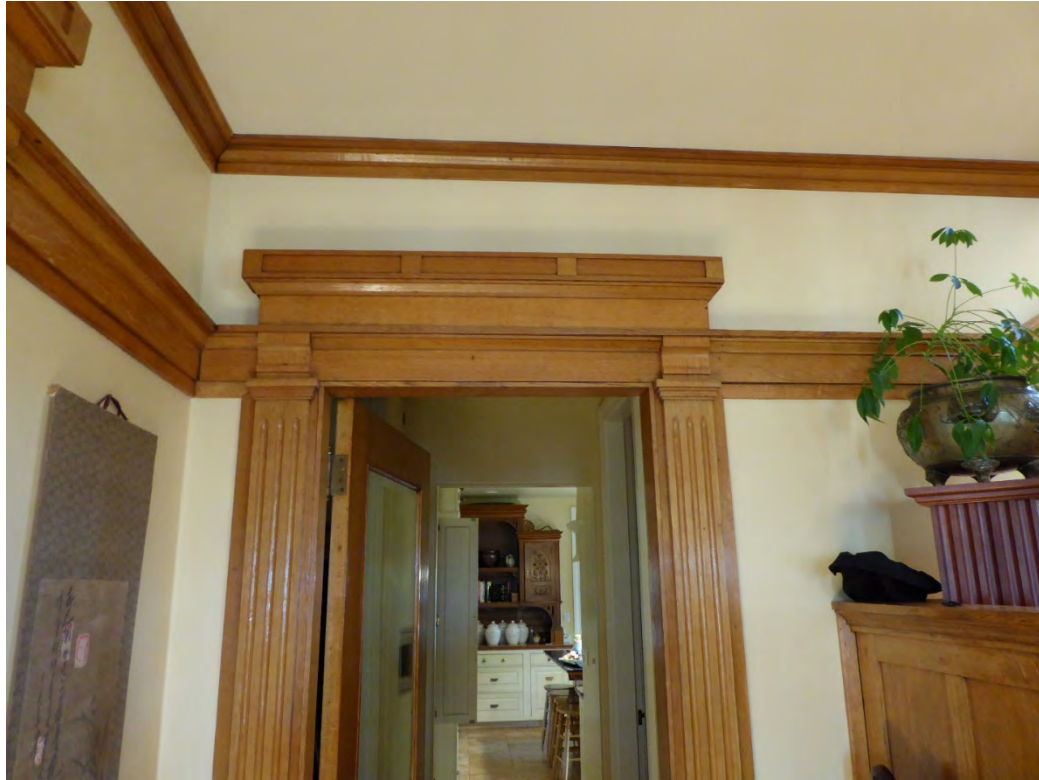
Fig. 38 Typical running & standing Golden Oak trim at First Floor (Jan 2015)
