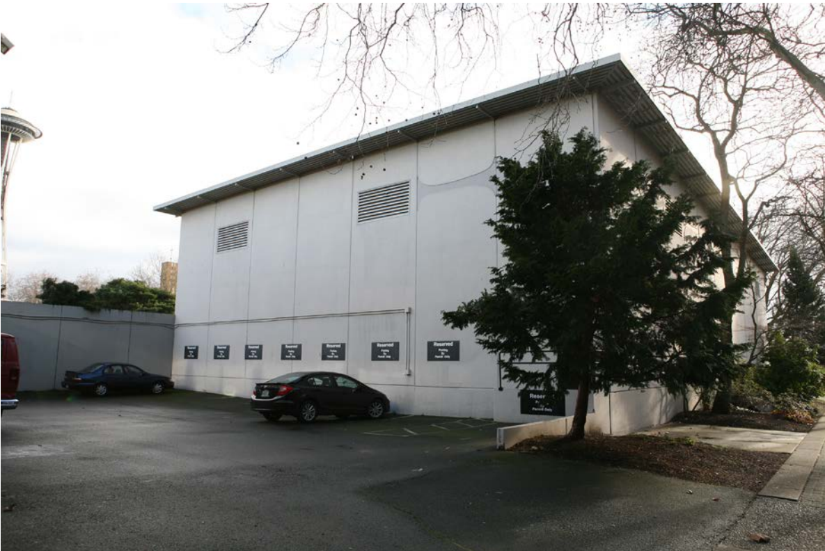
Photograph 30: 2017 view of the north elevation of the NASA Building. Courtesy Artifacts Consulting, Inc.
