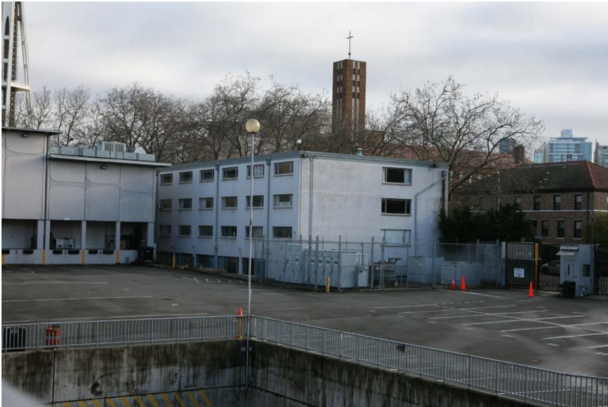
Photograph 39: 2017 view of the northwest corner of the Blue Spruce Building. Courtesy Artifacts Consulting, Inc.
