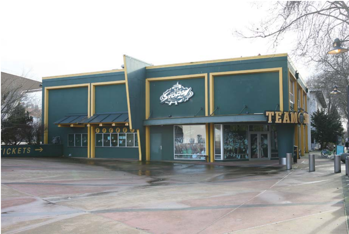
Photograph 31: 2017 view of the north elevation of the West Court Building. Courtesy Artifacts Consulting, Inc.
