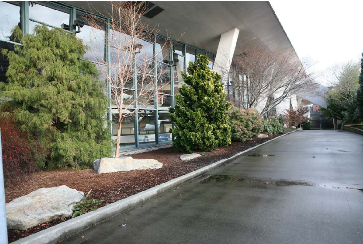
Photograph 25: 2017 view looking along the south elevation of KeyArena. Courtesy Artifacts Consulting, Inc.
