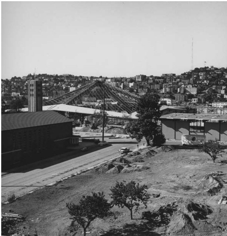
Photograph 4: Coliseum construction, 1961. Courtesy Seattle Municipal Archives, #167426.
