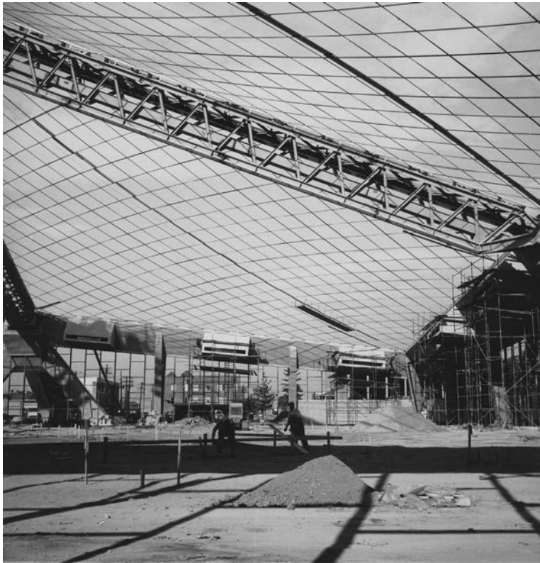
Photograph 3: Coliseum construction, 1961. Courtesy Seattle Municipal Archives, #167424.
