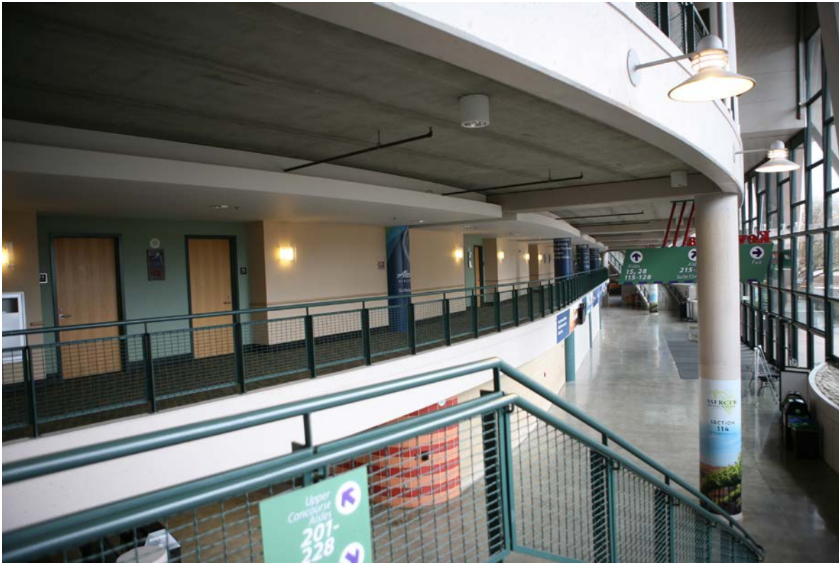
Photograph 49: 2017 view of suite level in KeyArena. Courtesy Artifacts Consulting, Inc.
