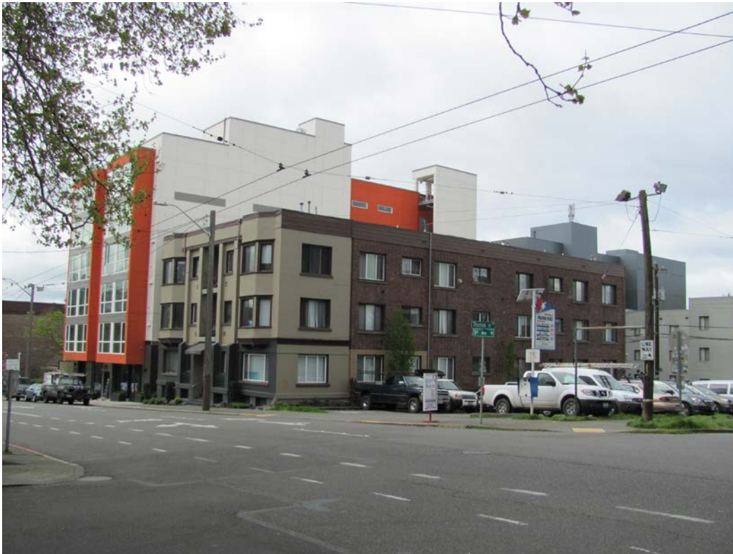
Photograph 61: View looking southwest from the southwest corner of the NASA Pavilion towards the parking lot and buildings occupying the eastern half of the block bounded by 1st Avenue N., Thomas Street, Queen Anne Avenue, and John Street. Courtesy Artifacts Consulting, Inc.
