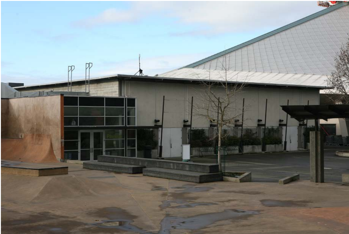
Photograph 41: 2017 view of the southeast corner of the Seattle Center Pavilion and the Skatepark which stands on the site of the former British Pavilion. Courtesy Artifacts Consulting, Inc.
