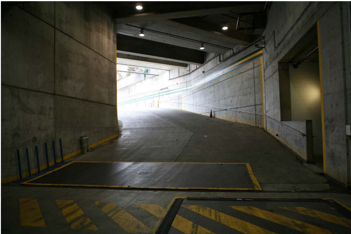
Photograph 50: 2017 view of KeyArena loading dock. Courtesy Artifacts Consulting, Inc.
