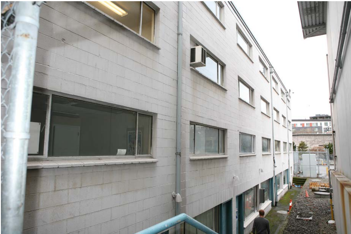
Photograph 40: 2017 view looking west along the north elevation of the Blue Spruce Building. Courtesy Artifacts Consulting, Inc.
