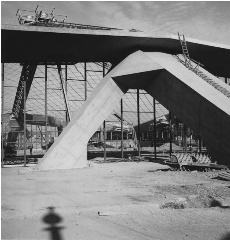
Photograph 21: Coliseum construction photograph. Courtesy Seattle Municipal Archives, #167425.
