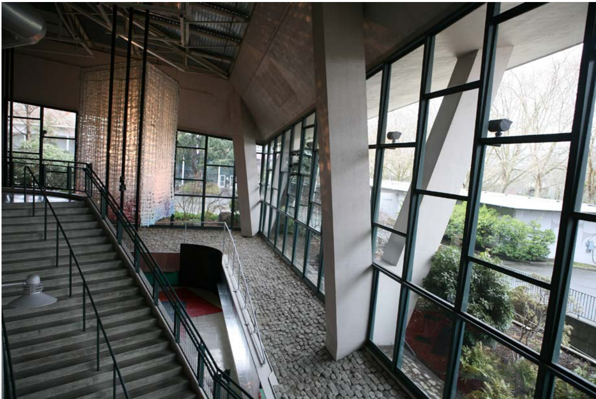
Photograph 46: 2017 interior view of KeyArena, showing glass curtain wall, concrete supports, and cobblestones. Courtesy Artifacts Consulting, Inc.
