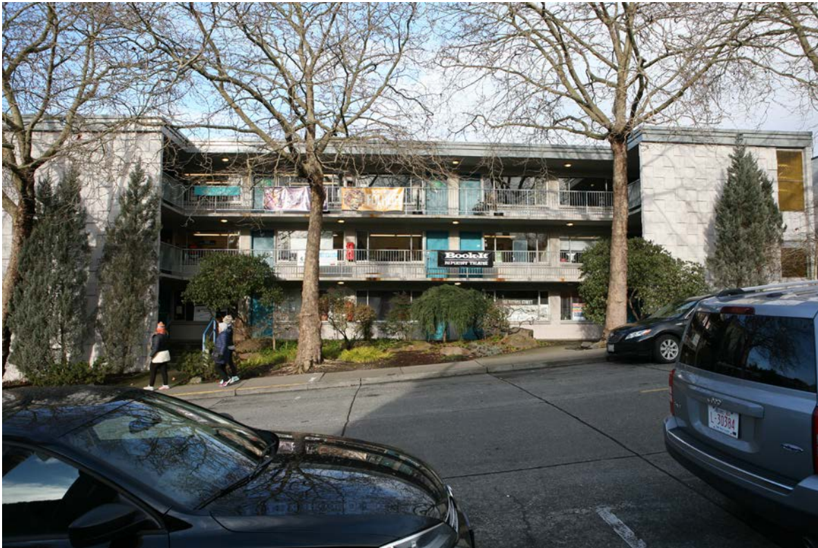
Photograph 37: 2017 view of the south elevation of the Blue Spruce Building. Courtesy Artifacts Consulting, Inc.
