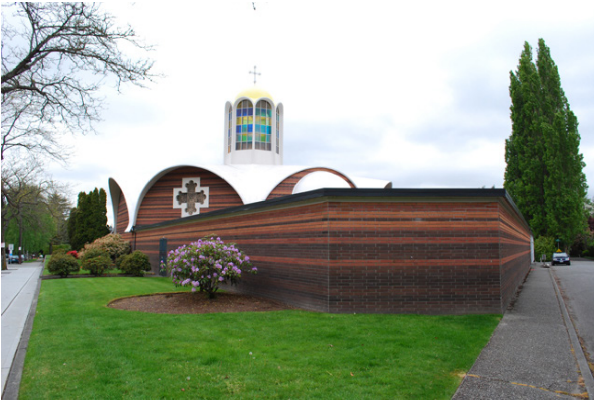
Photograph 65: Example of Paul Thiry's design and Paul Hostmark's structural engineering work. Saint Demetrios Greek Orthodox Church, Seattle, 1963. Courtesy the Department of Archaeology and Historic Preservation.
