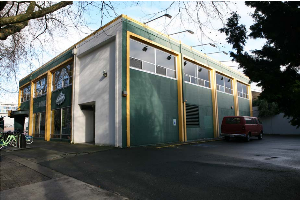
Photograph 34: 2017 view of the southwest corner of the West Court Building. Courtesy Artifacts Consulting, Inc.
