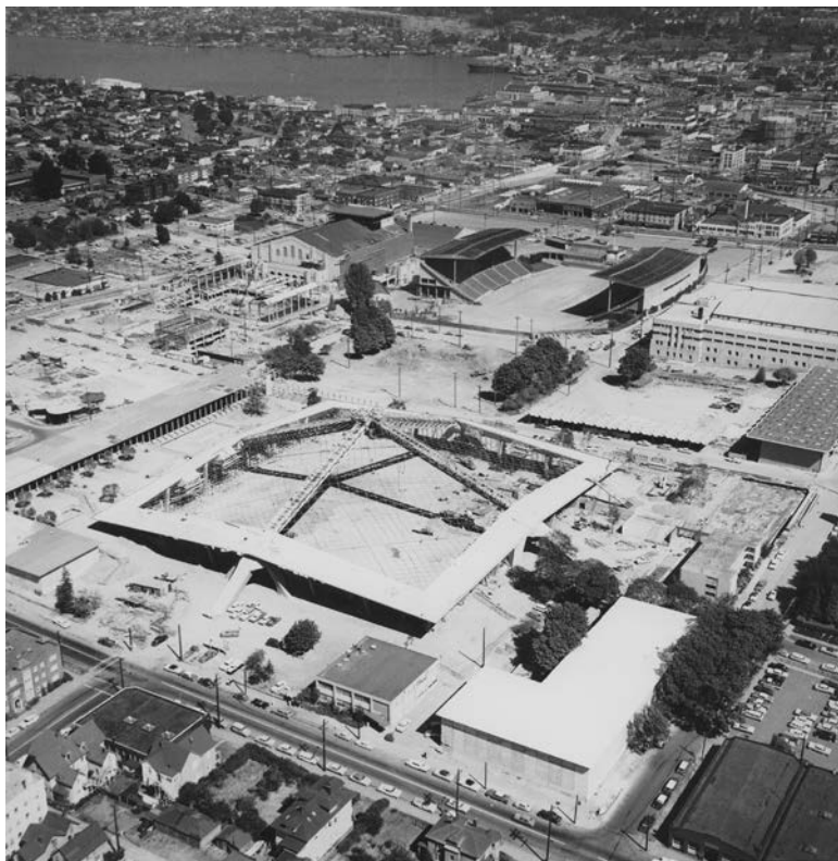
Photograph 2: Coliseum construction, November 1961. Courtesy Seattle Municipal Archives, #167458.
