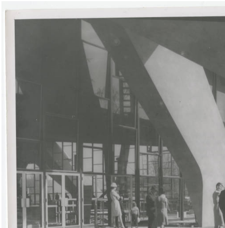
Photograph 10: View east along south elevation, 1962. Courtesy Seattle Public Library, Century 21 Exposition digital collection.
