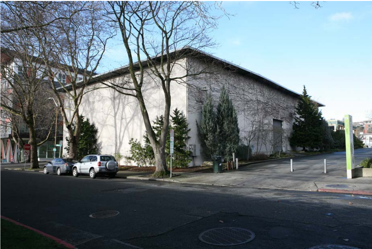
Photograph 29: 2017 view of the southeast corner of the NASA Building. Courtesy Artifacts Consulting, Inc.
