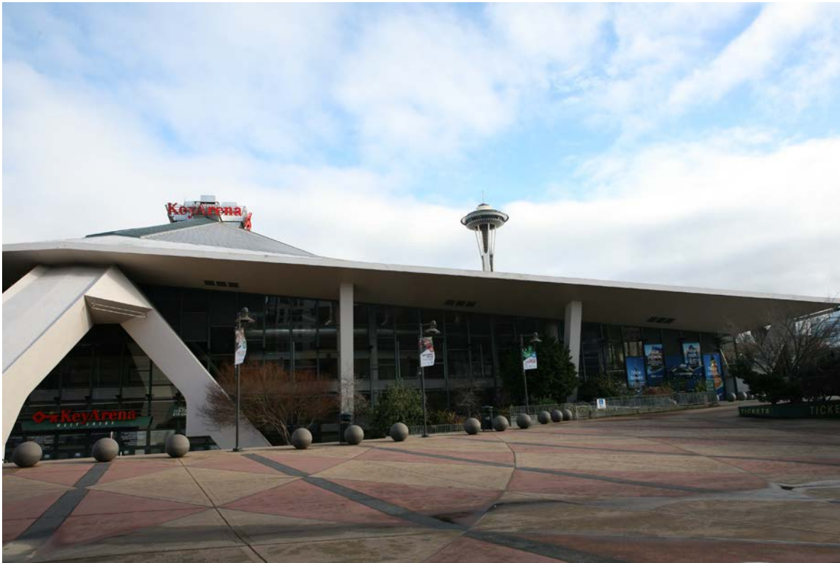
Photograph 23: 2017 view of southern end of KeyArena west elevation. Courtesy Artifacts Consulting, Inc.
