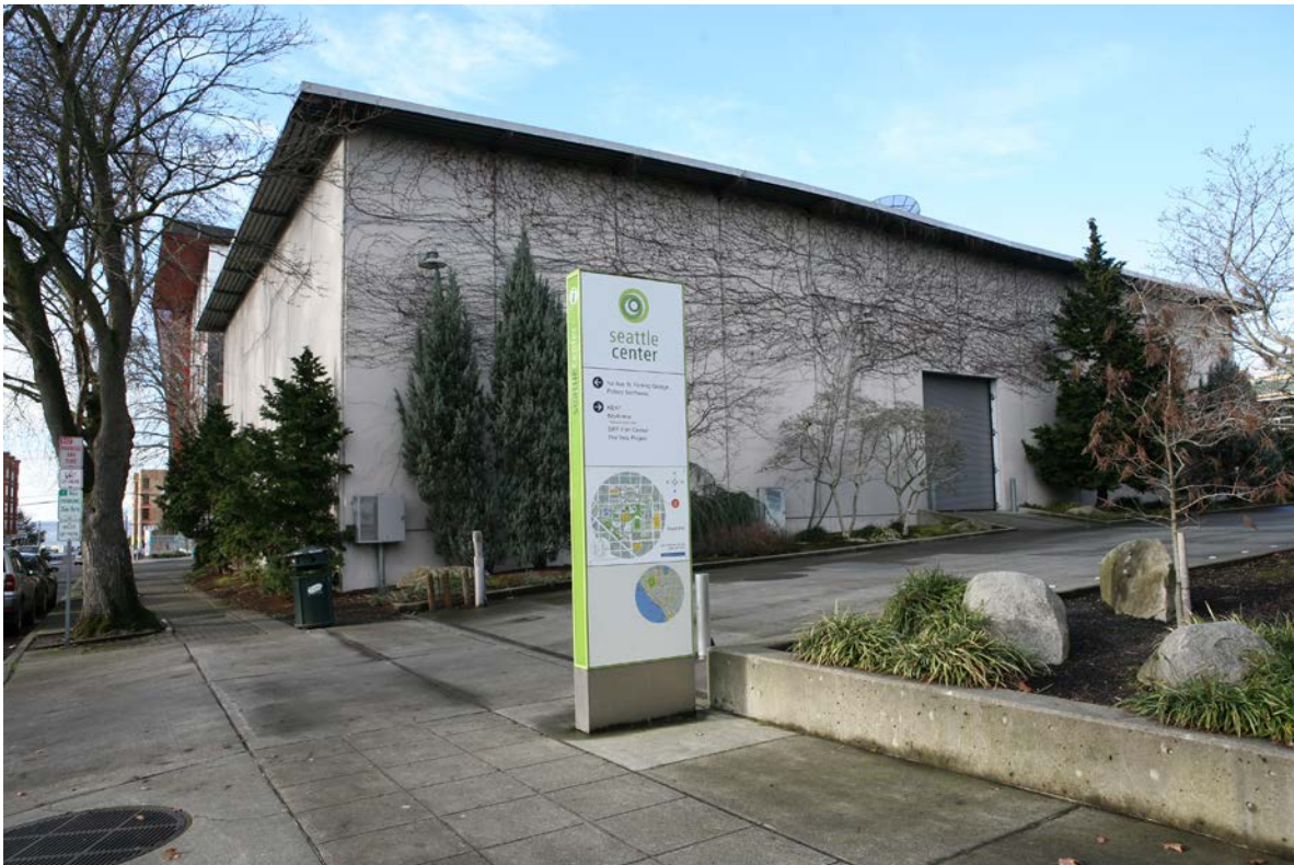
Photograph 28: 2017 view of the east elevation of the NASA Building. Courtesy Artifacts Consulting, Inc.
