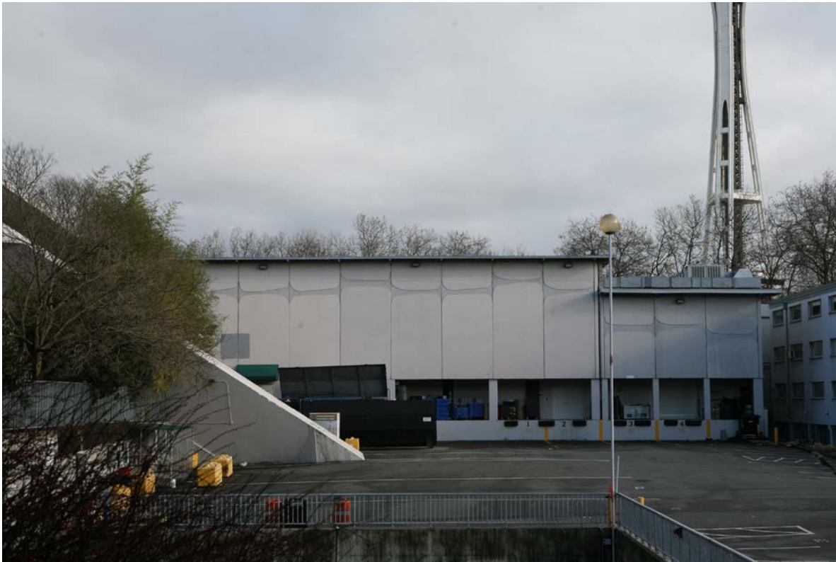
Photograph 43: 2017 view of the west elevation of the Seattle Center Pavilion. Courtesy Artifacts Consulting, Inc.
