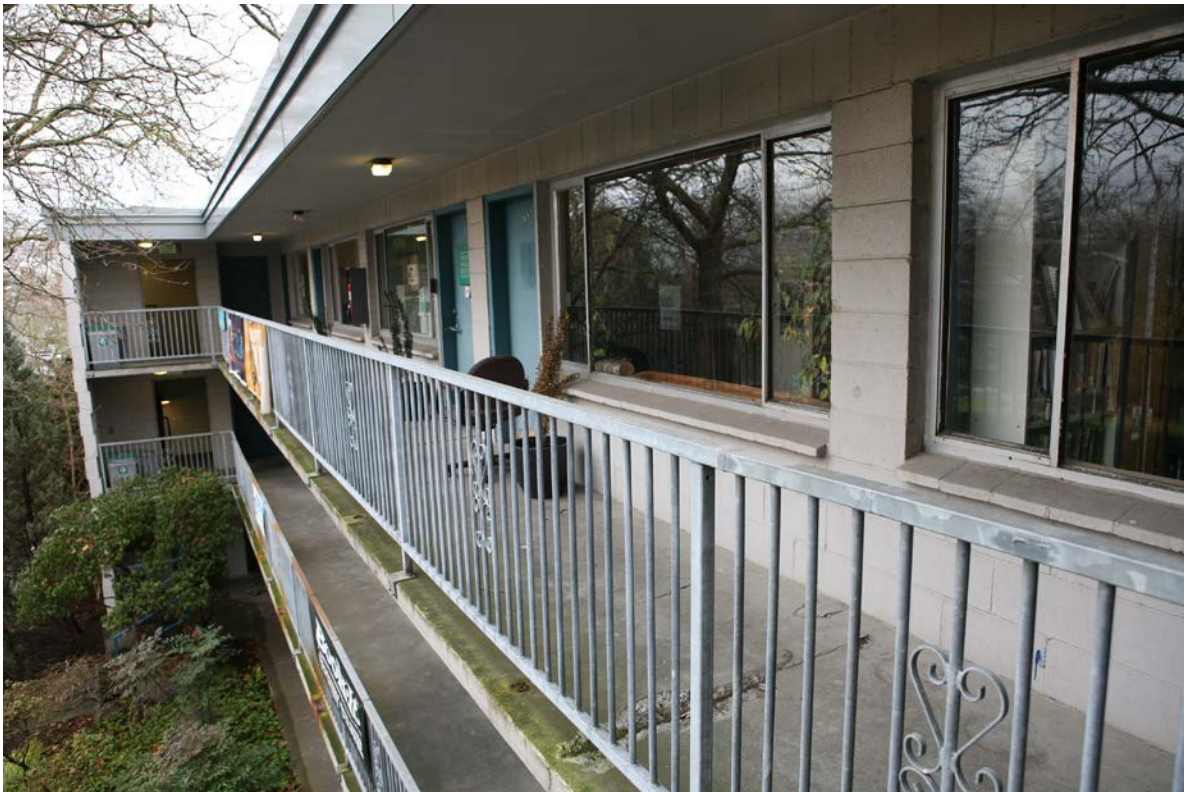
Photograph 38: View along 3rd floor balcony, looking west, Blue Spruce Building. Courtesy Artifacts Consulting, Inc.
