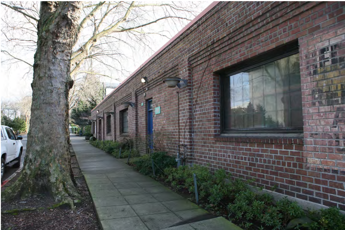
Photograph 8: 2017 view looking east along north elevation of Bressi Garage. Courtesy Artifacts Consulting, Inc.
