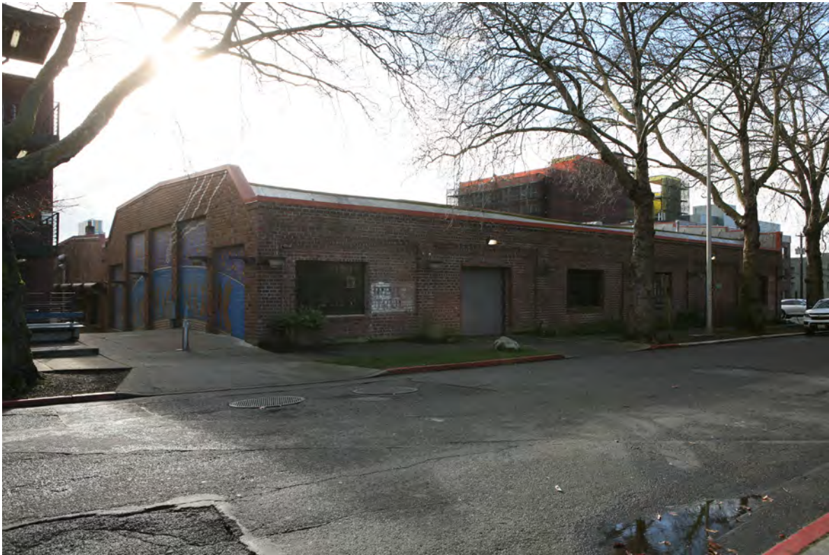
Photograph 3: 2017 view of Bressi Garage north and east elevations. Courtesy Artifacts Consulting, Inc.
