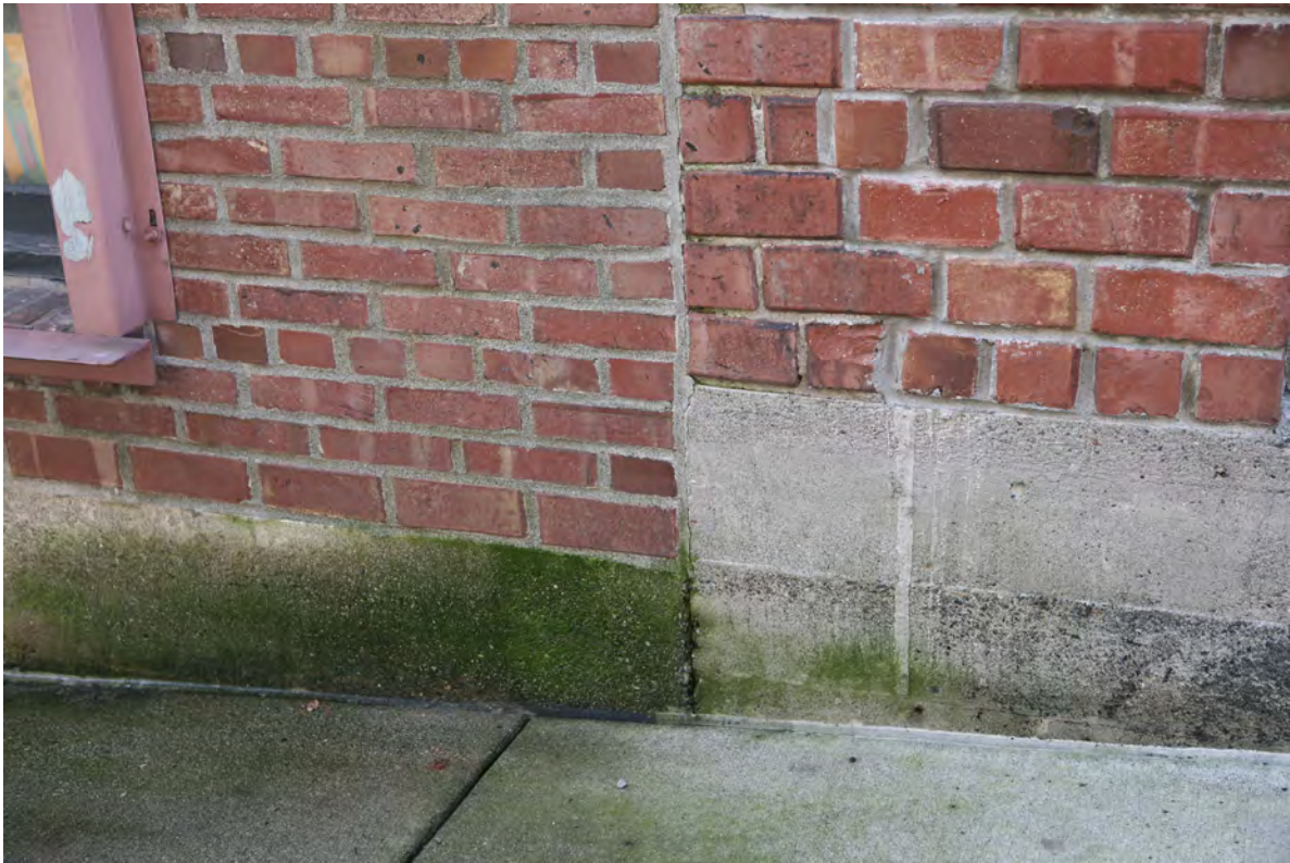
Photograph 7: 2017 detail view of foundation and structure on Bressi Garage east elevation. Courtesy Artifacts Consulting, Inc.
