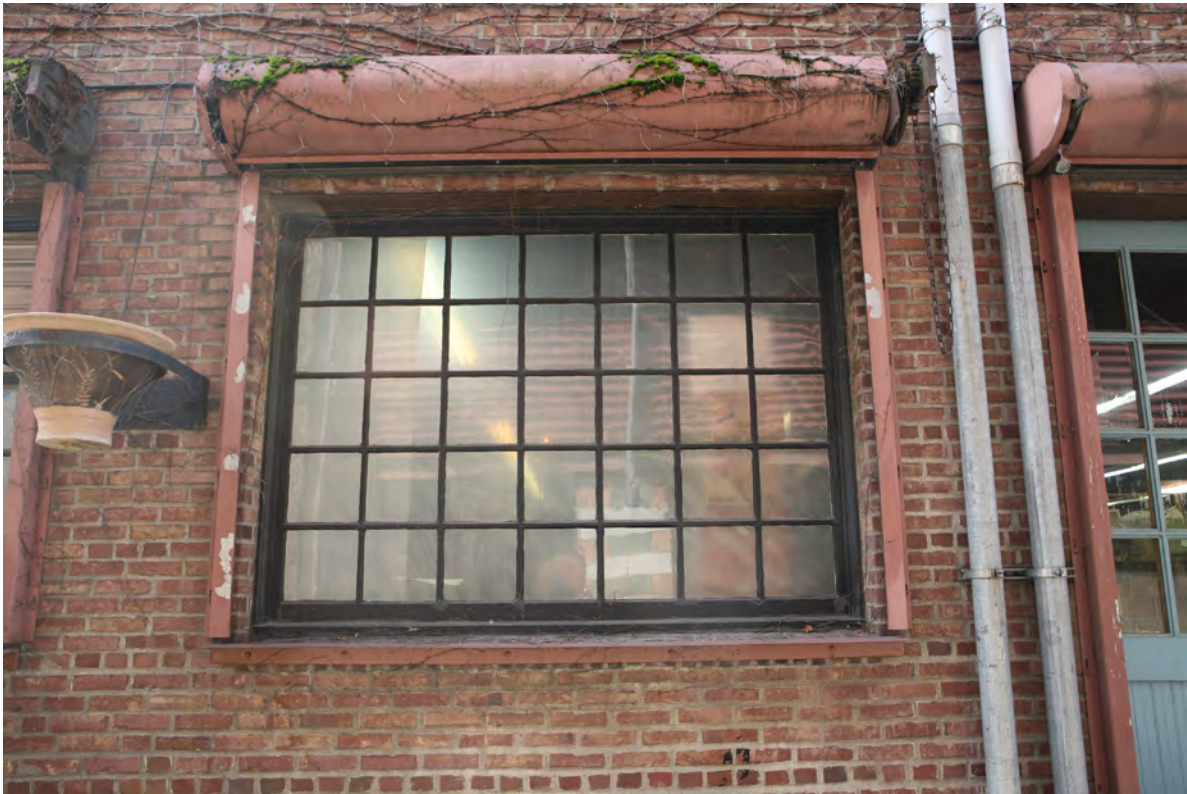
Photograph 15: 2017 view of extant original window on east elevation of the Bressi Garage. Courtesy Artifacts Consulting, Inc.
