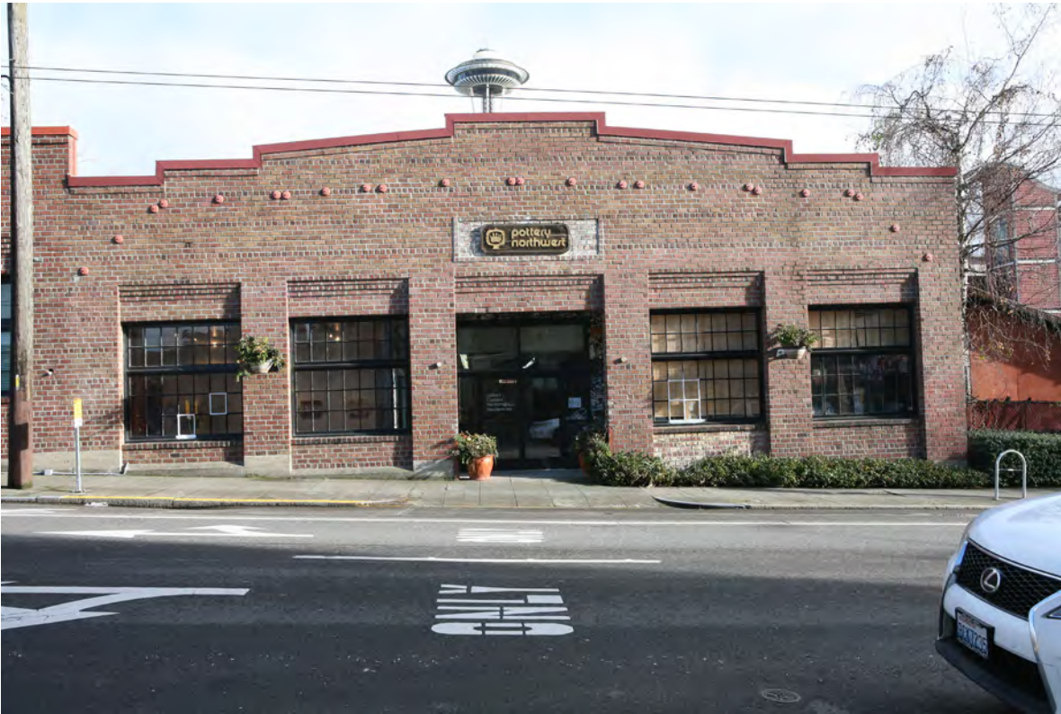
Photograph 11: 2017 view of Bressi Garage west elevation, south storefront. Courtesy Artifacts Consulting, Inc.
