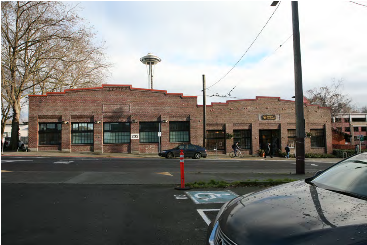
Photograph 1: 2017 view of Bressi Garage west elevation. Courtesy Artifacts Consulting, Inc.
