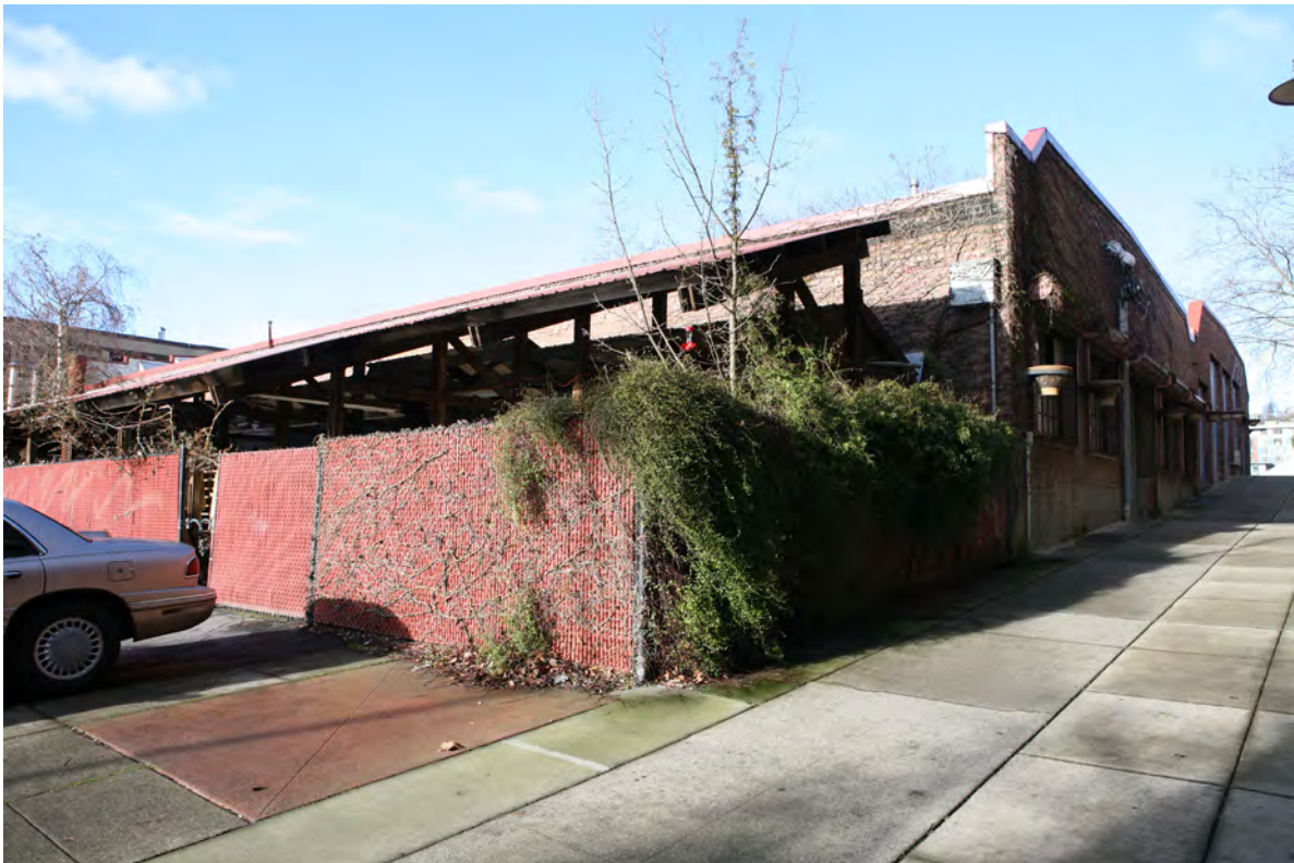
Photograph 4: 2017 view of Bressi Garage south and east elevations. Courtesy Artifacts Consulting, Inc.
