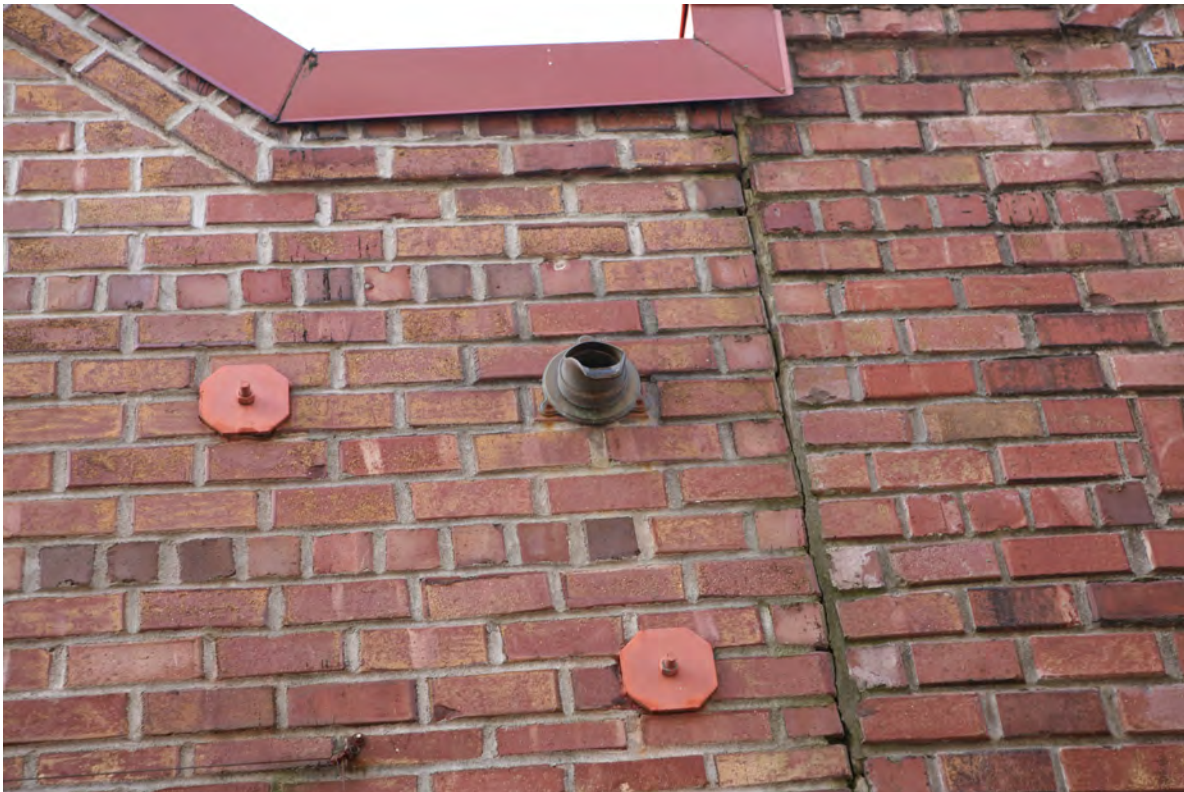
Photograph 6: 2017 detail view of Bressi Garage brick and parapet on east elevation. Courtesy Artifacts Consulting, Inc.
