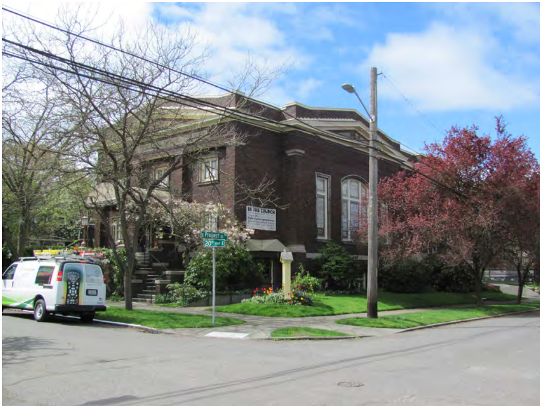
Photograph 30: An example of Heinemann's work, Prospect Congregational Church (1924) at 1919 E Prospect Street. Courtesy Artifacts Consulting, Inc.
