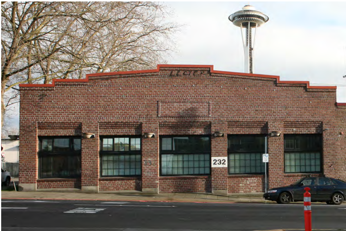
Photograph 13: 2017 view of Bressi Garage west elevation, north storefront. Courtesy Artifacts Consulting, Inc.
