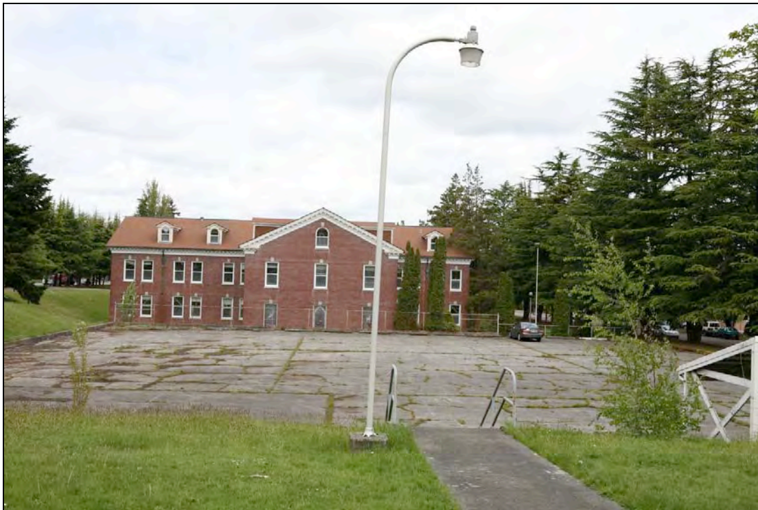
Figure 72: 2009, light fixture next to the parking lot at the southern end of Building 9 (Site ID Number 41). Photo by Artifacts Consulting, Inc.
