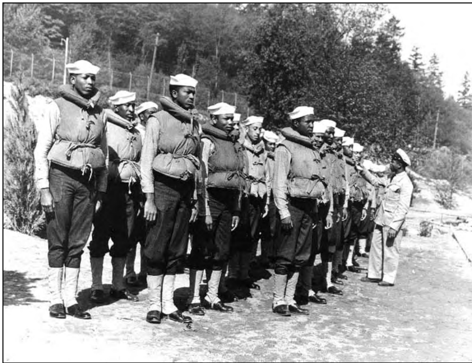
Figure 29: 1944, a photo depicting Steward's Mates trainees preparing for boat drills at Naval Air Station, Seattle. Photo by U.S. Navy. Source: National Archives, Image No. 80-G-233286.
