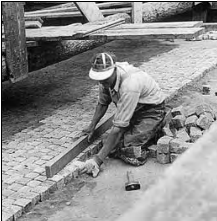
Figure 20: 1930, photo depicting the laying of granite blocks as part of the construction of the runway, shop and storehouse at Naval Air Station, Seattle. Photo by U.S. Navy. Source: HistoryLink.org, Essay No. 2249.
