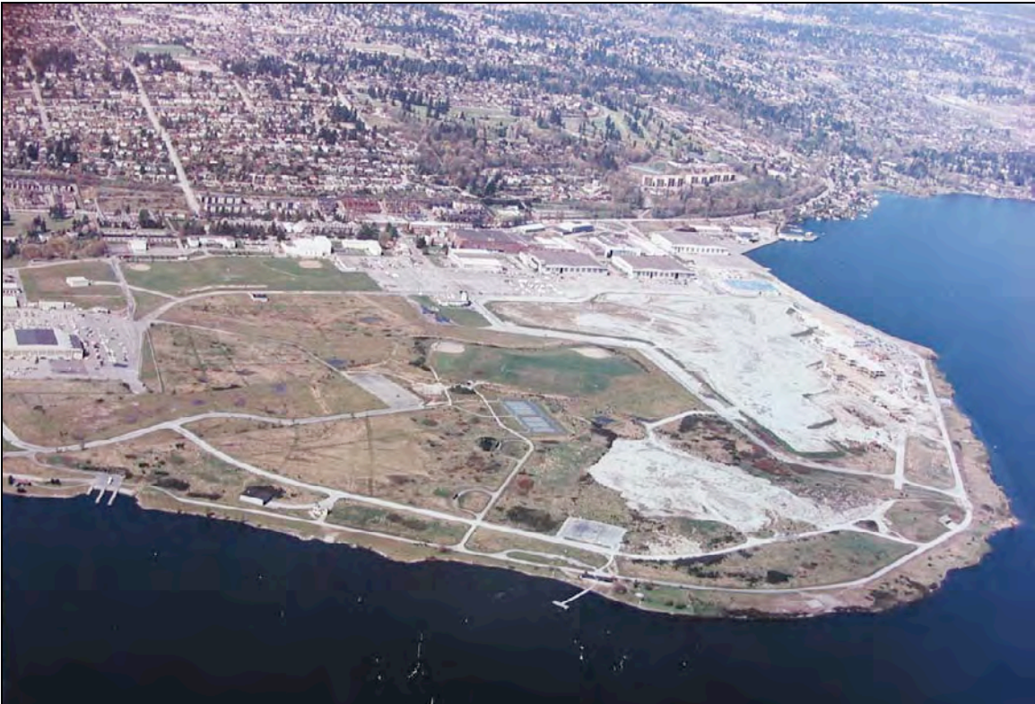
Figure 41: 1981-82, aerial view showing the construction of the National Oceanic and Atmospheric Administration facilities. Source: Seattle Parks and Recreation.
