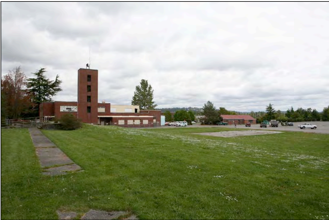
Figure 86: 2009, looking north at the lawn between Buildings 18 and 47 (Site ID Numbers 10 and 11). Photo by Artifacts Consulting, Inc.
