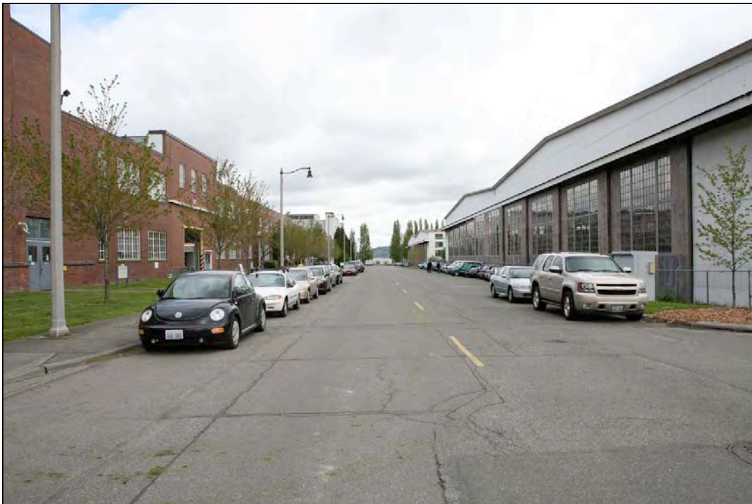
Figure 69: 2010, a photo looking north on 63 rd Avenue NE, between Buildings 5 and 33 (Site ID Numbers 51 and 2). Photo by Lynn Ferguson.
