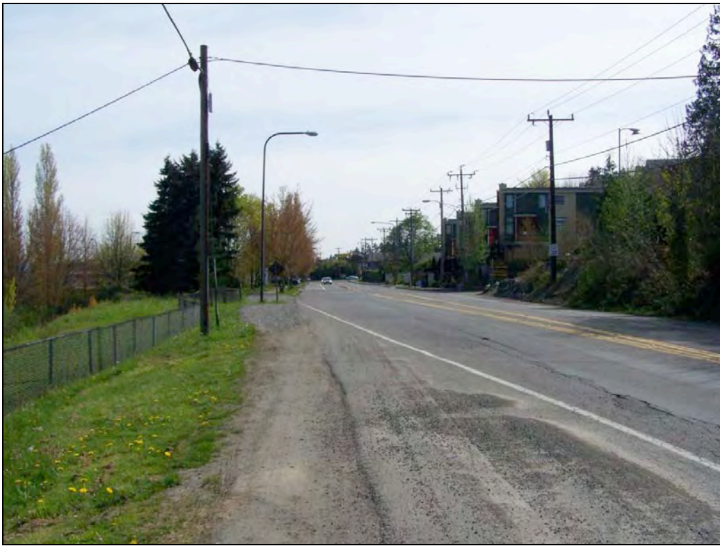
Figure 58: 2010, a photo looking south on Sand Point Way NE, towards the northern end of the proposed district. Photo by Lynn Ferguson.
