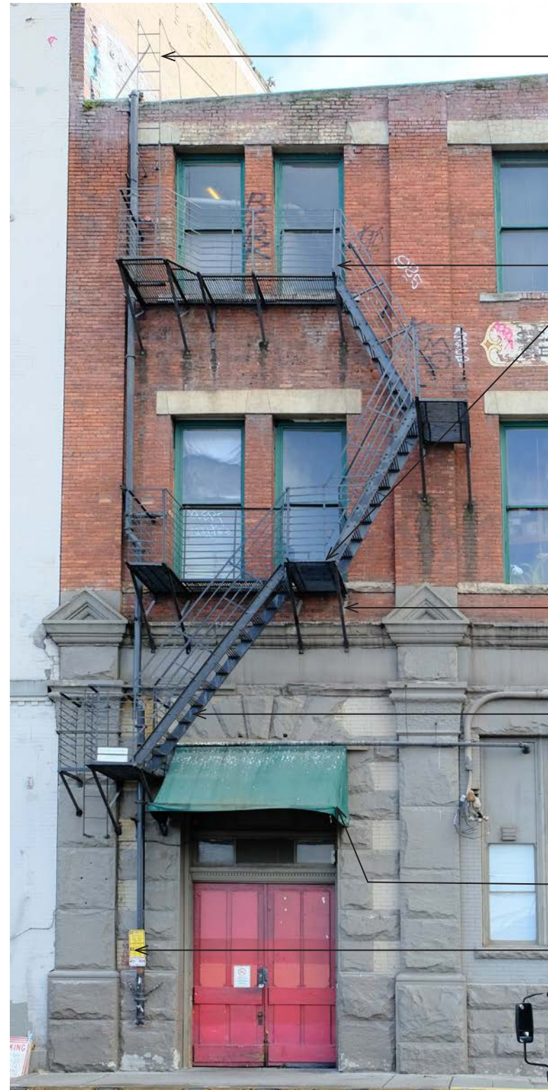
EXISTING FIRE ESCAPE AT WEST ELEVATION
