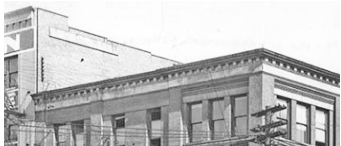
HISTORIC CONDITION OF WEST BRICK PARAPET
