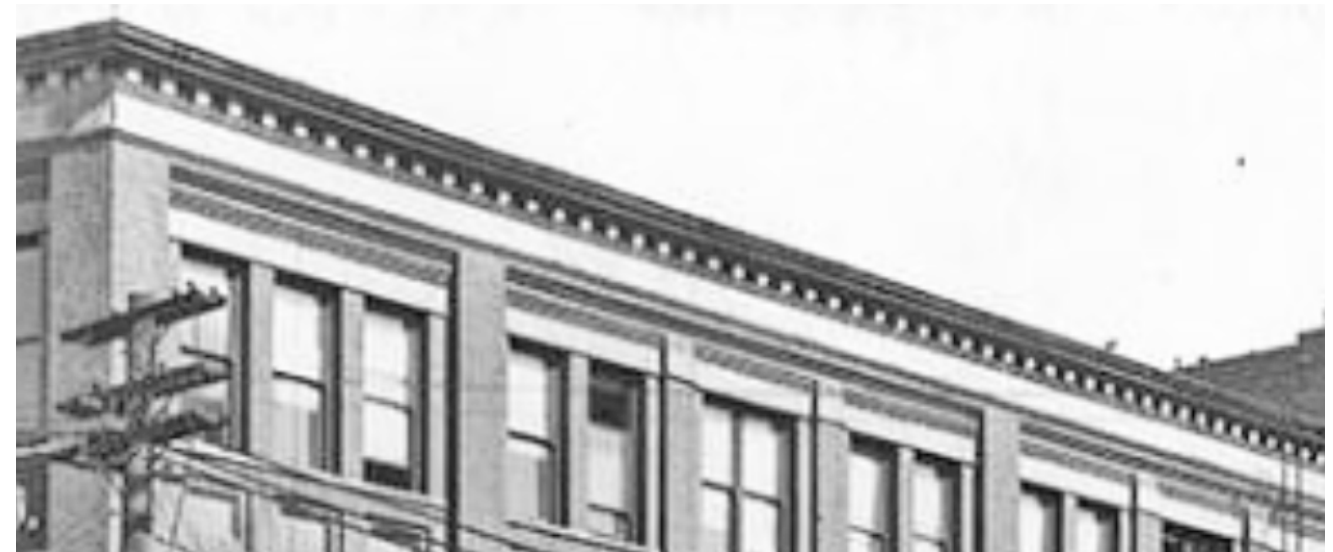
HISTORIC CONDITION OF SOUTH BRICK PARAPET AND CORNICE
