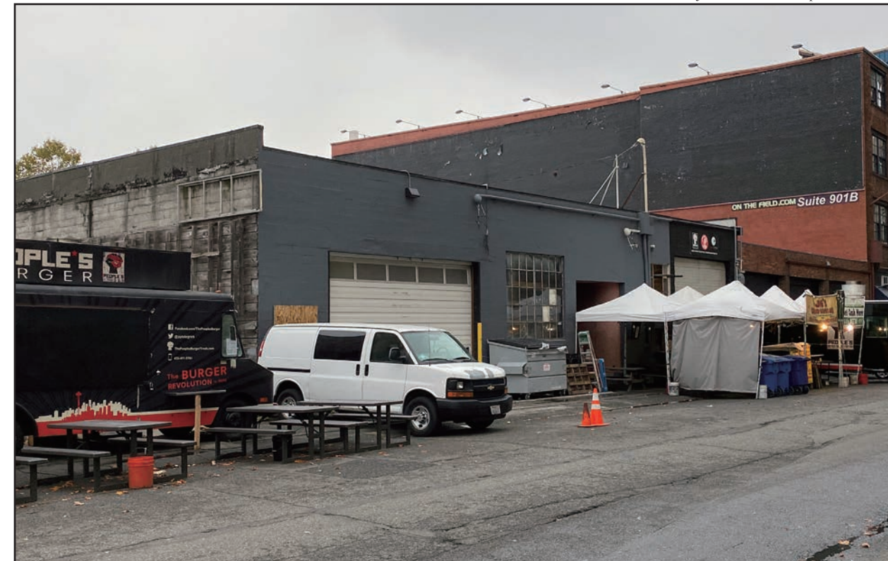
Figure 15 • 904 First Avenue S, eastern façade
