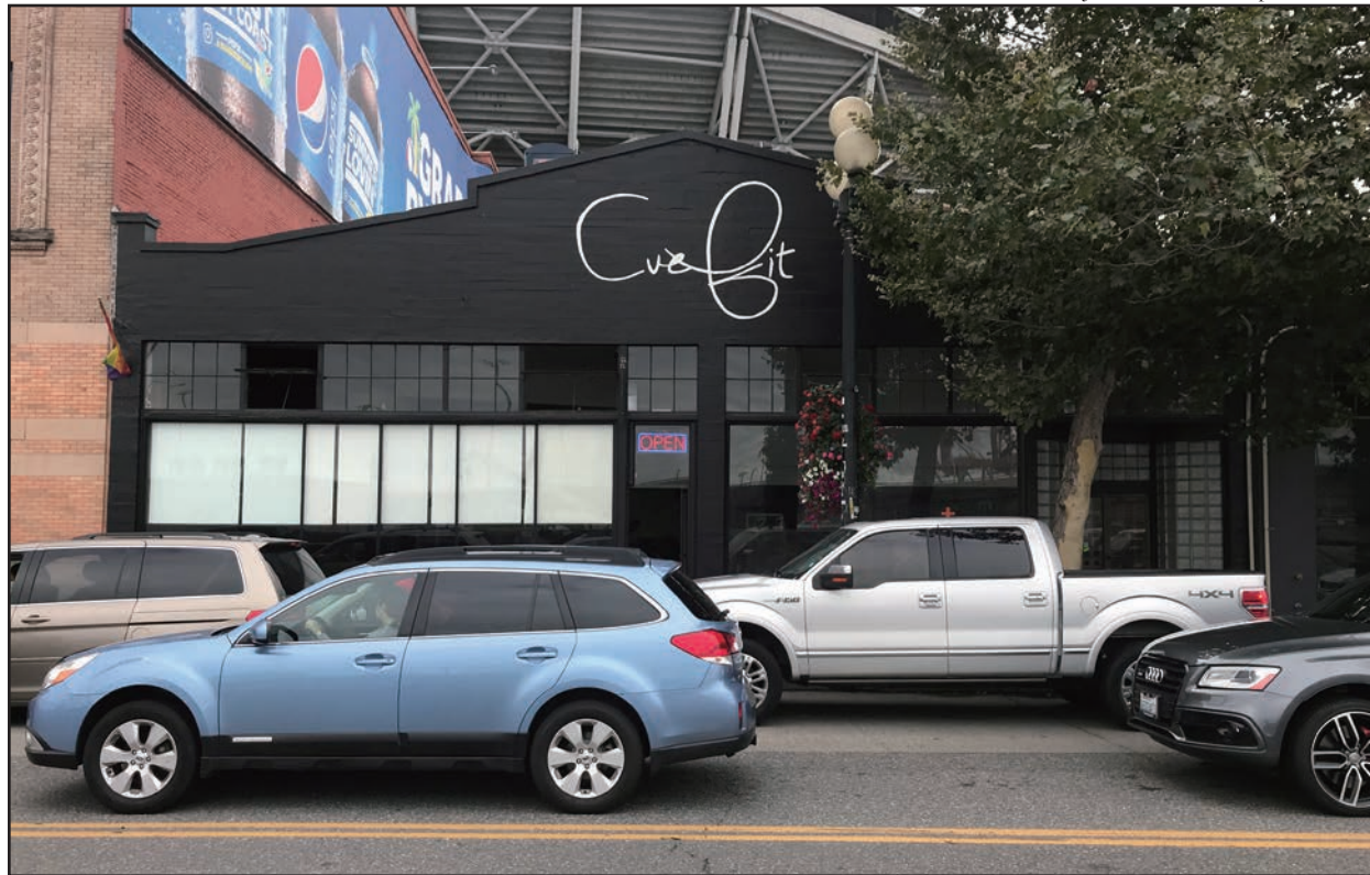
Figure 9 • 902 First Avenue S, western façade
