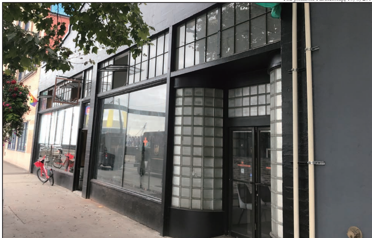
Figure 10 • 902 First Avenue S, western façade
