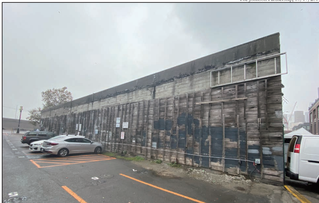
Figure 14 • 904 First Avenue S, southern façade
