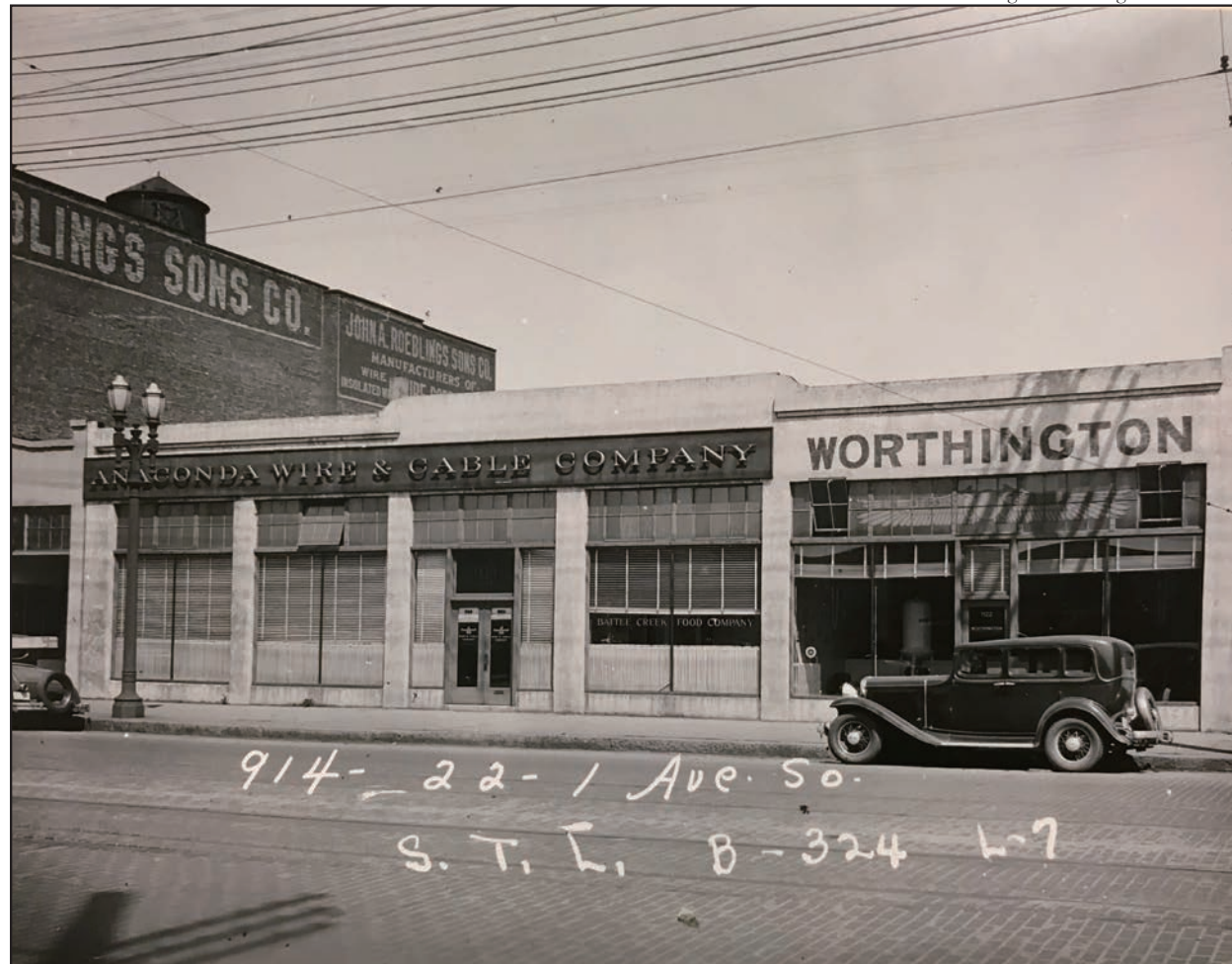
Figure 35 • 904 First Avenue S (formerly 914 First Avenue S), Tax Assessor photo, 1937
