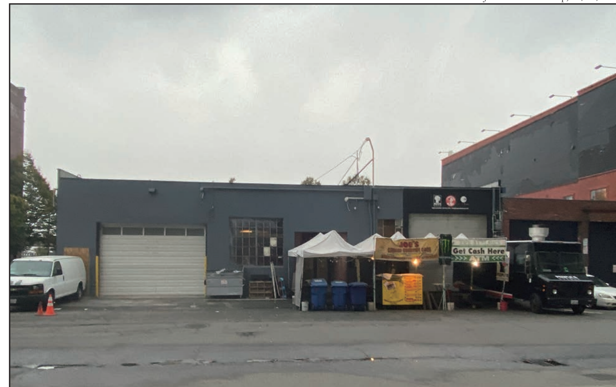
Figure 16 • 904 First Avenue S, eastern façade
