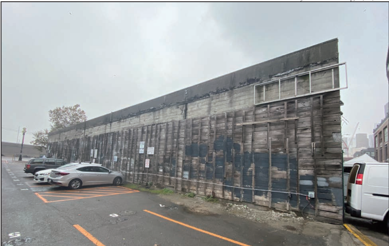
Figure 14 • 904 First Avenue S, southern façade
