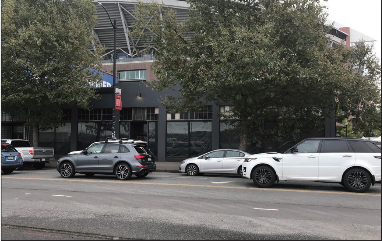
Figure 13 • 904 First Avenue S, western façade
