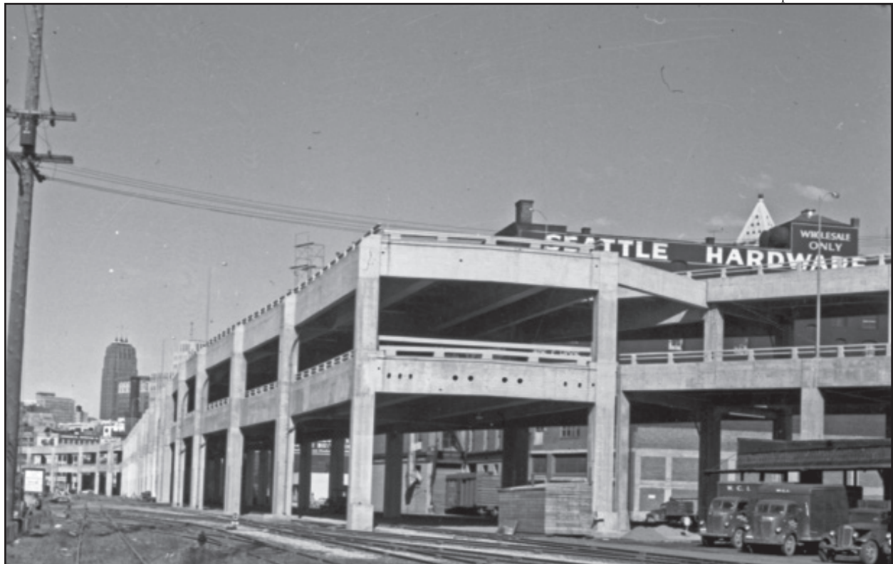
Figure 28 • Alaskan Way Viaduct, 1953
