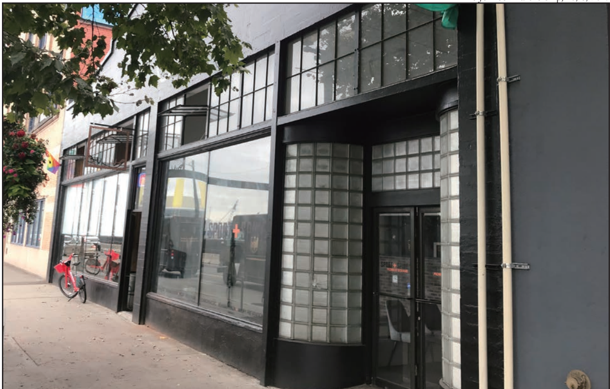
Figure 10 • 902 First Avenue S, western façade
