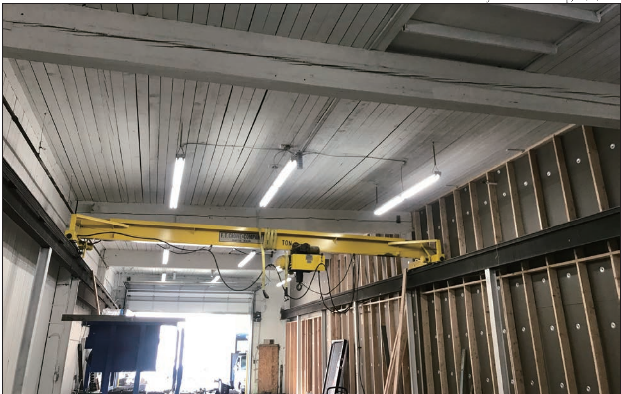
Figure 18 • 904 First Avenue S, southernmost tenant space interior
