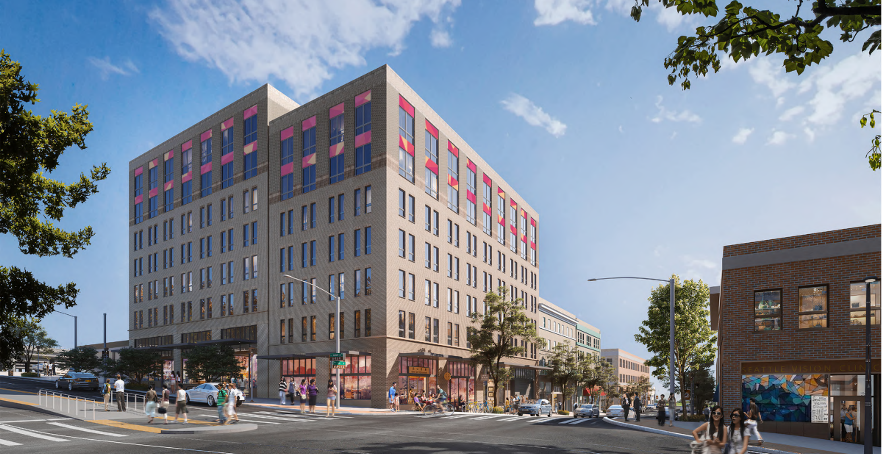
VIEW OF NORTHWEST CORNER WITH ARTWORK ON UPPER LEVEL SPANDRELS
