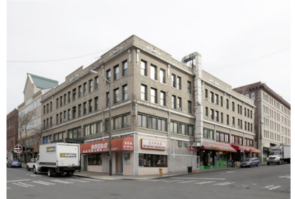
A / ATLAS APARTMENTS: 420 MAYNARD AVENUE S
