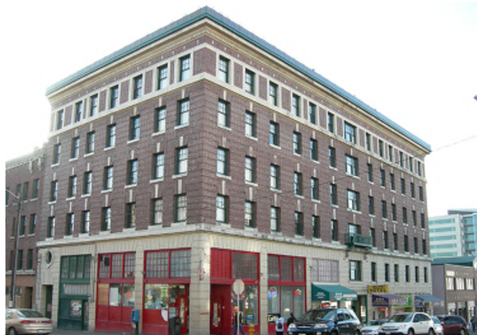
G/ ALPS APARTMENTS: 621 S KING STREET
