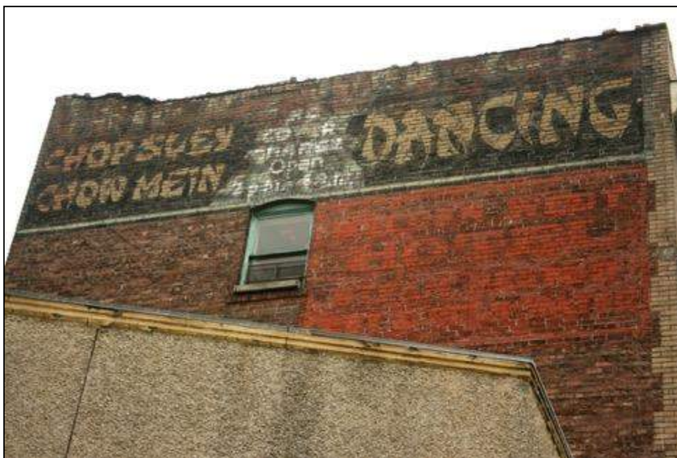
Below, a 2008 photo of painted signage on the upper north façade of the Republic Hotel, showing and the condition of the masonry and parapet. The stucco clad walls in the foreground are part of the subject garage.
