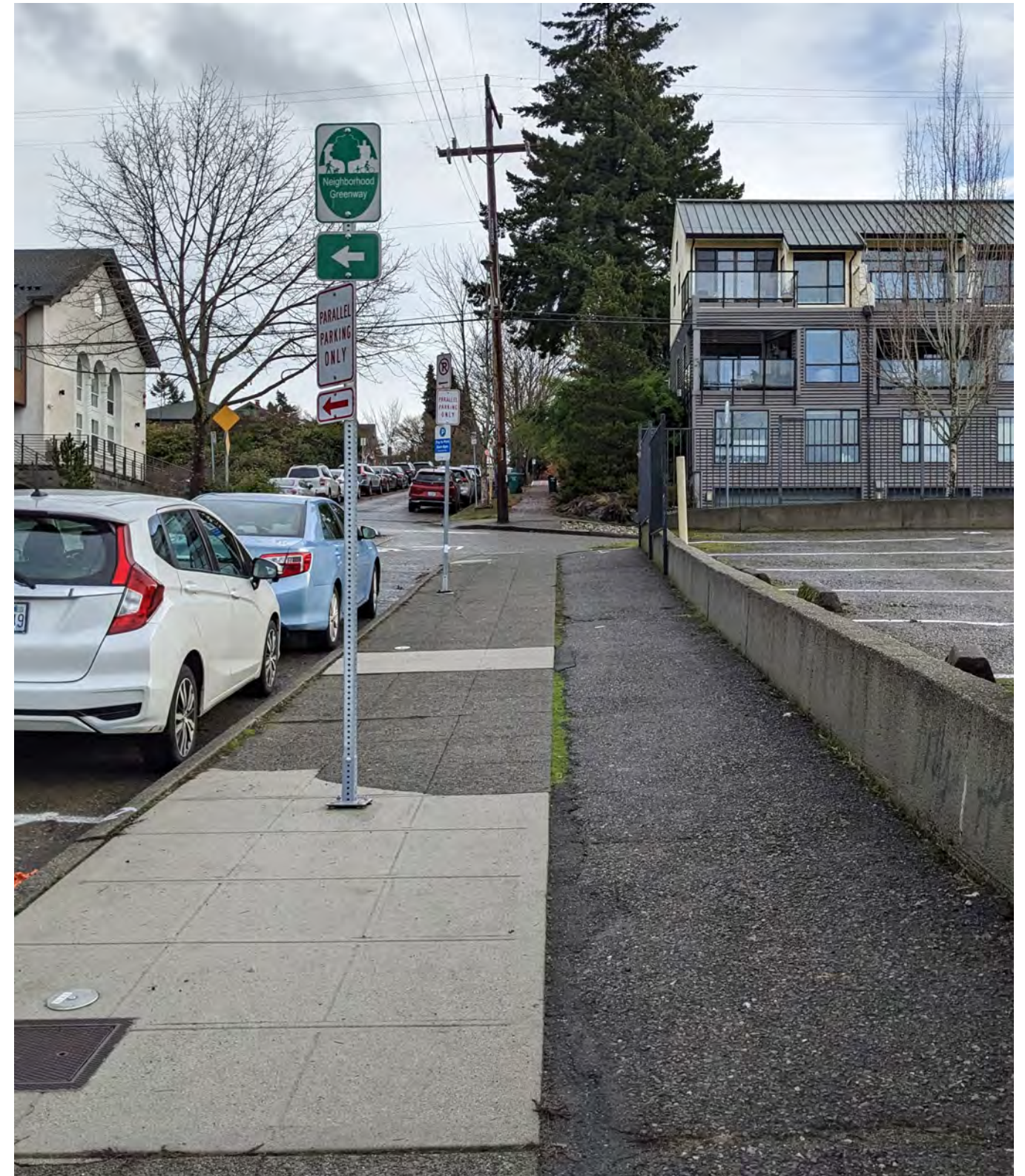
EXISTING SIDEWALK EAST OF POWER POLE, LOOKING EAST
