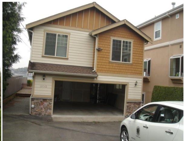
Back of house with garage
