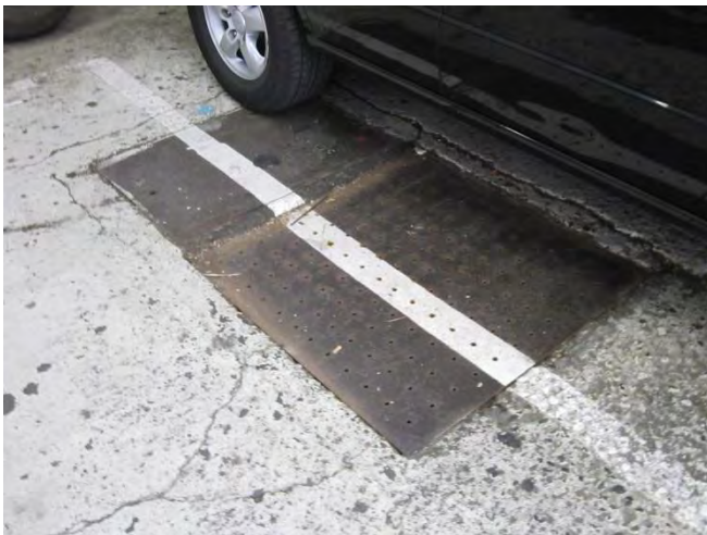
Photograph 3. Oil-water separator located within the eastern portion of the on-Property building.
