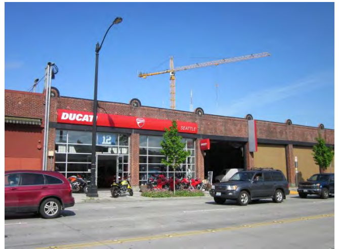
Photograph 8. Ducati showroom on the northwest-adjointing property.
