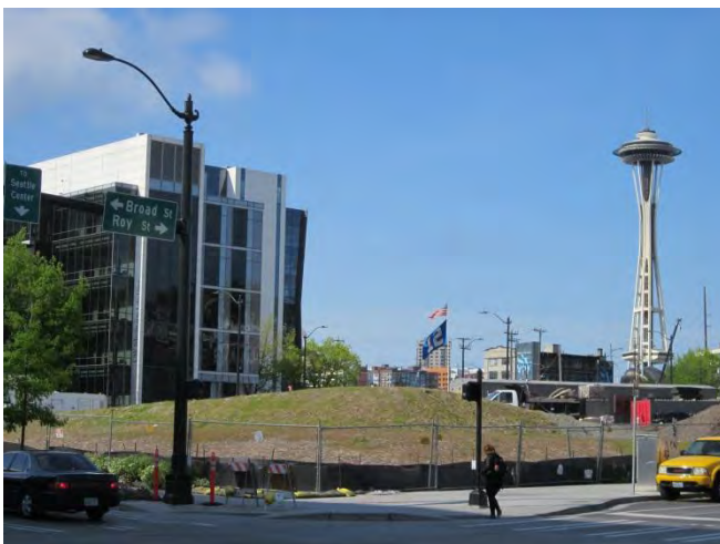
Photograph 11. Cleared and graded land on the southwest-adjointing property.
