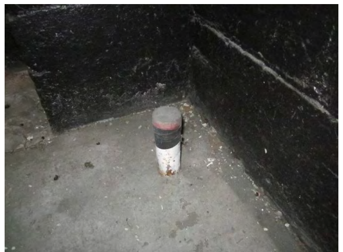
Photograph 6. Unidentified one-inch pipe with rubber cap located on the northwestern portion of the Property.
