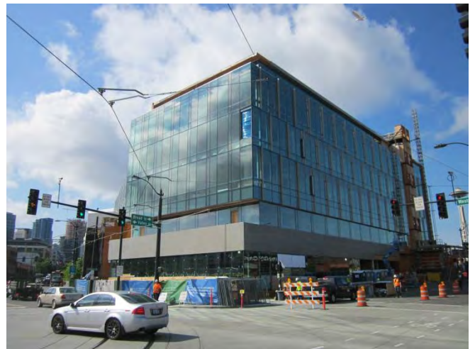
Photograph 10. Office building under construction on the south-adjointing property.
