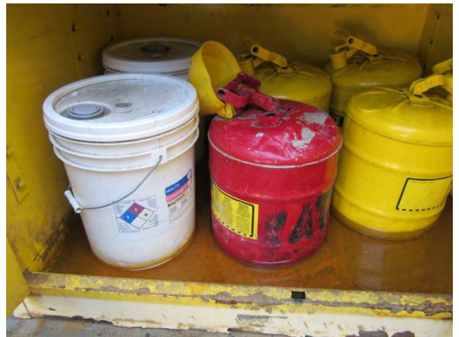
Photograph 4. Gasoline and diesel containers stored in a flammable materials cabinet on the Property.
