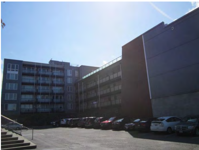
Photograph 9. Apartment building on the north-adjointing property.
