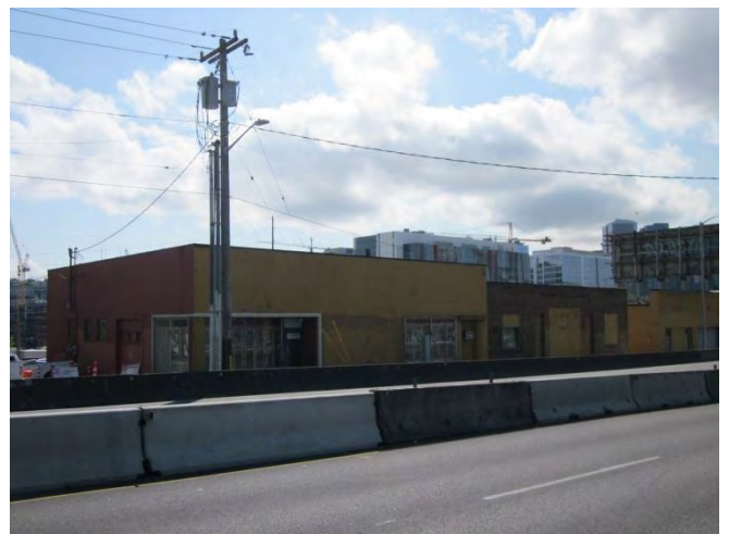
Photograph 12. Warehouse on the southeast-adjointing property.
