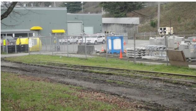
View of PMA No. 139, City owned property at the north end of the Subject Property.
