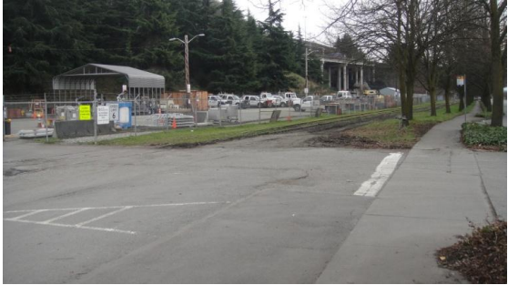
North end of PMA No. 1477 at the entrance to PMA No. 139 (Sunny Jim) off Airport Way South. The railroad tracks end at the pavement.
