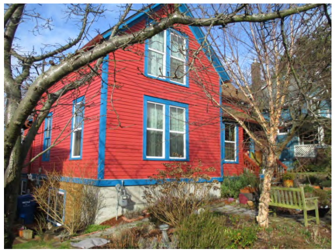
Photograph 2. North-adjointing single family residence. Photo facing west.
