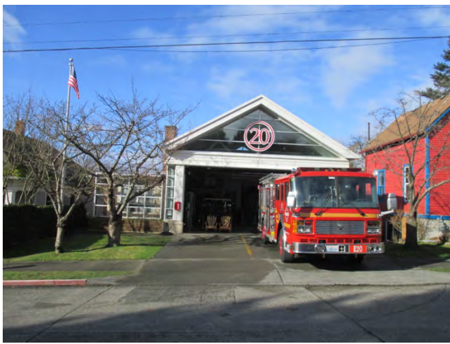
Photograph 1. Fire Station 20. Photo facing west.
