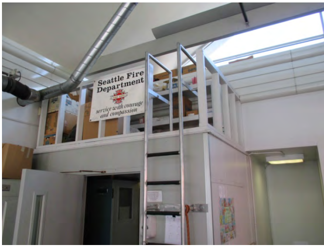
Photograph 13. Loft located in southwest corner of garage.
