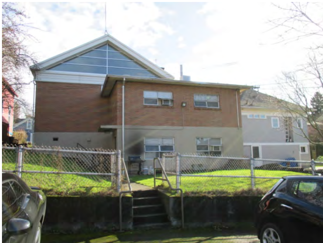
Photograph 17. View of Fire Station #20, seen facing east.
