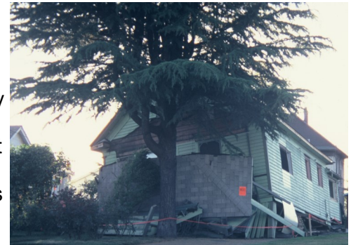
Damage to home that has not been retrofitted
