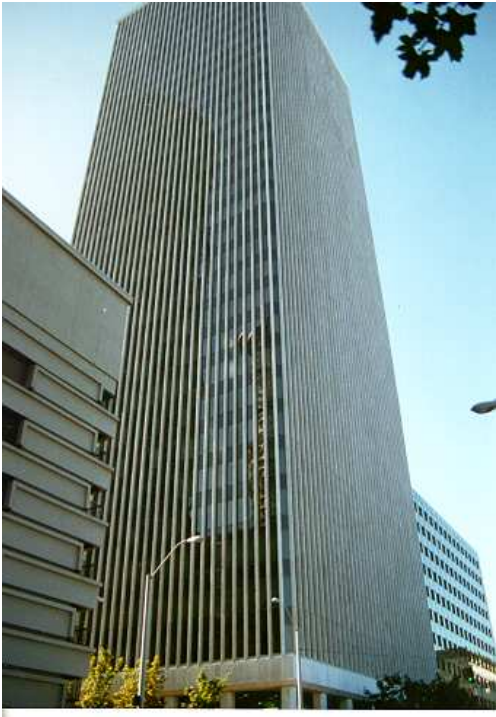
Figure 8: The Westin Building in downtown Seattle sits atop the juncture of several fiber-optic trunk cables.
