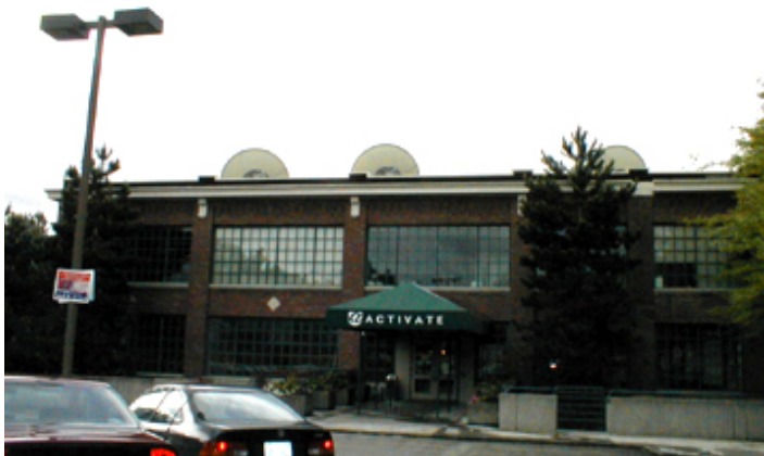
Figure 7: By locating outside the downtown core along Rainier Avenue, Activate.net protected its rooftop satellite dishes from high-rise shadows and interference.
