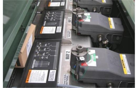
**Automated Switch Controls and Fiber Optic Transceiver**
