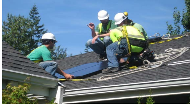
Photo Credit: Puget Sound Solar
