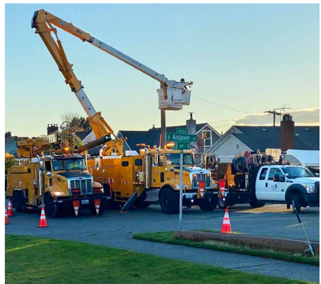
Pole replacement in South Seattle
