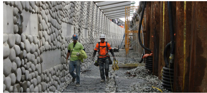
Marine mattresses help create shallow water habitat near seawall
