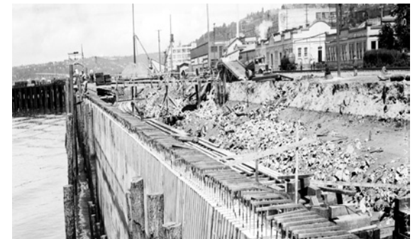
Seawall being constructed in 1934.. Photo Credit: Seattle Municipal Archives Photograph Collection.
