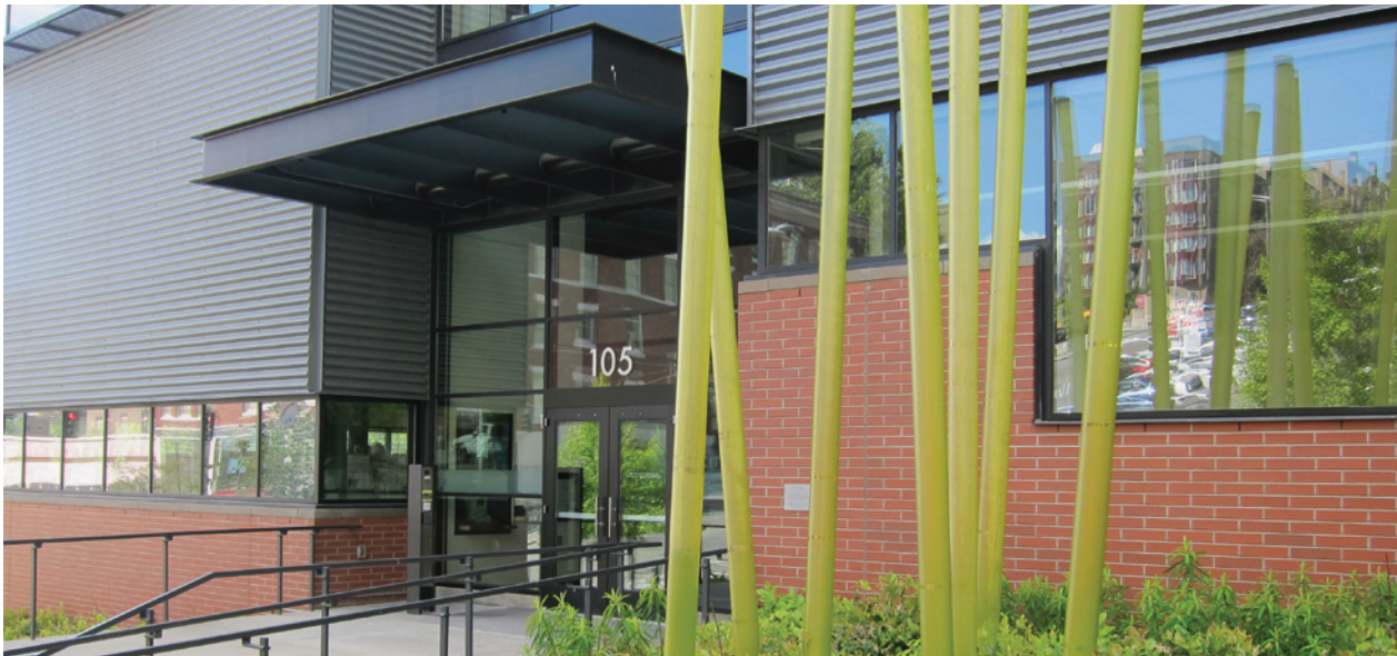
City of Seattle Emergency Operations Center. Photo: City of Seattle.
