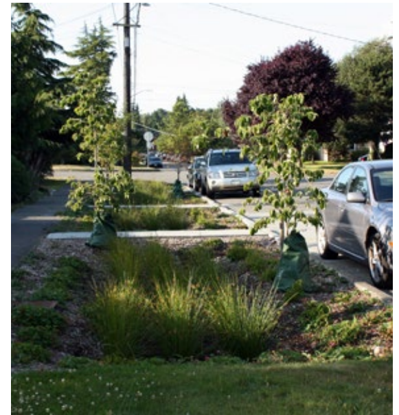
Ballard rain garden
