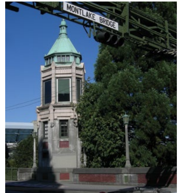
Montlake bridge, south tower
