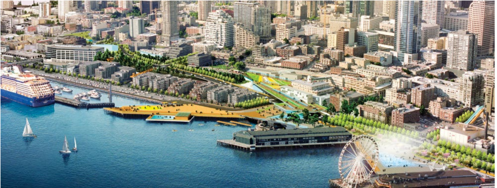
Design of post-tunnel waterfront
