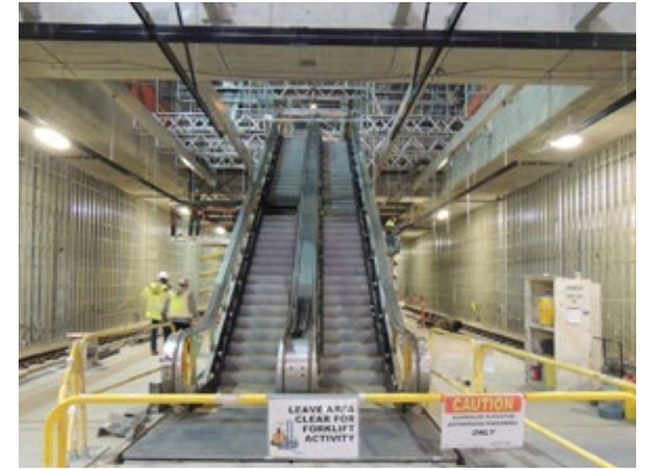
Light rail tunnel hole, left. Preview of light rail tunnel, above.
