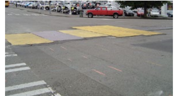
Steel plates on Seattle streets
