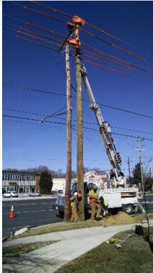
Figure 22: OSP Crew Replacing a Pole
