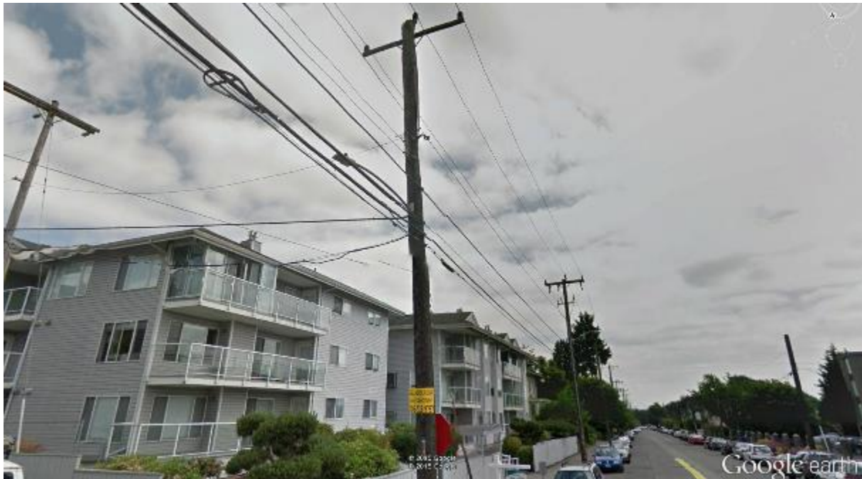
Figure 20: Example of a Pole in Seattle with Congested Communications Space (Google Earth)
