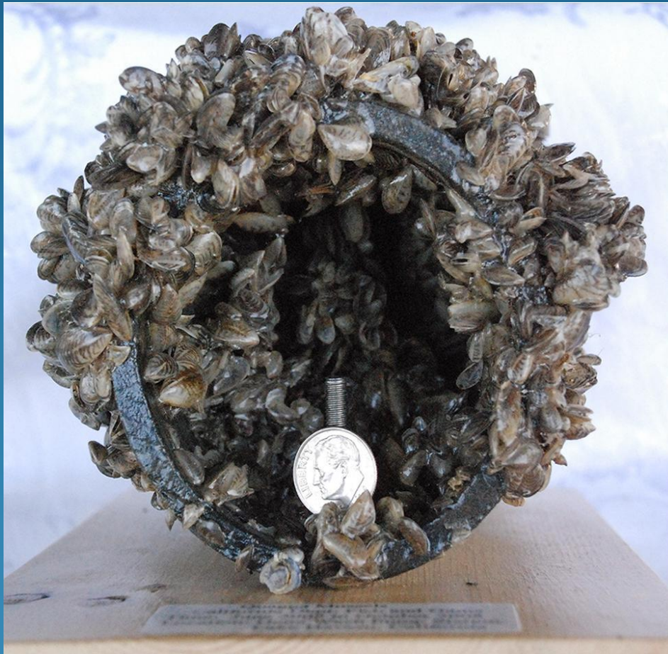
Pipe clogged with mussels
