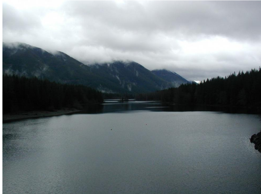
Masonry Pool Reservoir taken on March 21, 2010
