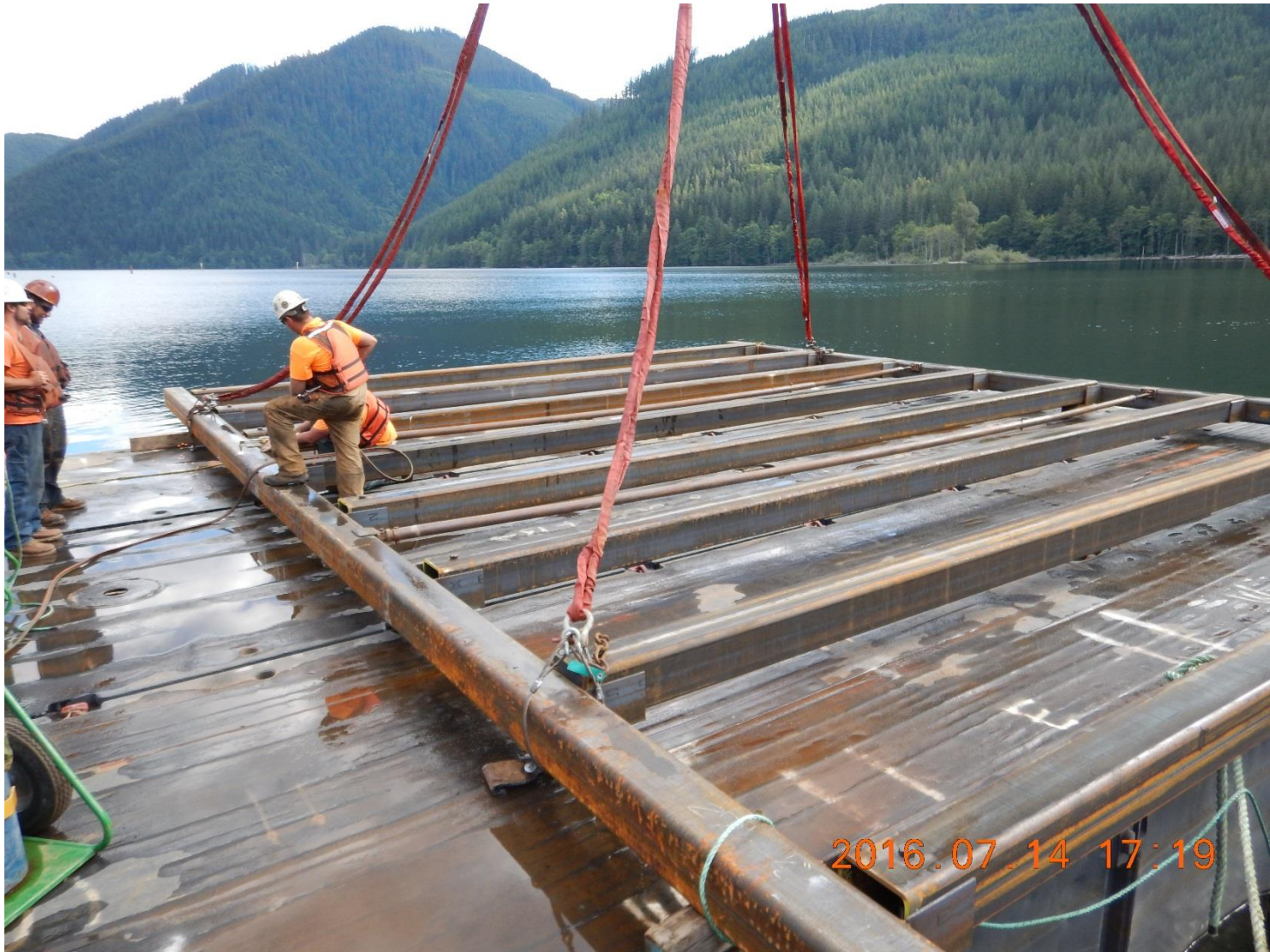
Morse Lake Pump Plant
