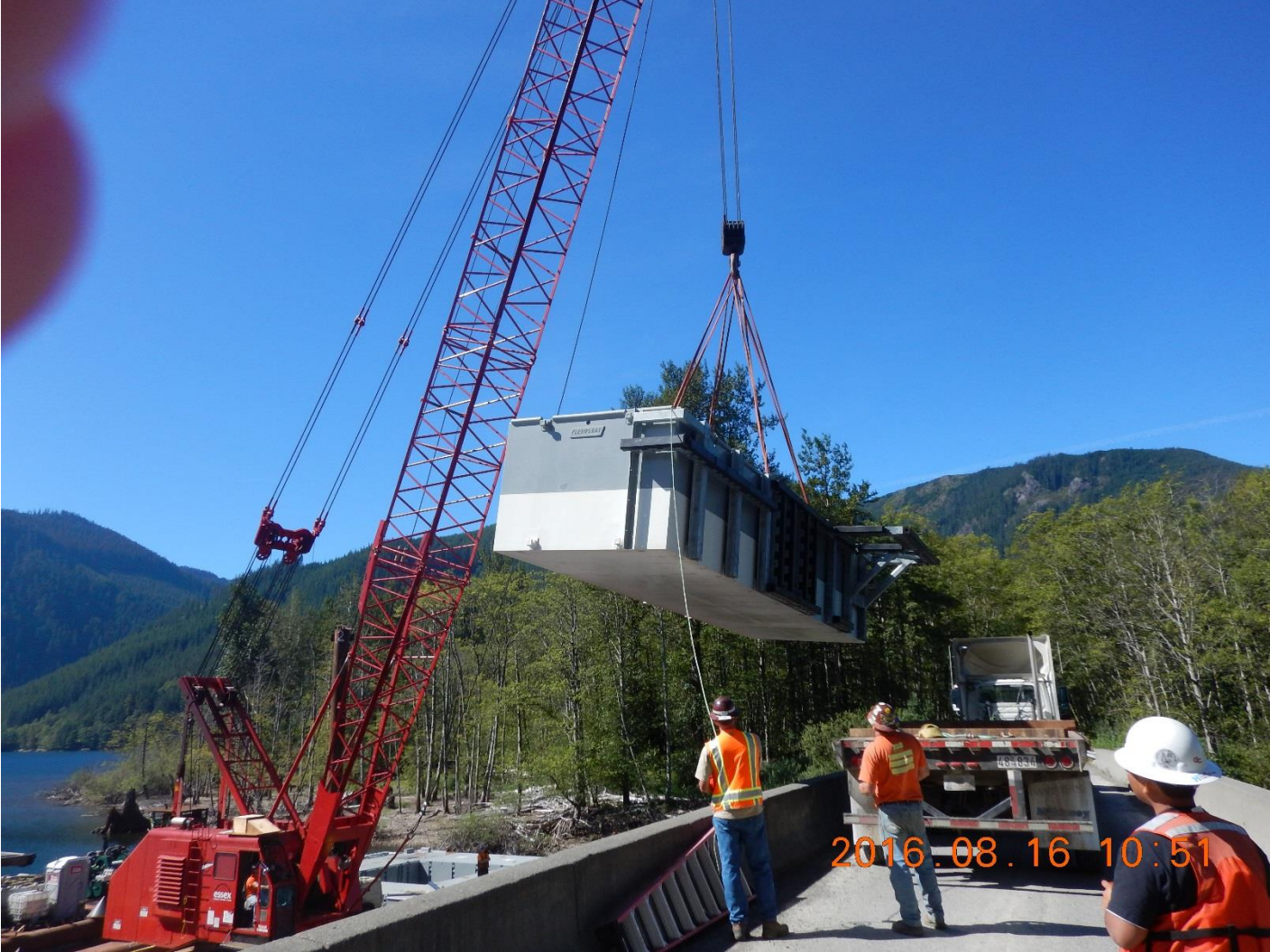
Morse Lake Pump Plant
