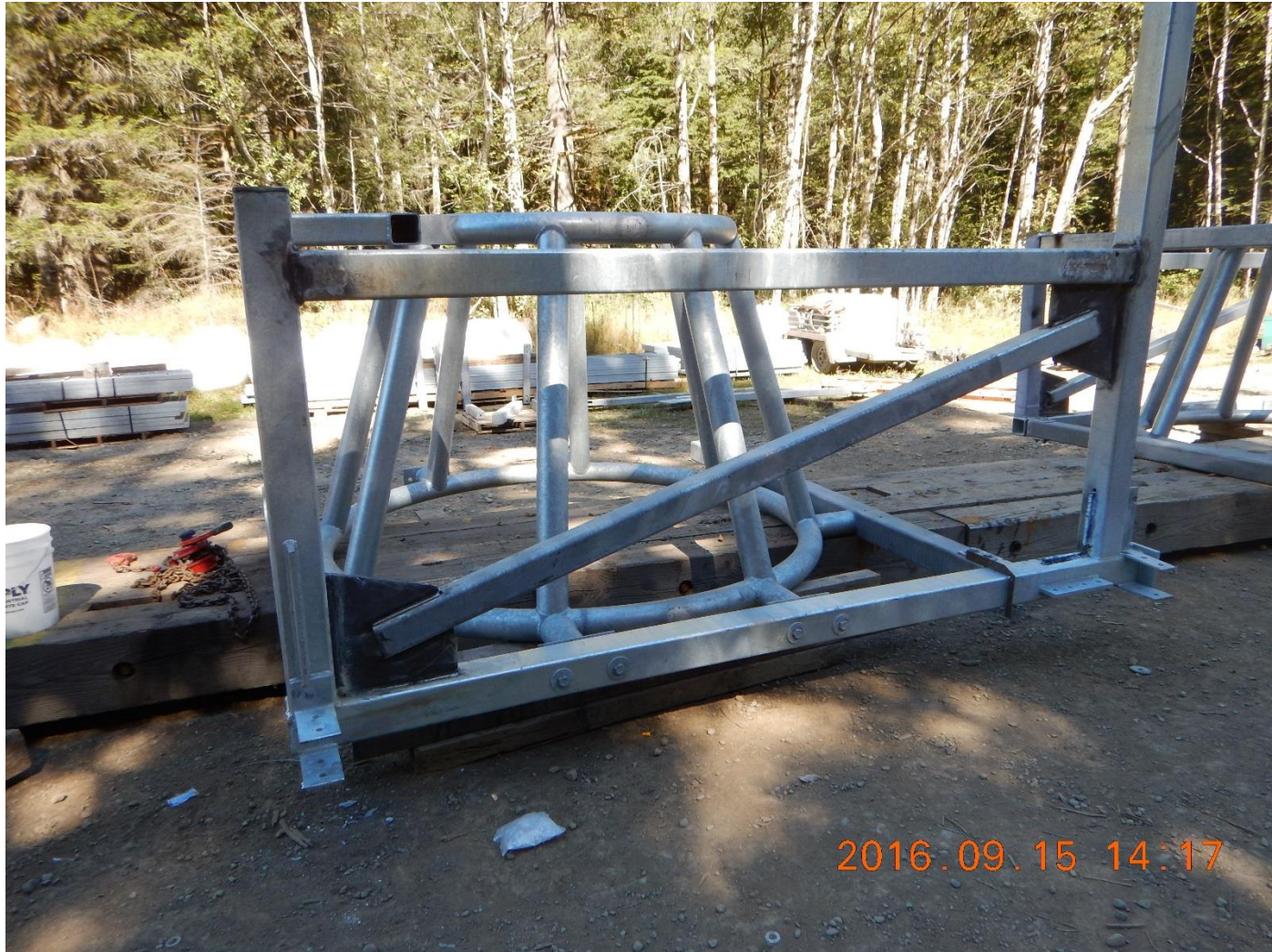
Morse Lake Pump Plant
