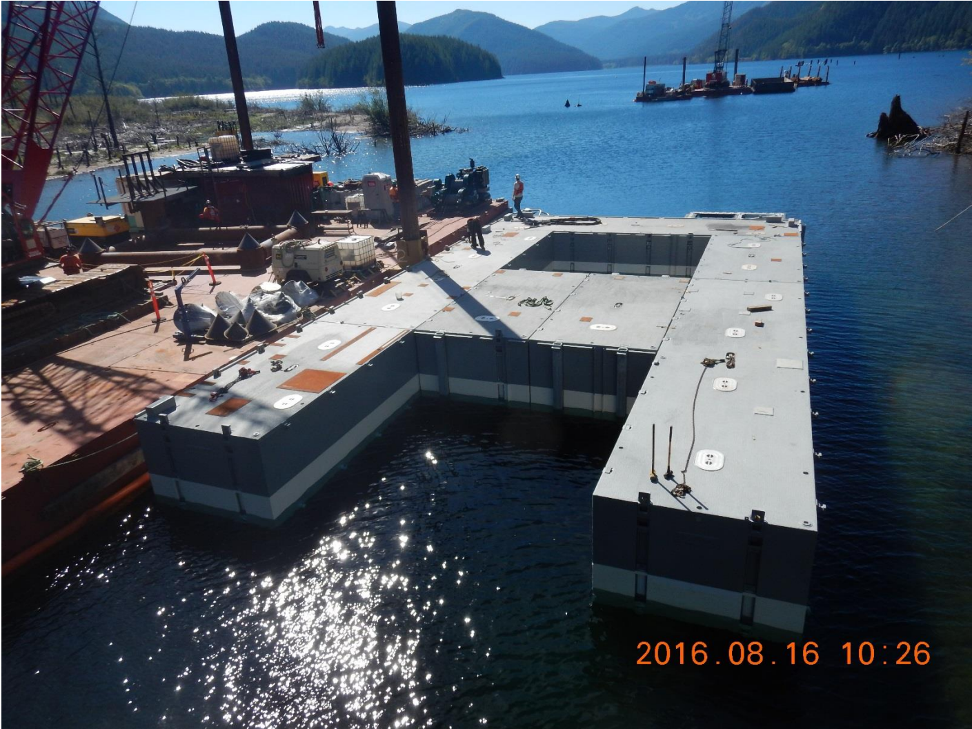
Morse Lake Pump Plant
