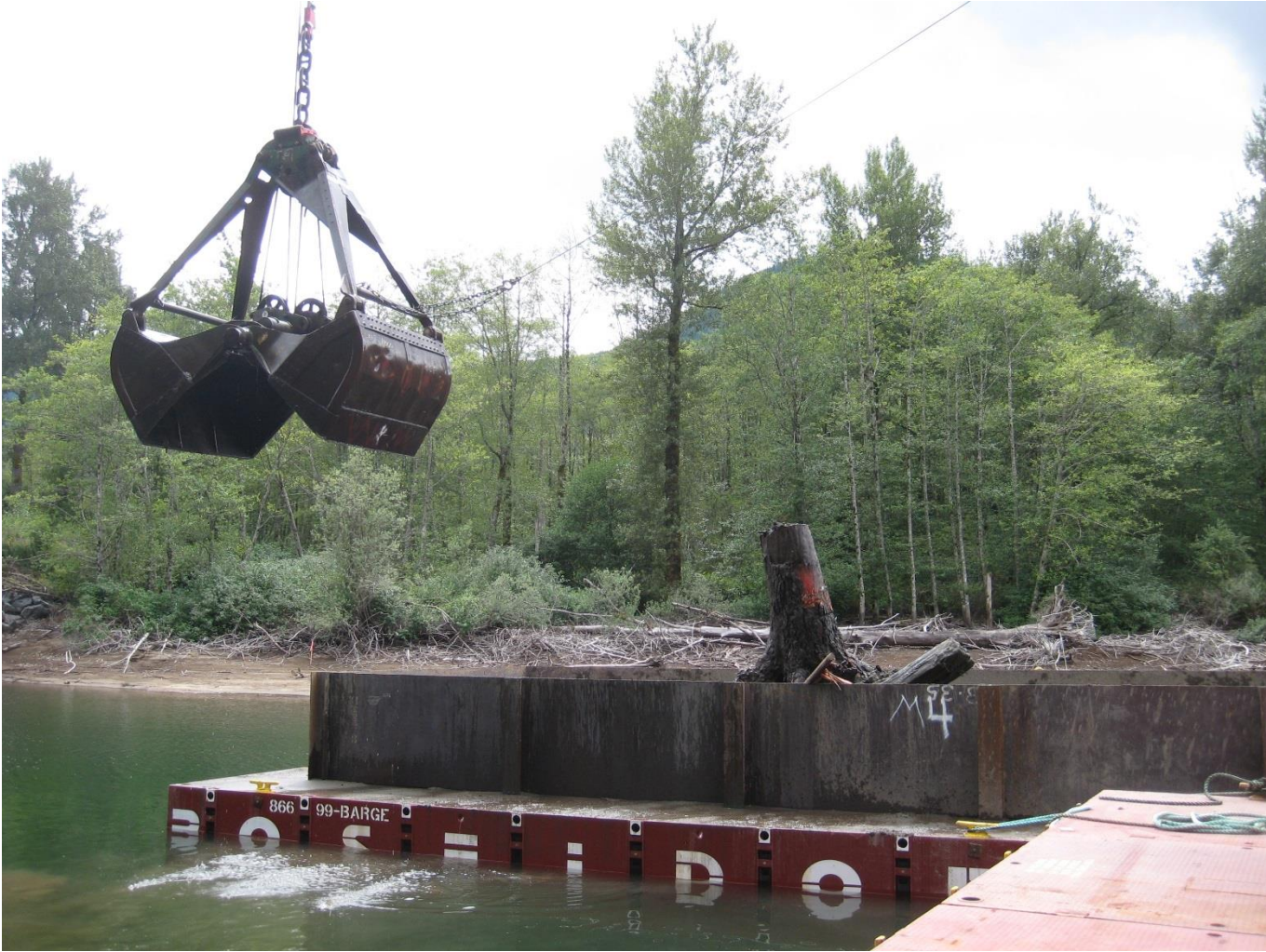
Morse Lake Pump Plant
