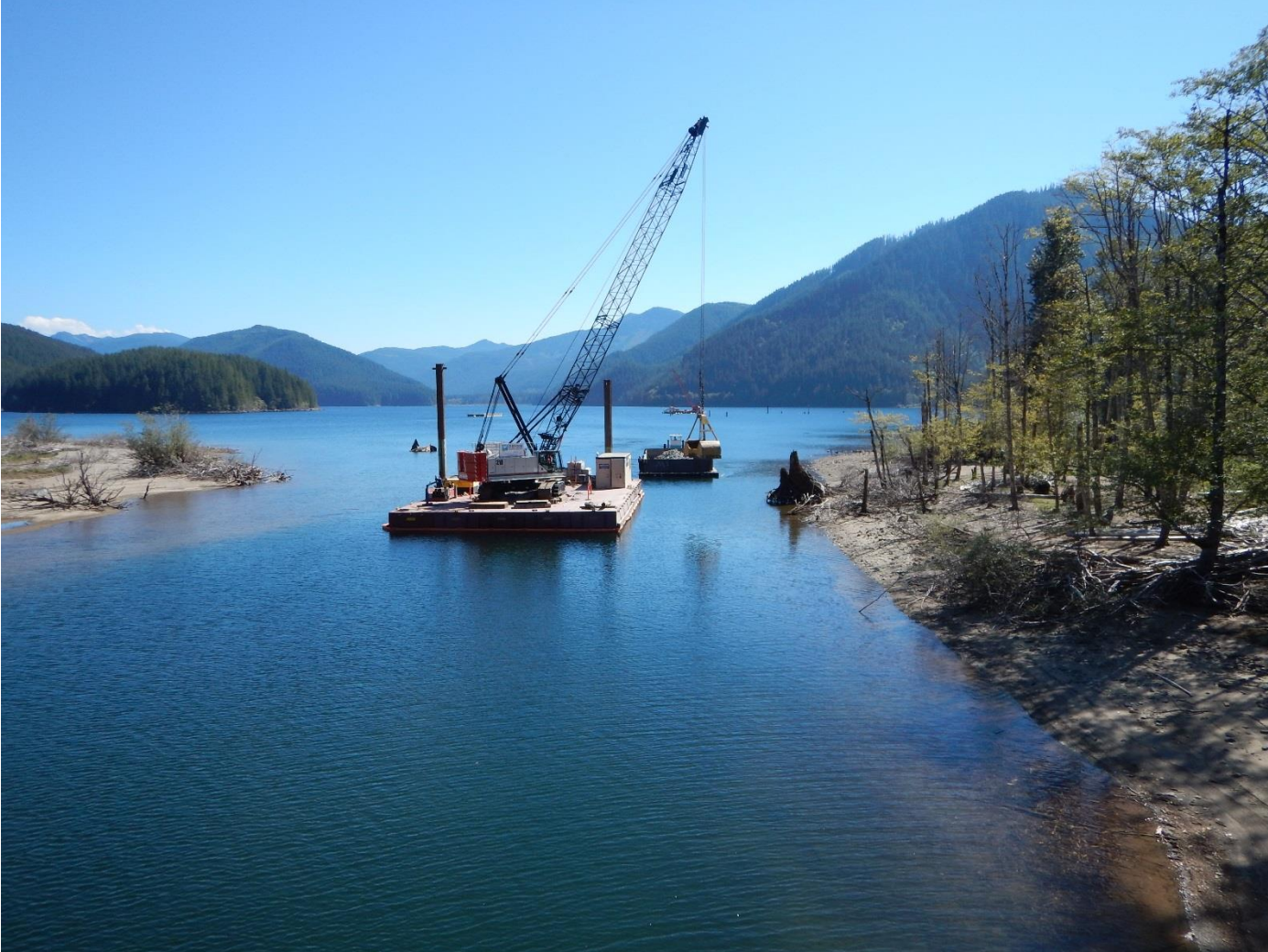
Morse Lake Pump Plant
