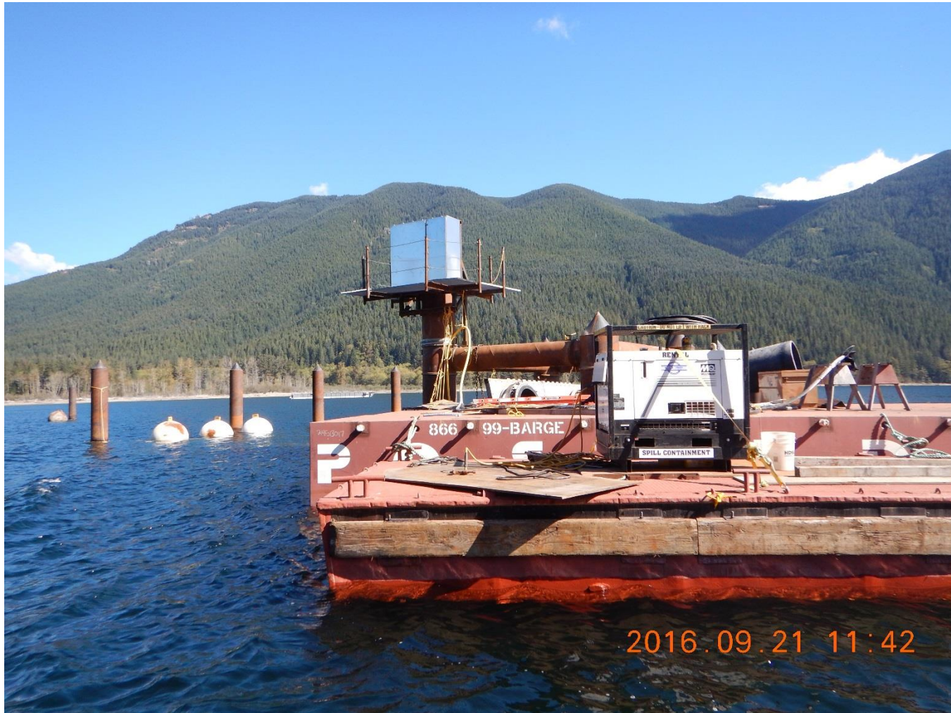
Morse Lake Pump Plant
