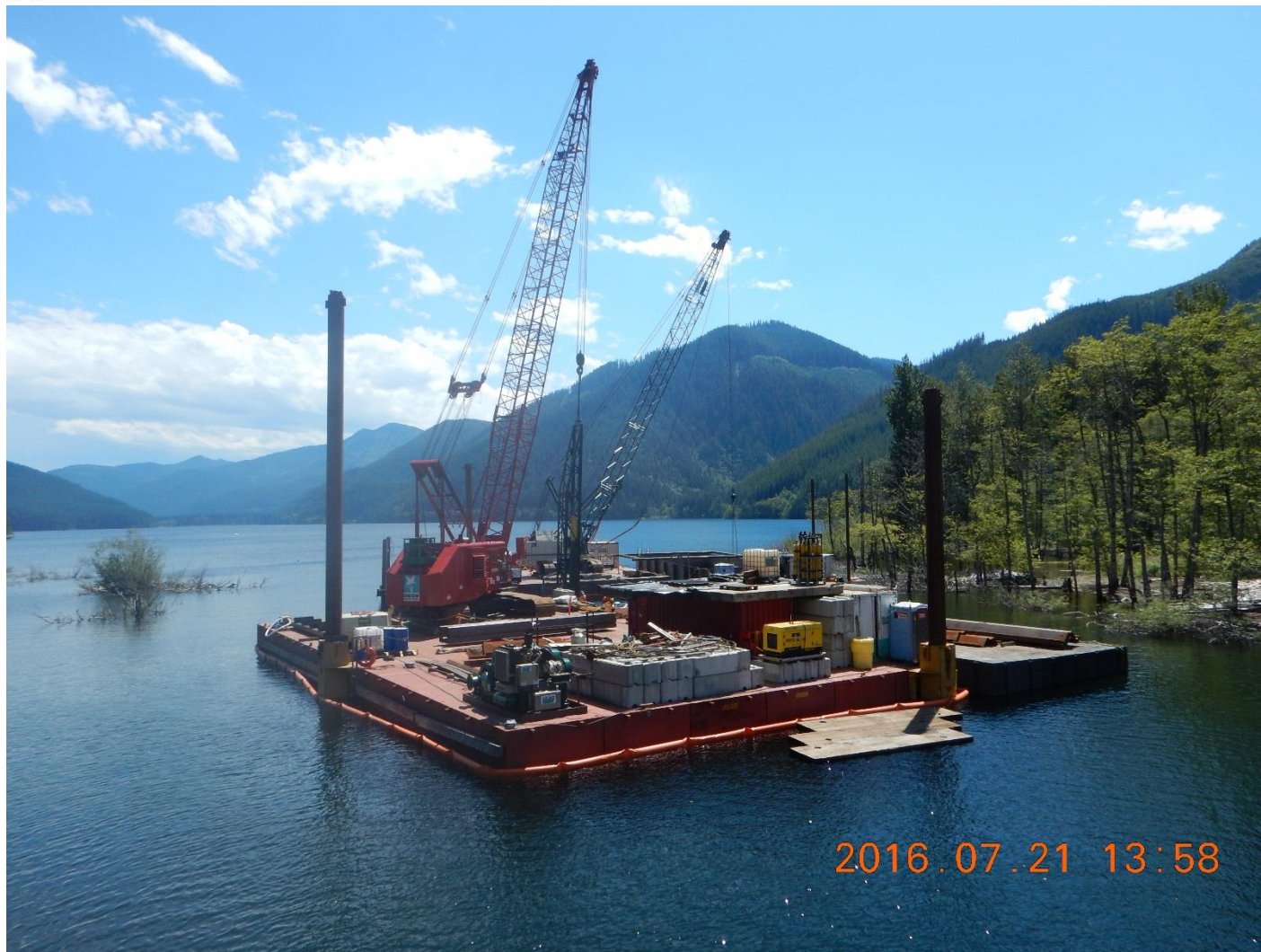
Morse Lake Pump Plant
