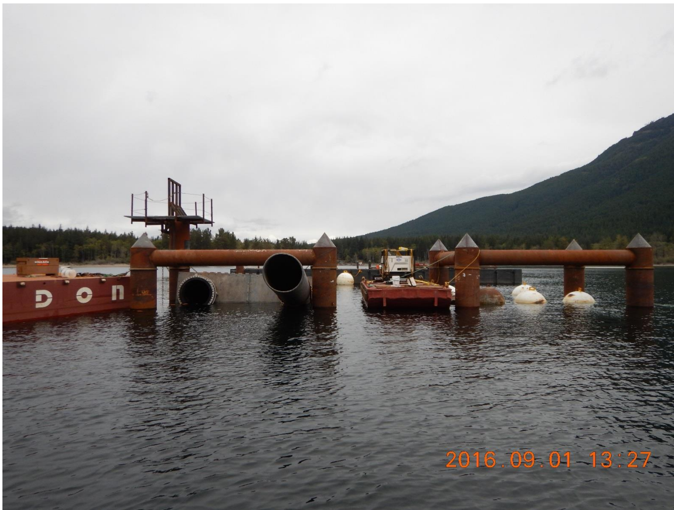
Morse Lake Pump Plant
