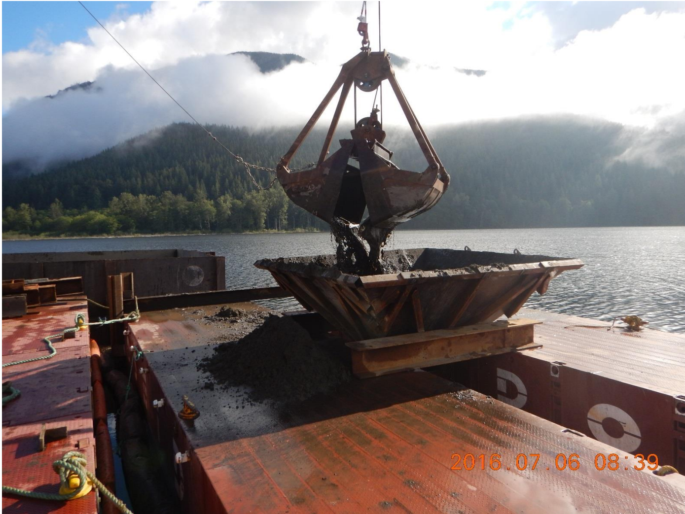
Morse Lake Pump Plant
