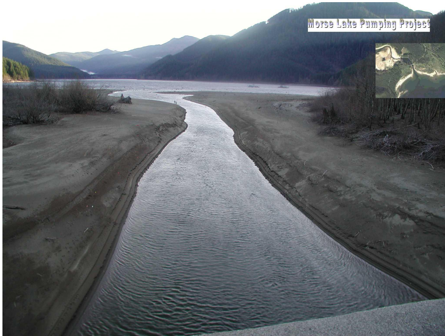
Morse Lake Pump Plant
