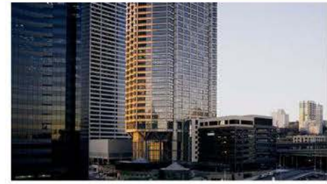
Municipal Tower, Seattle, WA
