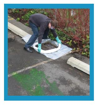
Protect the storm drain. If material has entered a storm drain, notify agencies listed on the back of this poster.
