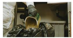
5 Scrape the sides, the lid, and the baffles with a putty knife to remove as much of the grease as possible. Put it into a watertight container.
