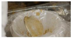
3 Remove all the accumulated grease out of the interceptor and put it in a watertight container.
