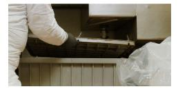
1 Remove the lid of the grease interceptor and bail out any water.
