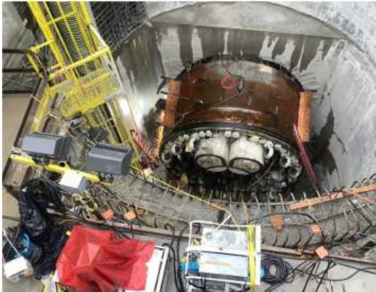
Figure 4-6. 8 ft. MudHoney completes mining of the 18 ft-10 in diameter Storage Tunnel
