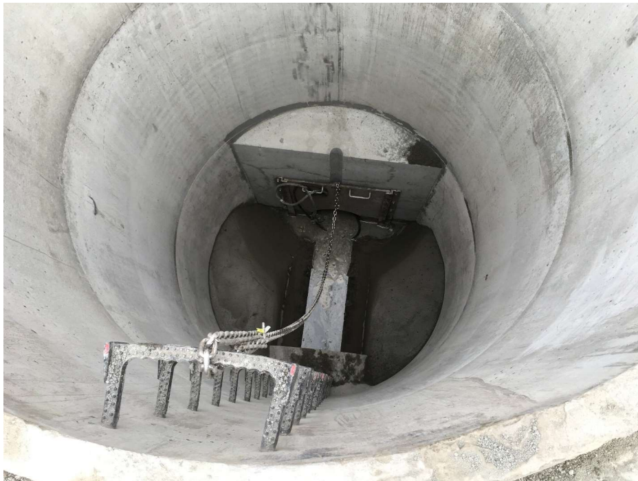
Figure 4-7. Central Waterfront Construction – Pike St Control Structure Orifice Plate
