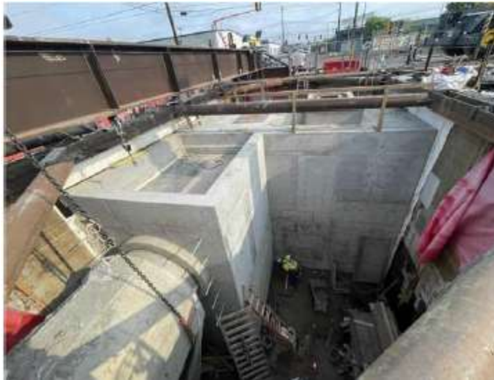
Figure 4-5. Construction of the 11 th Ave NW Flow Diversion Structure
