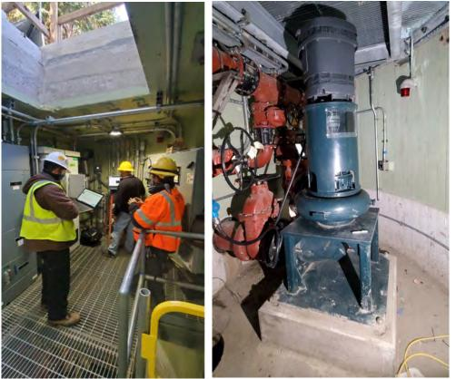
Figure 4-3. Operational Testing of Upgraded Pump Station 13 (left) and new pumps and valving (right)
