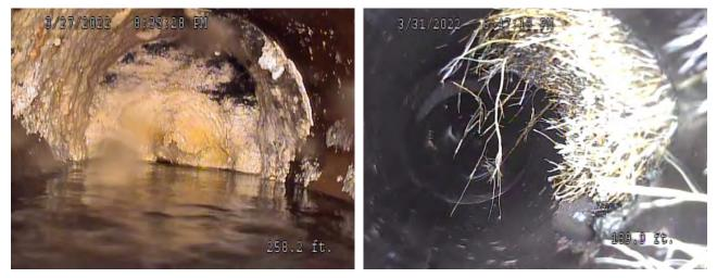
Figure 3-2. 2022 Private side sewer connections demonstrating visible FOG accumulations and impacts from root intrusion
