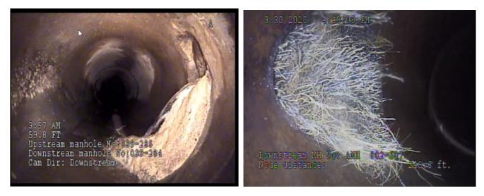
Figure 3-5. Private side sewer connections demonstrating visible FOG accumulations and impacts from root intrusion
