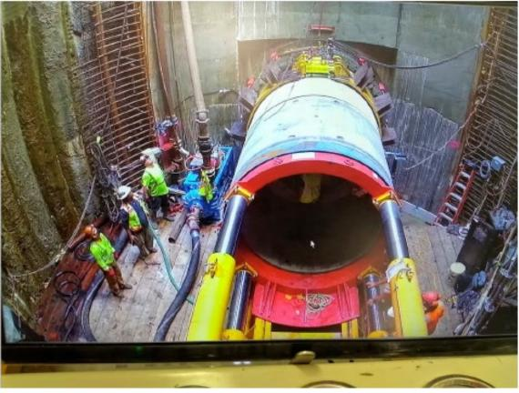
Figure 4-6. 8 ft. Diameter Microtunnel Installation
