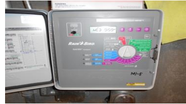
The irrigation system is controlled by a stand-alone Rainbird ESP-MC 12 controller.
