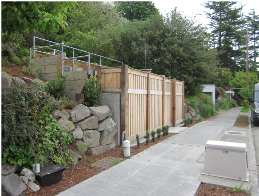
Figure 4-15. Pump Station 39 Backup Generator
