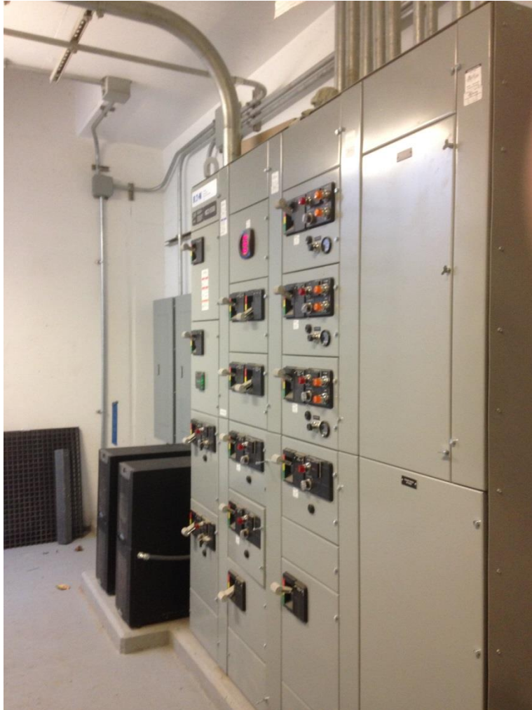
Figure 4-12. Genesee (CSO 9A) CSO Reduction Project Construction, September 2014
