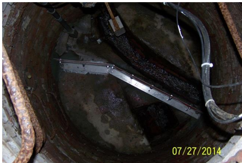
Figure 4-5. Outfall 29 Raised Weir Installation
