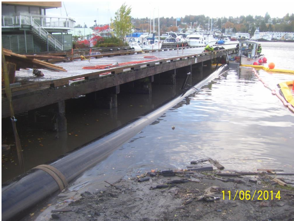
Figure 4-16. Outfall 150 Rehabilitation Project
