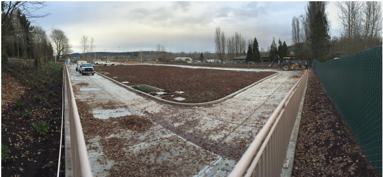
Figure 4-10. Windermere CSO Reduction Project Construction, February 2015
