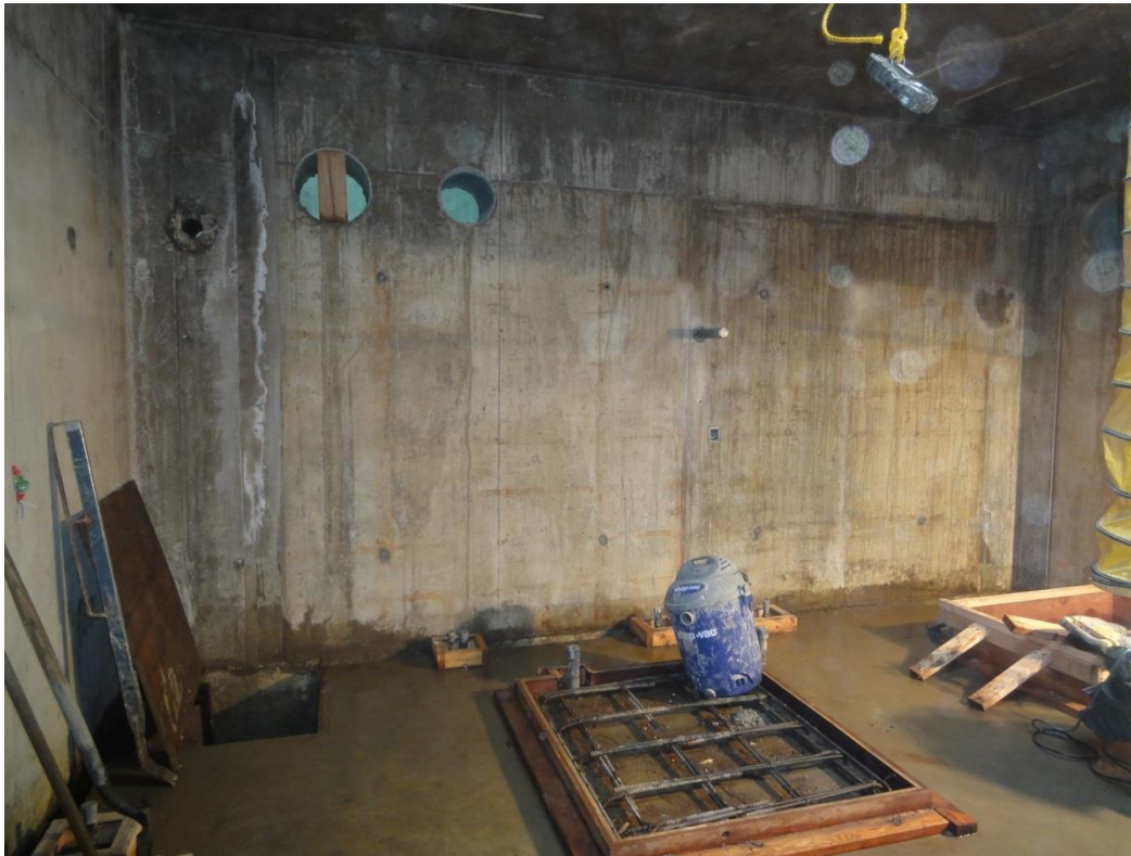
Figure 4-11. Genesee (CSO 11A) CSO Reduction Project Construction, July 2014
