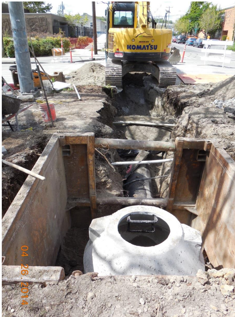
Figure 4-13. 52 nd Ave S Conveyance Project Construction, April 2014
