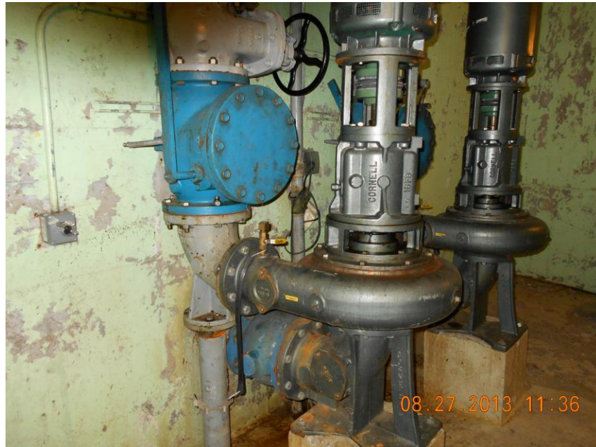
Figure 4-14. Pump Station 9 Rehabilitation Project
