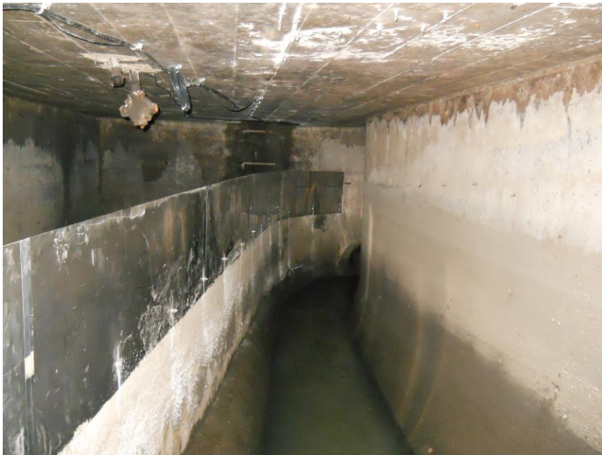
Figure 4-2. Retrofit Improvements At Overflow Structure 47C
