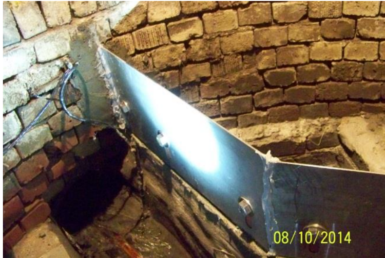
Figure 4-6. Outfall 30 Raised Weir Installation
