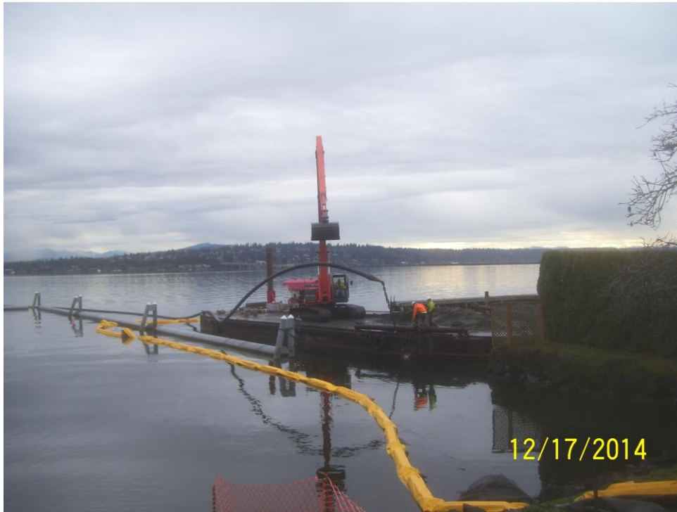
Figure 4-17. Outfall 31 Rehabilitation Project
