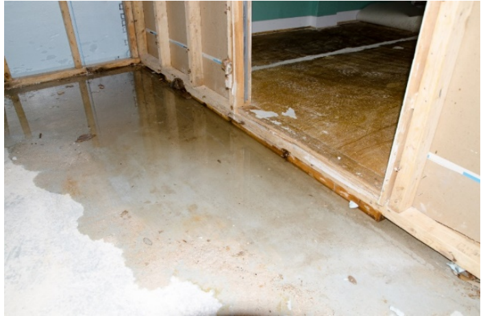
Flooding in a home's basement
