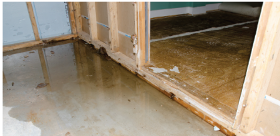
Storms can overwhelm pipes and lead to interior flooding and property damage.
