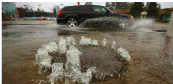
Heavy rain can lead to drain overflows that back up into sidewalks, streets, private property, and parking lots.
