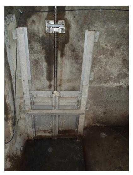
Figure 4-2. New Slide Gate in Basin 13 (Windermere Area)
