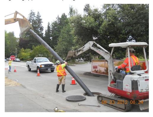
Figure 4-3. New Side Sewer Interceptor Pipe (North Union Bay Area)
