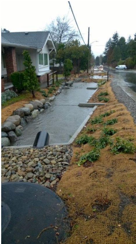
Figure II.6-4 Street View of Venema Natural Drainage System Project
