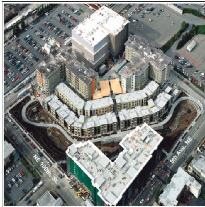
Figure III.6-3. TCWQC Project Site (Construction Phase)
