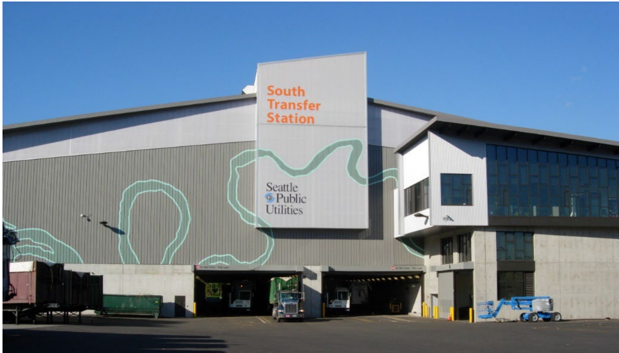
The South Transfer Station (Source: SPU Image Library)
