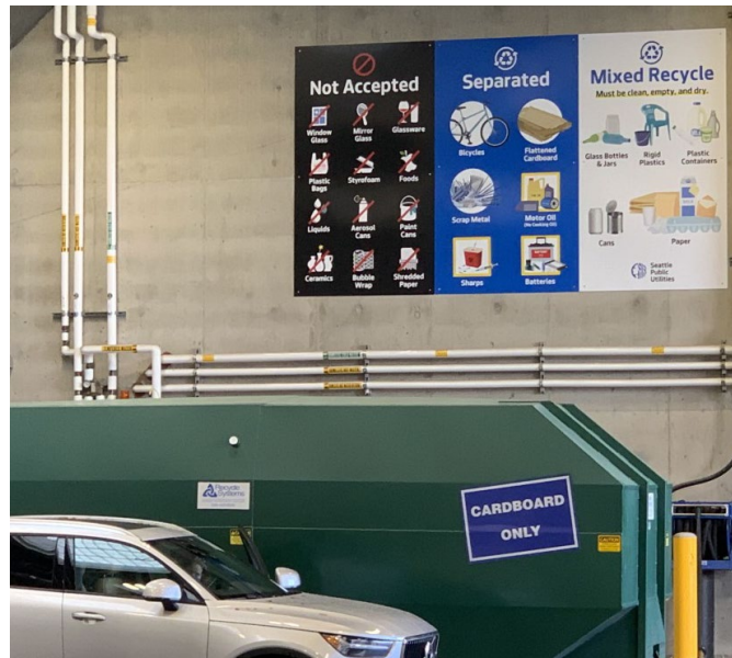
Compactor and signage at the North Transfer Station (Source: SPU Image Library)
