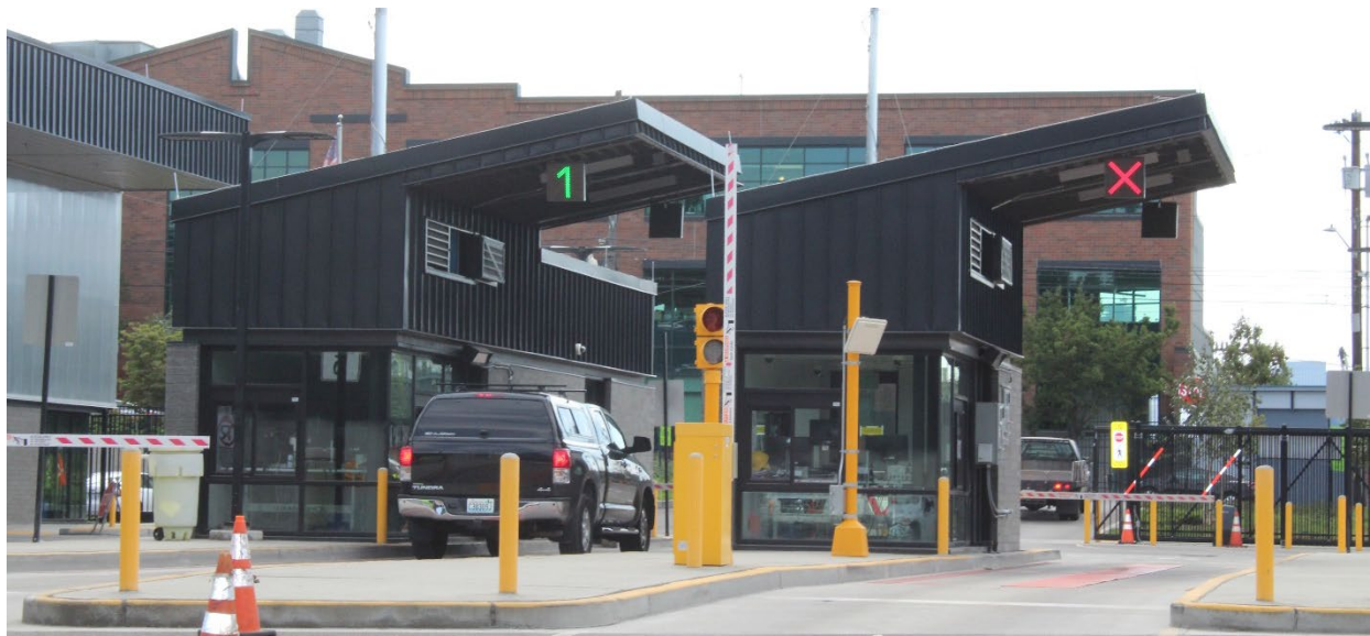
Customers drive across a scale at the North Transfer Station (Source: SPU Image Library)
