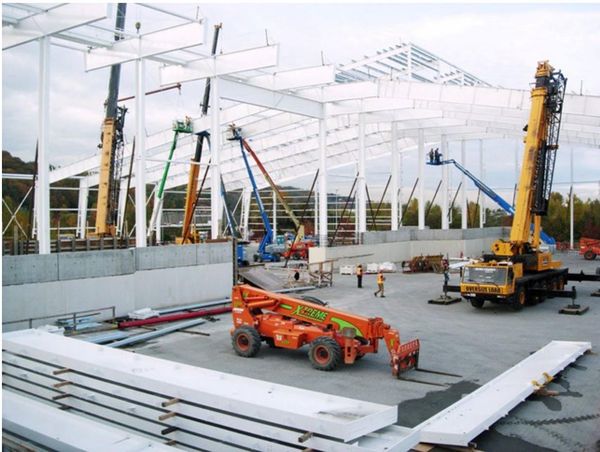
SPU’s South Transfer Station during construction (Source: SPU Image Library)
